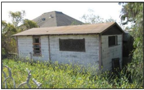
Figure 18: Guest house/bunkhouse situated to the immediate northeast of the main house. View looking southeast. One of the original Victorian-era windows is on the left hand side of the north elevation, while one of the new, unfinished openings is visible in the upper façade of the west elevation.
