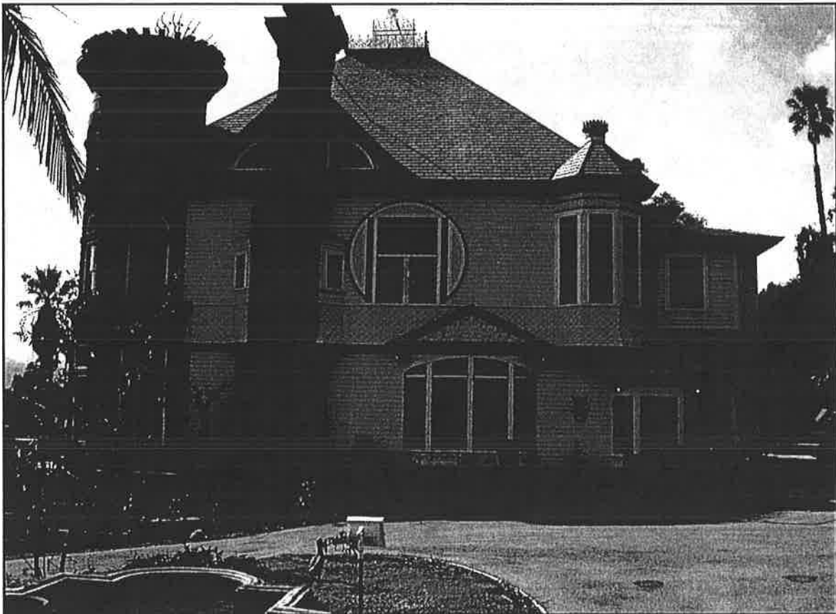
Photo 12. Side (eastern) elevation, Judy Triem, photographer [January 31, 2007]
