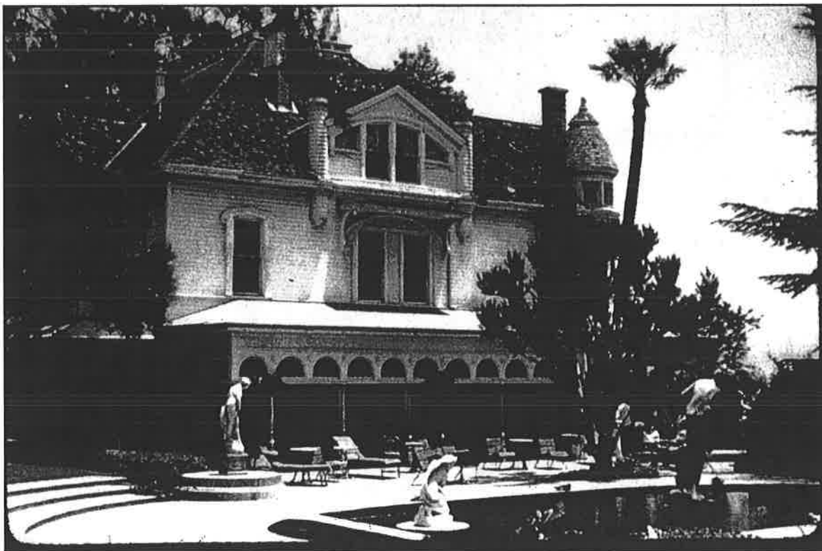
Photo 2. Side (Western) elevation, pre-fire, Phil Hardison, photographer [1980]
