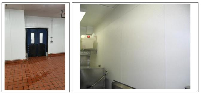
Typical FRP installation behind wall surface of sinks and prone splashing areas.
