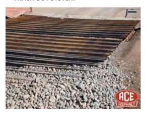
This BMP consists of stabilizing the defined entrance/exit point of the facility to reduce the sediment (mulch and dirt) onto public roads by vehicles. Stabilized entrances/exits are an effective method for reducing the tracking of sediment from the site.
