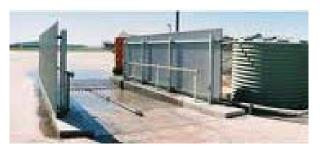
This BMP consist of washing equipment to maintain proper pathogen reduction and containing wash water to reduce cross-contamination potential.
