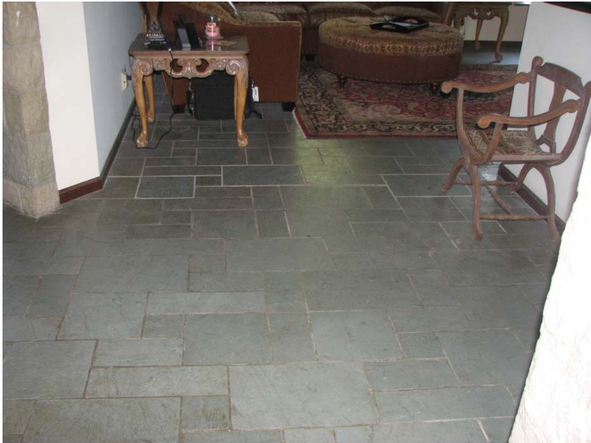
Warring Stone House, living room slate floor, 837 Park Street, Piru, June 6, 2012 (Charles J. Fisher photo)
