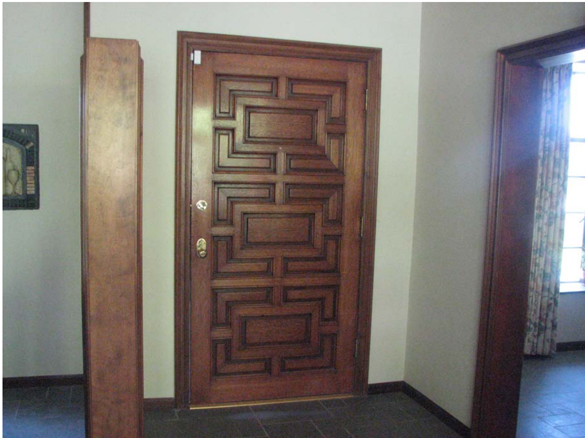
Warring Stone House, front entry, 837 Park Street, Piru, June 6, 2012 (Charles J. Fisher photo)
