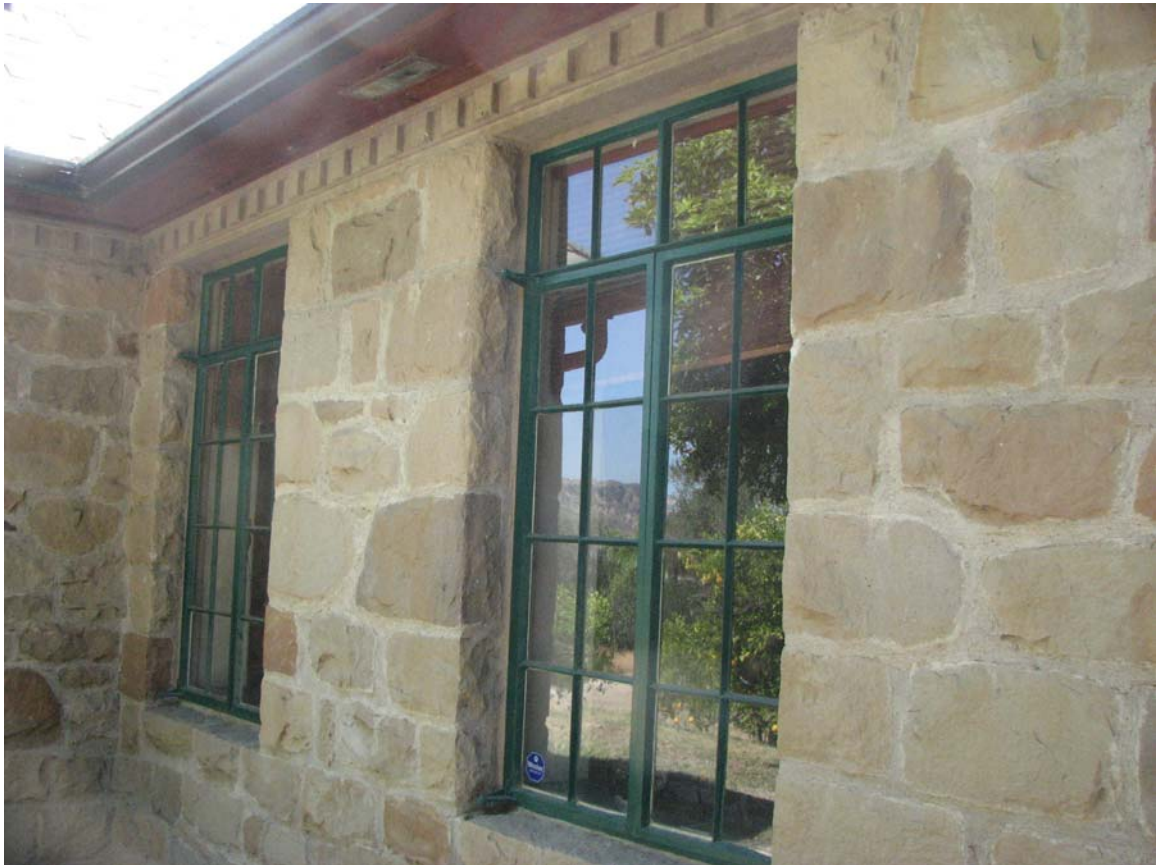
Warring Stone House, large casement windows, 837 Park Street, Piru, June 6, 2012 (Charles J. Fisher photo)
