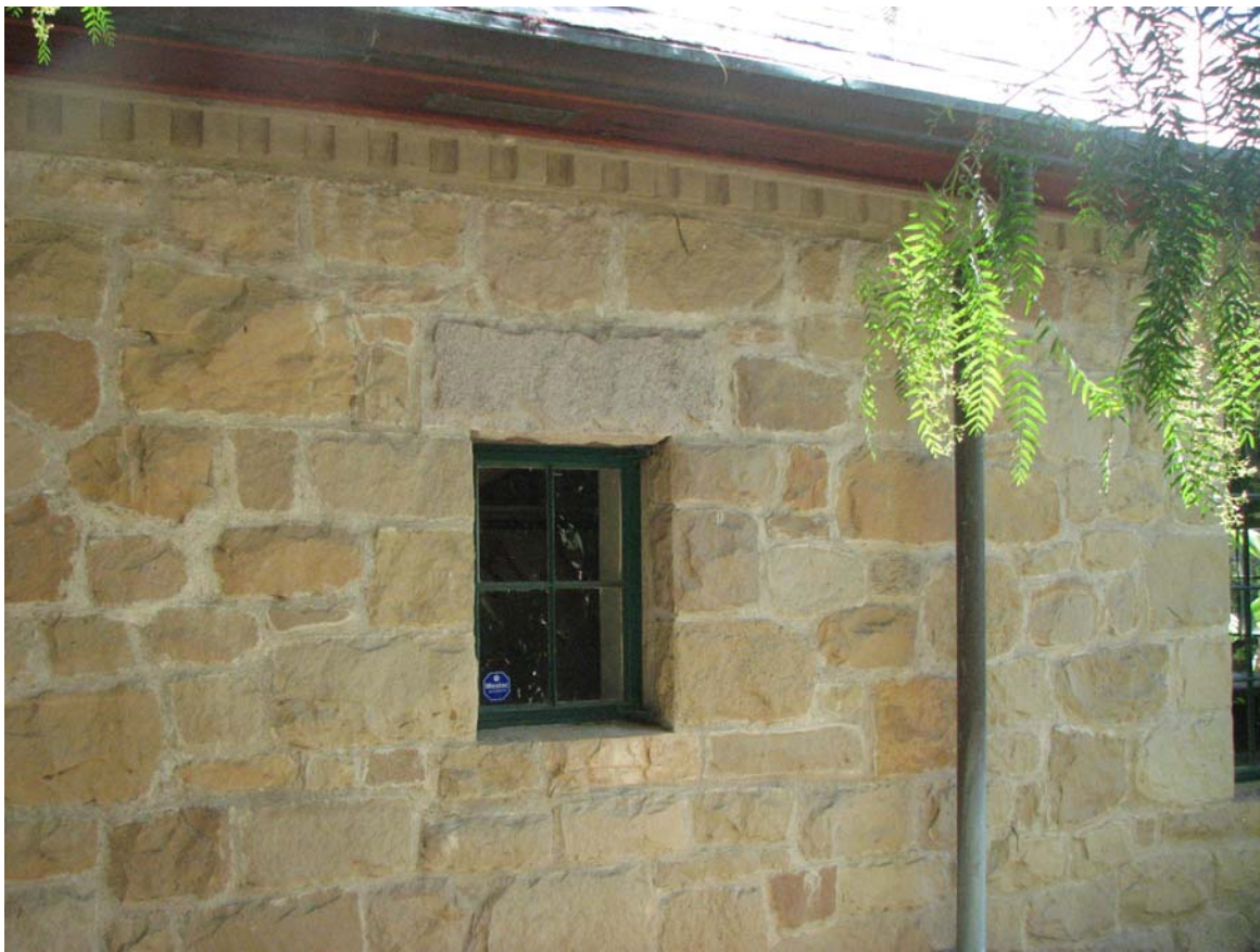
Warring Stone House, small window with lentil, 837 Park Street, Piru, June 6, 2012 (Charles J. Fisher photo)
