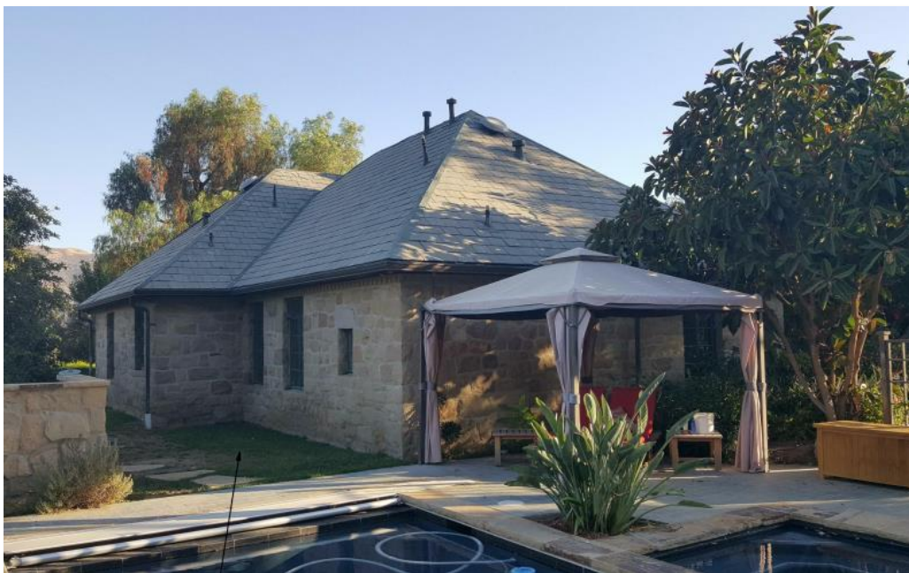
Figure 4 – Residence at 837 Park Street (east elevation)
