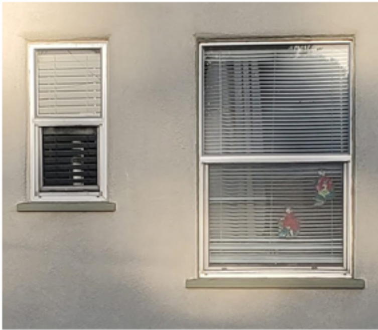
Existing Aluminum Single Hung Windows
