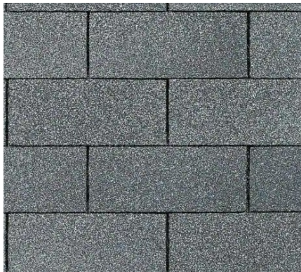
EXISTING ROOF SHINGLES TO REMAIN
