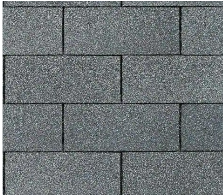
EXISTING ROOF SHINGLES TO REMAIN
