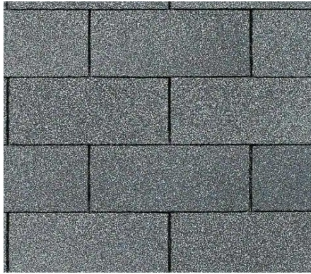
EXISTING ROOF SHINGLES TO REMAIN
