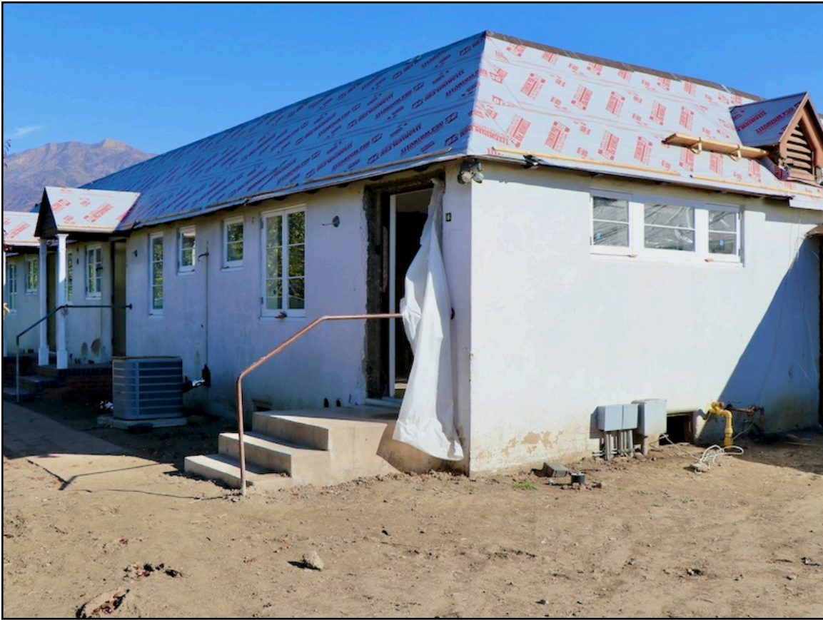
Photo 11. Recreation Room/Dorm (Building E/F), viewed from southwest. [12-8-2021]
