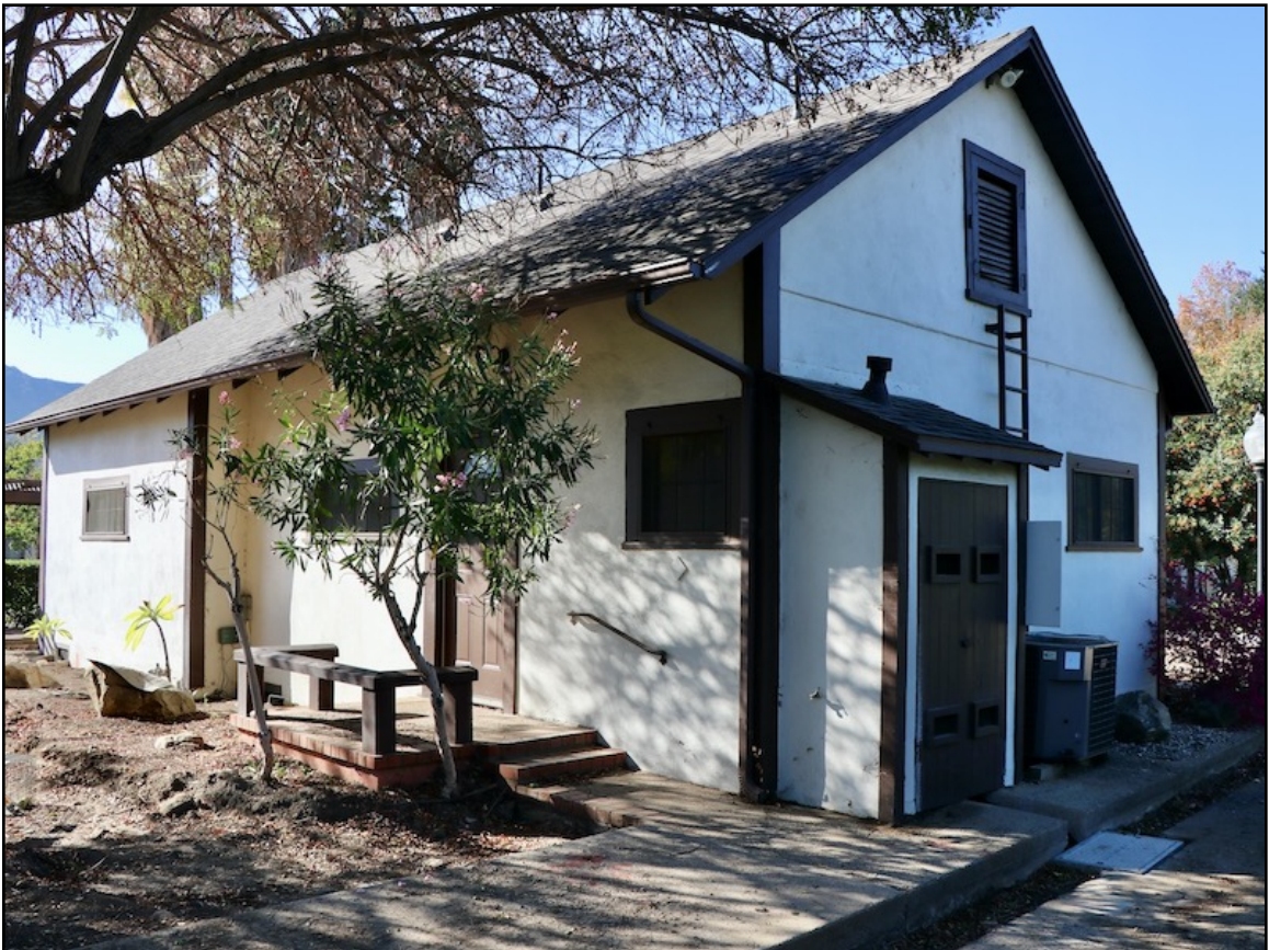
Photo 2. Residence [Building A], viewed from northeast. [12-8-2021]
