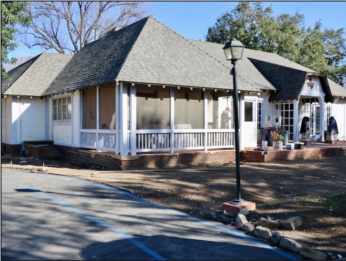
Photo 7. Main Residence (Building D), viewed from southwest. [12-8-2021]
