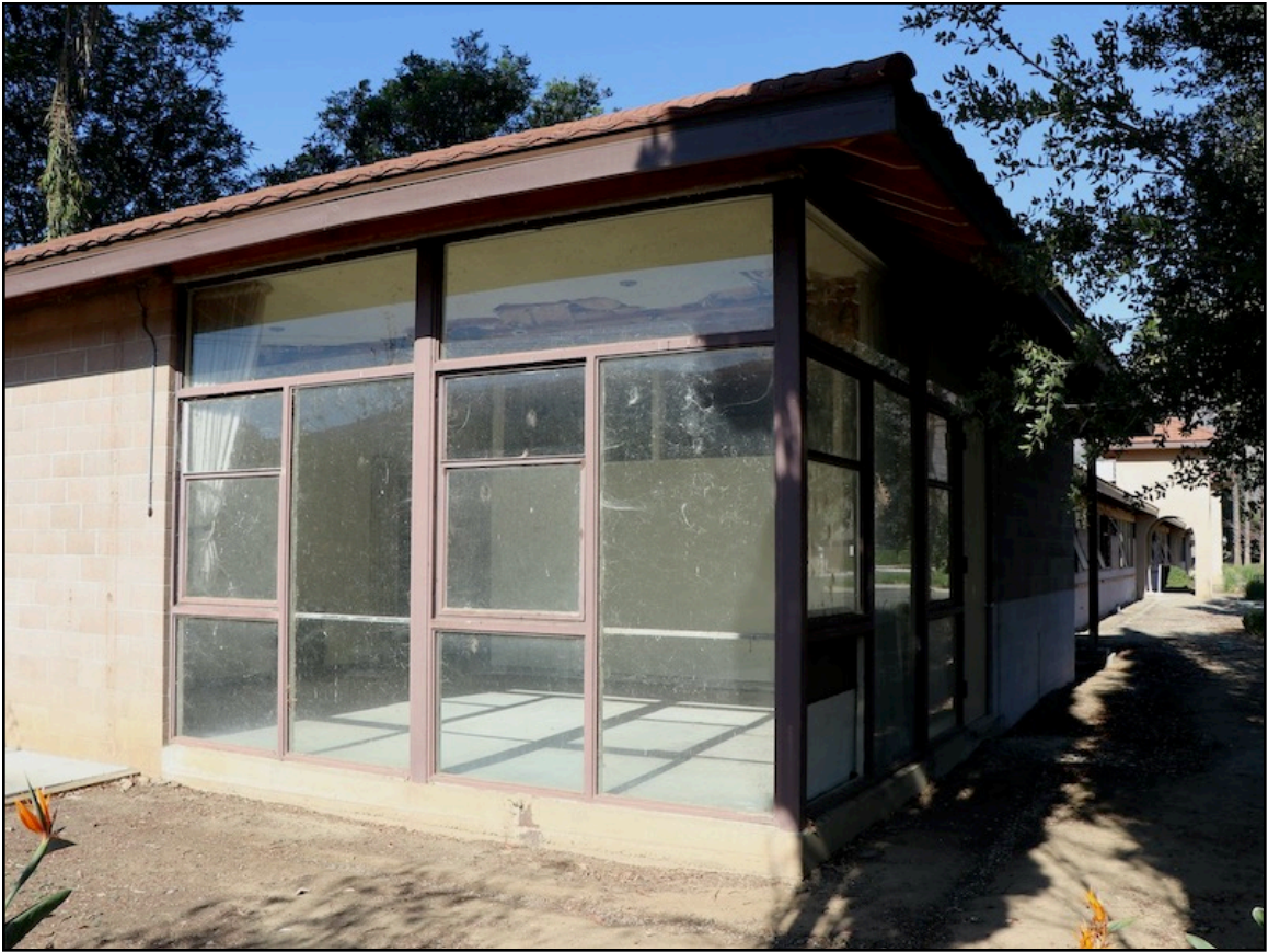
Photo 21. Novitiate (Building L), southeastern corner of east wing, viewed from southeast. [12-8-2021]
