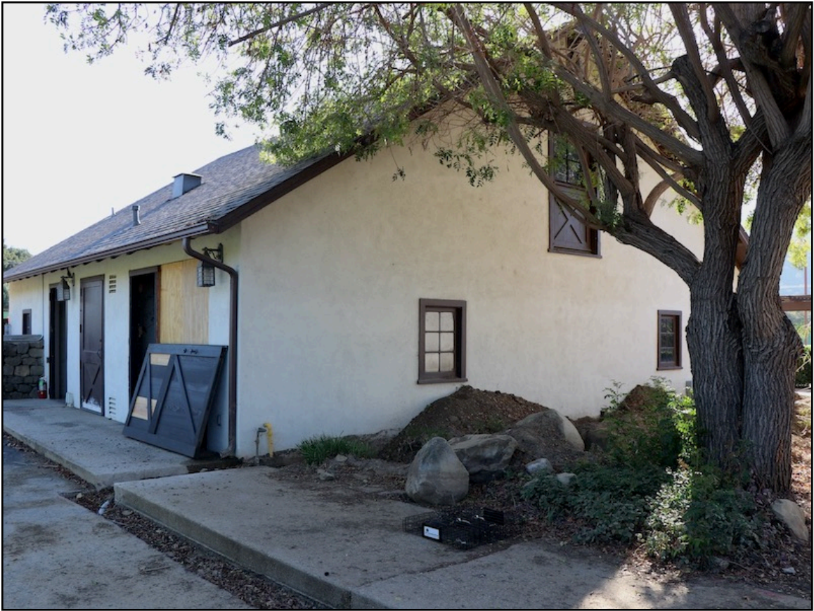
Photo 3. Barn/Stables (Building B), viewed from northwest. [12-8-2021]
