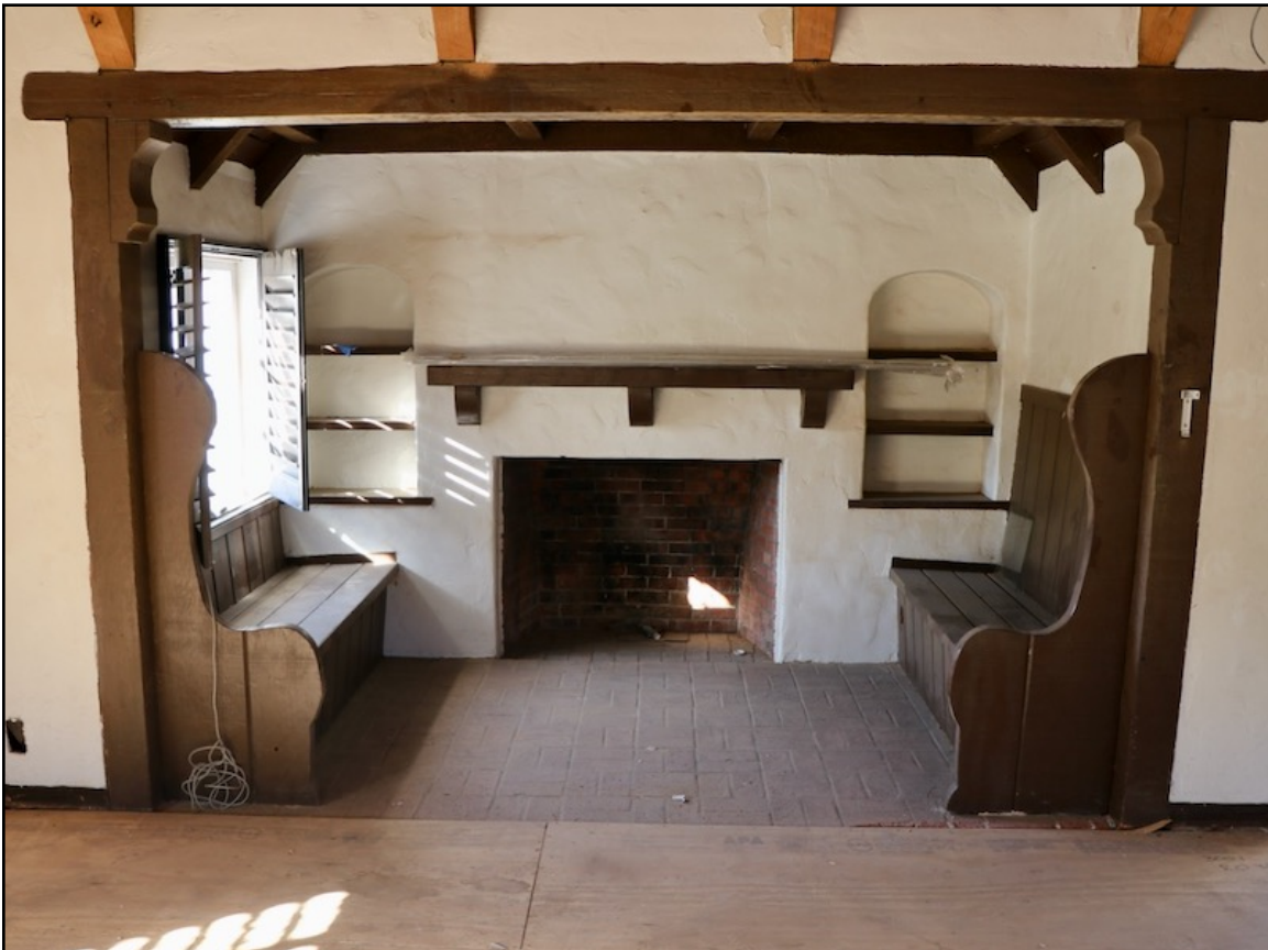
Photo 12. Recreation Room/Dorm (Building E/F, interior. [12-8-2021]
