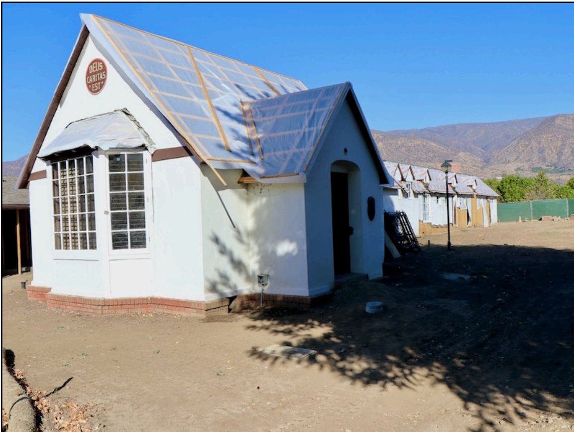
Photo 10. Recreation Room/Dorm (Building E/F), viewed from southeast. [12-8-2021]
