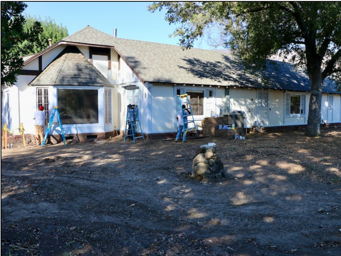
Photo 8. Main Residence (Building D), viewed from east. [12-8-2021]
