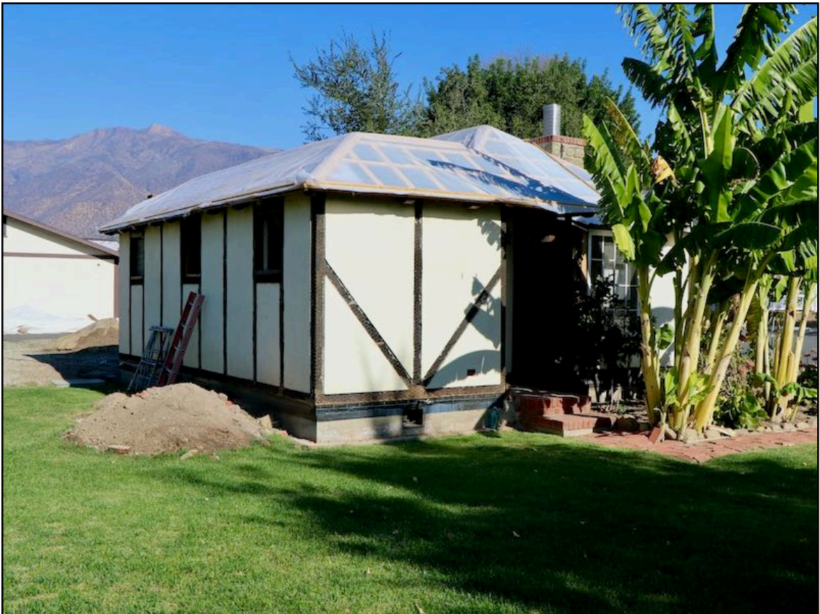
Photo 16. Doll House (Building J), viewed from southwest. [12-8-2021]
