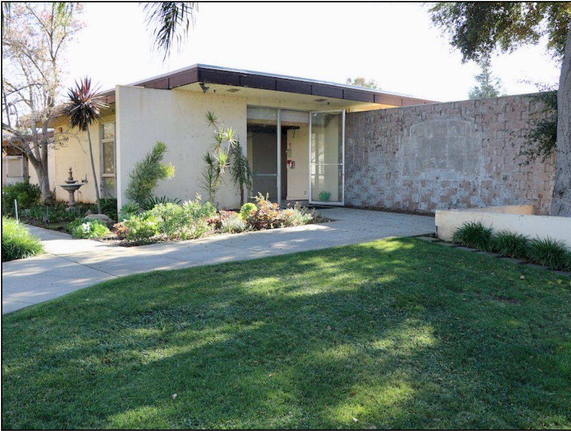
Photo 17. Hospital (Building K), main entry, viewed from northwest. [12-8-2021]
