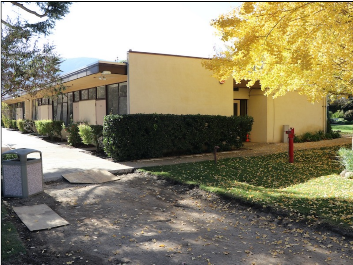
Photo 18. Hospital (Building K), patient room wing, viewed from northeast. [12-8-2021]
