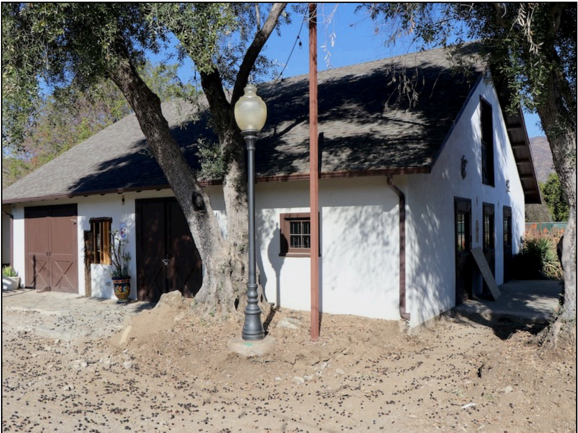
Photo 4. Barn/Stables (Building B), viewed from southeast. [12-8-2021]
