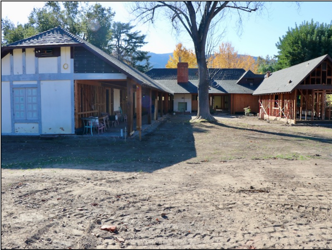
Photo 9. Main Residence (Building D), viewed from north. [12-8-2021]
