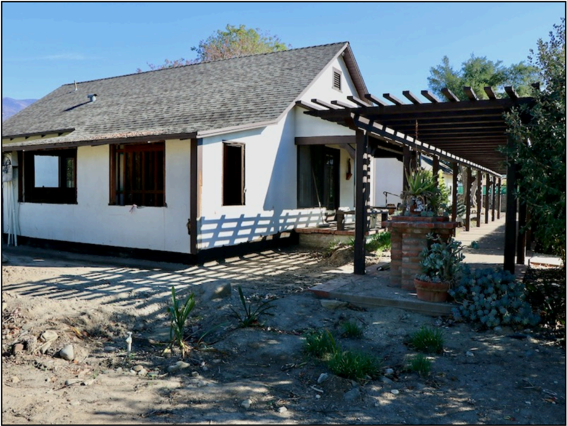
Photo 1. Residence (Building A), viewed from southwest. [12-8-2021]
