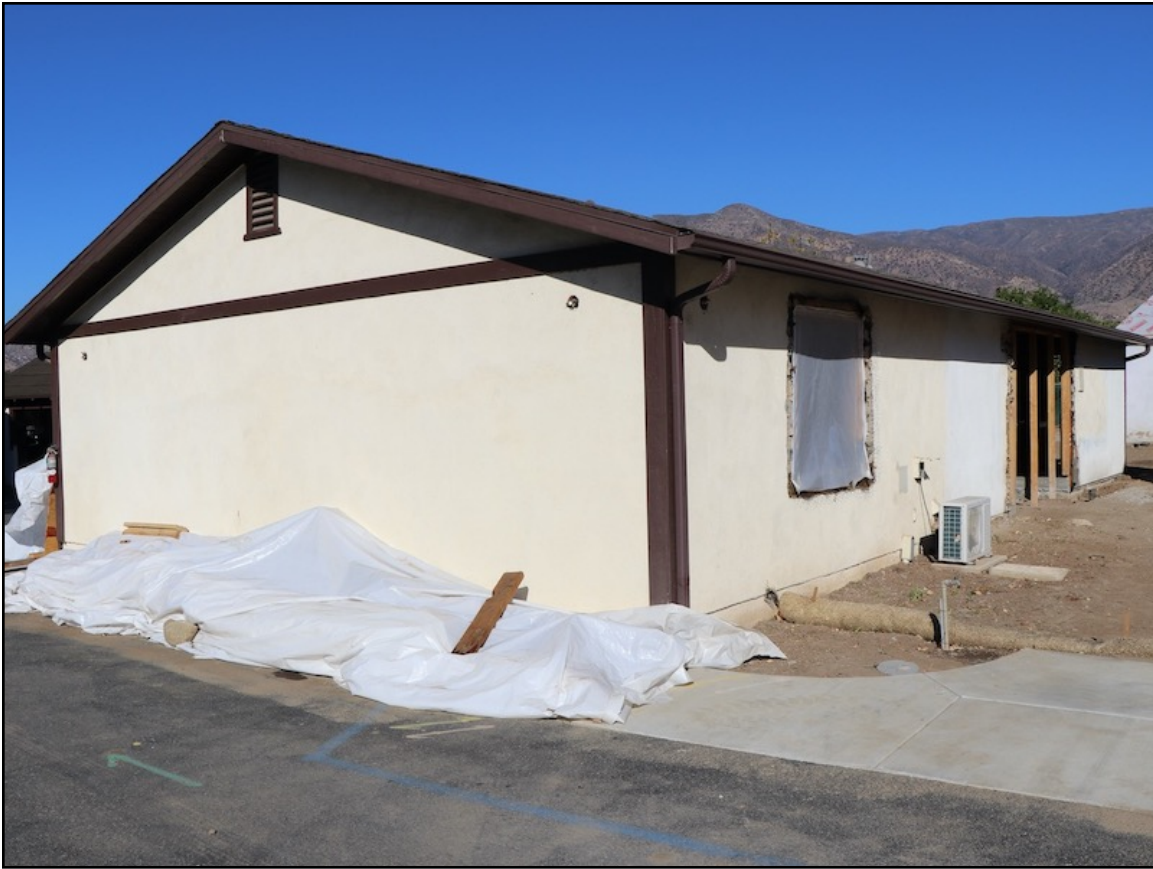
Photo 13. Garage/Shop (Building G), viewed from southeast. [12-8-2021]
