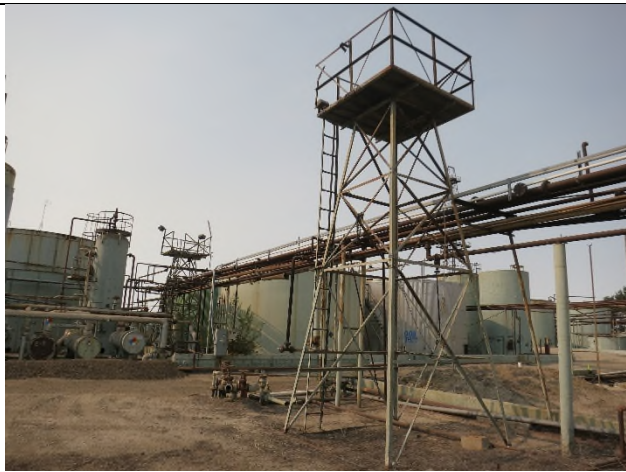
Image 3. Access platform and pipelines looking southwest.
