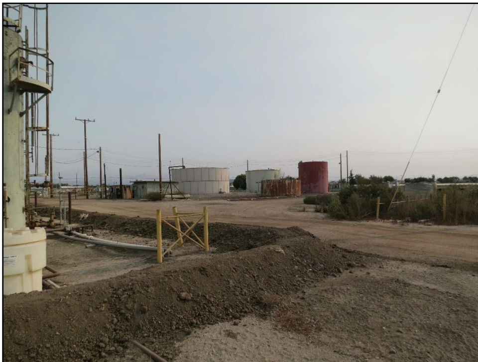
Figure 46. Overview of tanks on east side of driveway, looking northeast.
