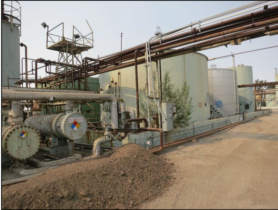
Figure 33. Tanks 2009 and 2008, looking west.
