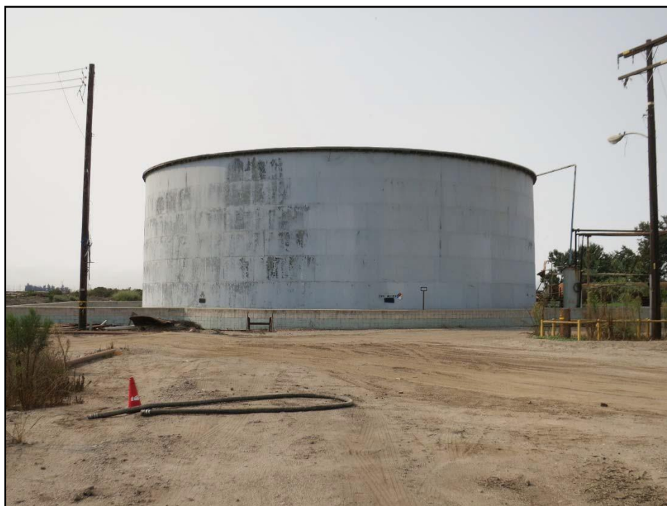
Figure 38. Tank 30001, looking south.
