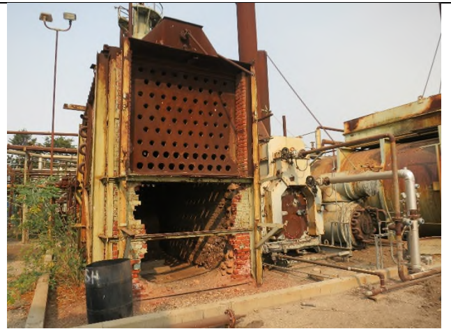
Image 4. Brick heater looking northwest
