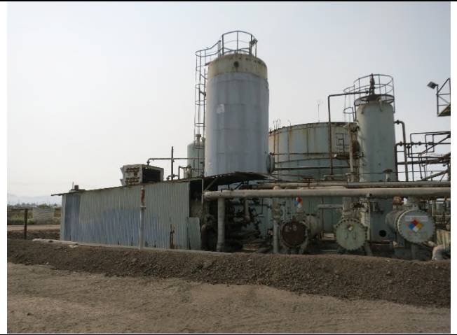
Image 2. Structures to the north of the Water Tank looking south.
