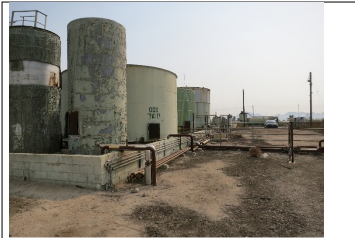
Image 3. Tanks 2011, 2012 and water tank looking east.
