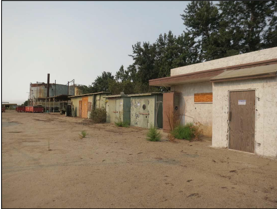
Figure 18. View of Lab, Fire Station and Maintenance Shop, looking southwest.
