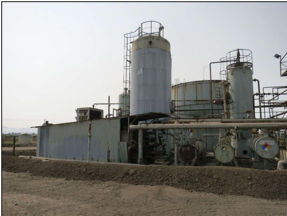
Figure 40. Structures to the north of the Water Tank, looking south.
