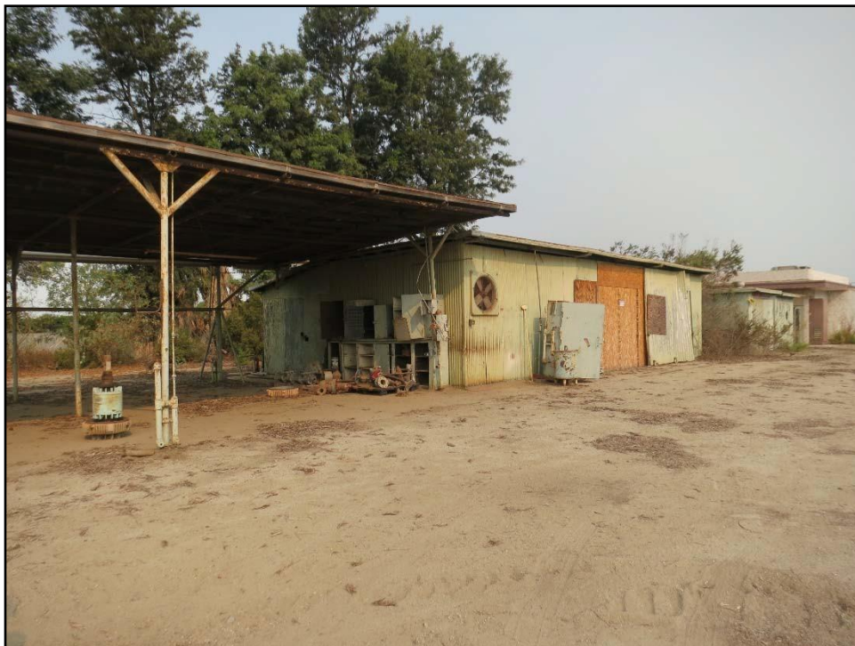
Figure 15. View of the Maintenance Shop, looking northwest.
