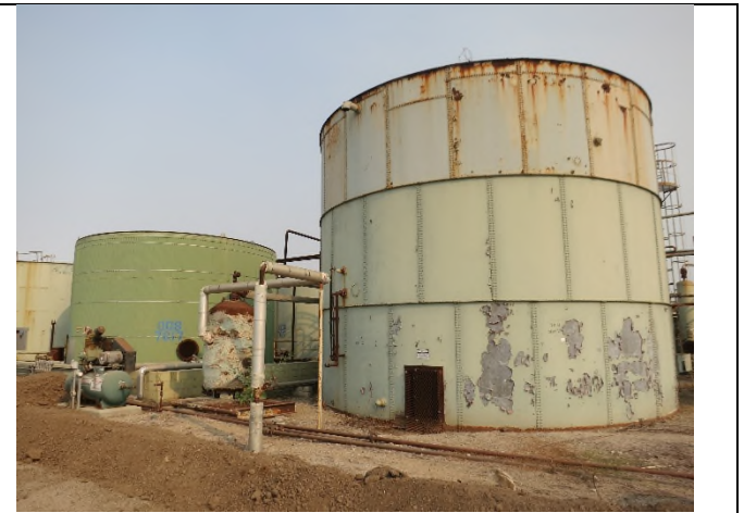
Image 4. View of Water Tank looking northwest
