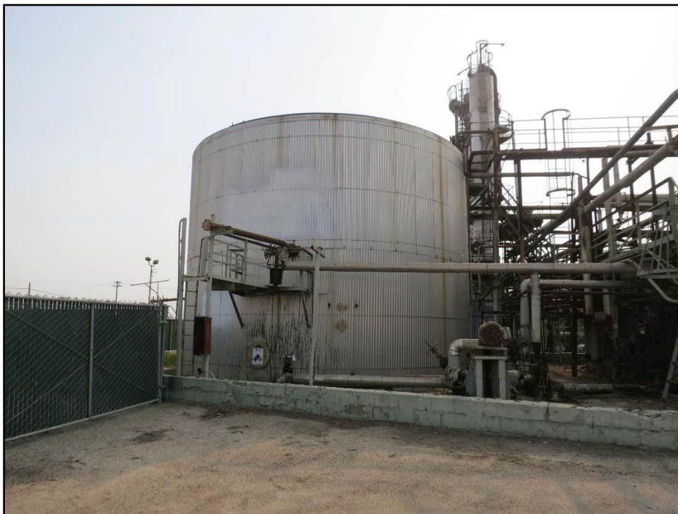
Figure 36. View of Tank 3501, looking east.
