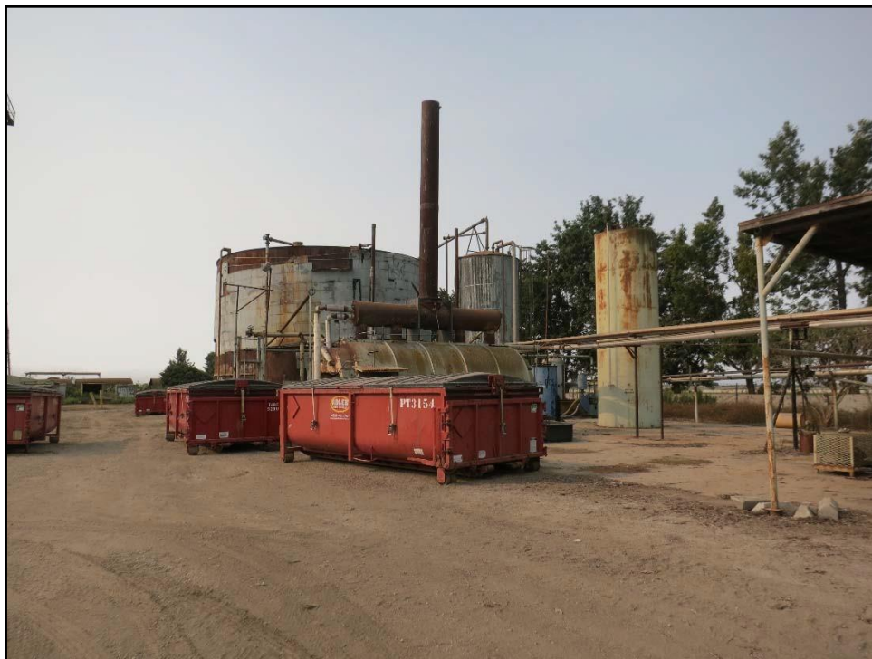
Figure 26. Tanks 506 and 506, looking south.
