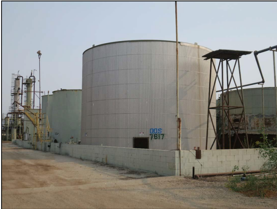
Figure 35. View of Tank 3502, looking northeast.
