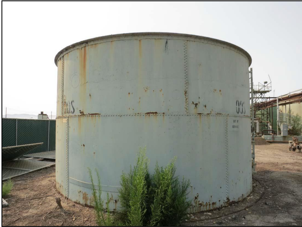
Figure 25. View of Tank 501, looking south.
