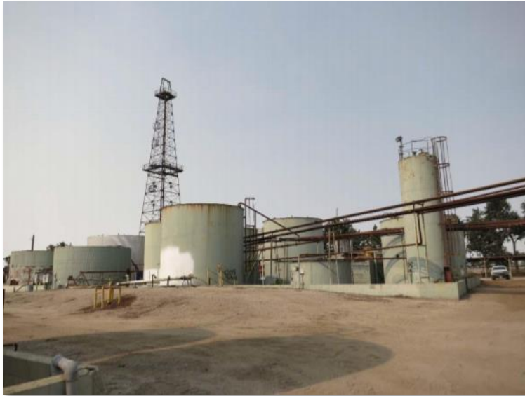
Figure 7 – View of 1500 Series Tanks
