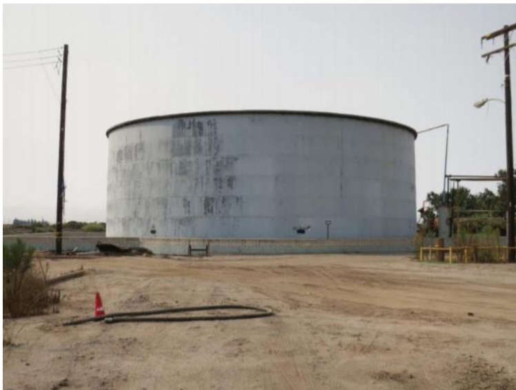
Figure 8 – View of Tank 30001
