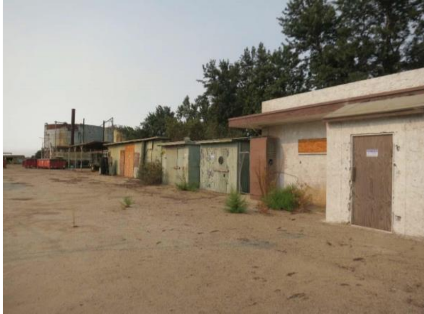
Figure 5 – View of Lab, Fire Station and Maintenance Shop
