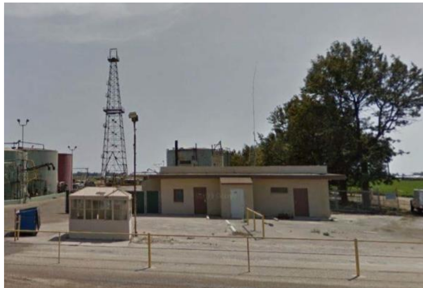
Figure 6 – View of North Façade of Lab
