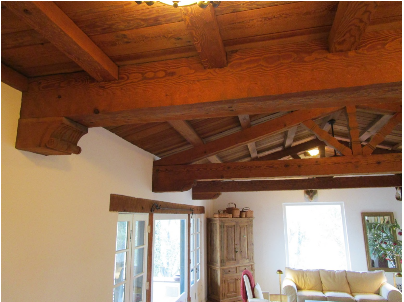
Photograph 22c, Living room, detail of open truss ceiling
