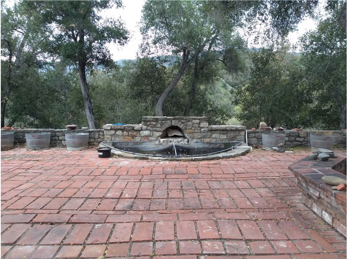
Photograph 34, Rear Terrace, ornamental water feature, existing conditions, looking south
