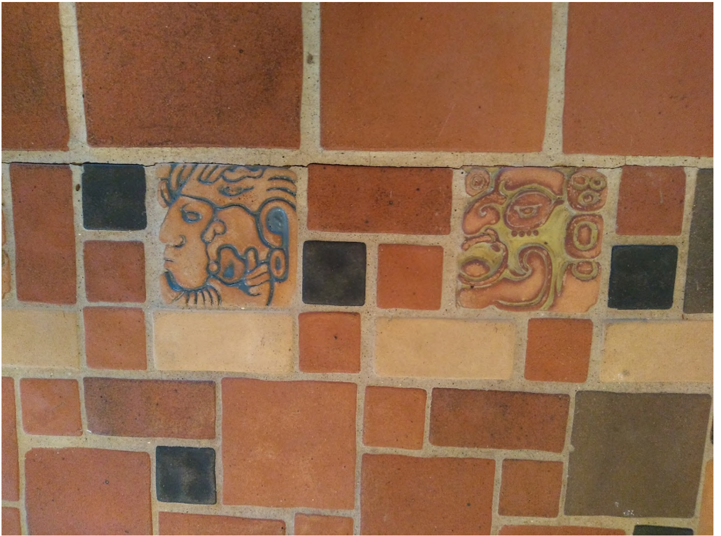
Photograph 21, Entry Hall, detail of Mayan inspired tilework by Ernest Allan Batchelder
