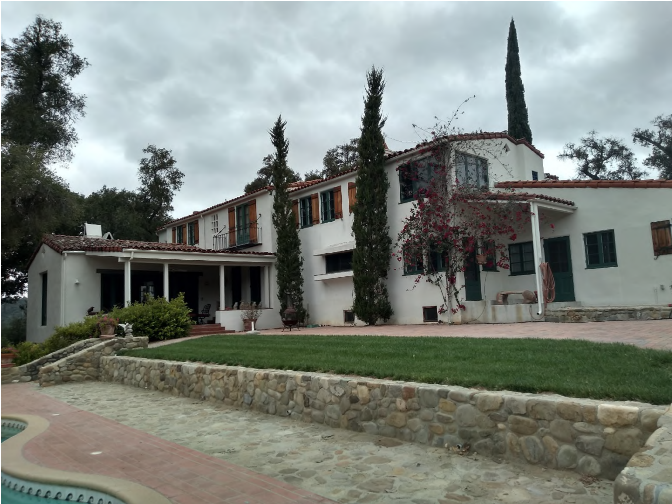
Photograph 6, South Elevation, rear of house, existing conditions, looking northwest
