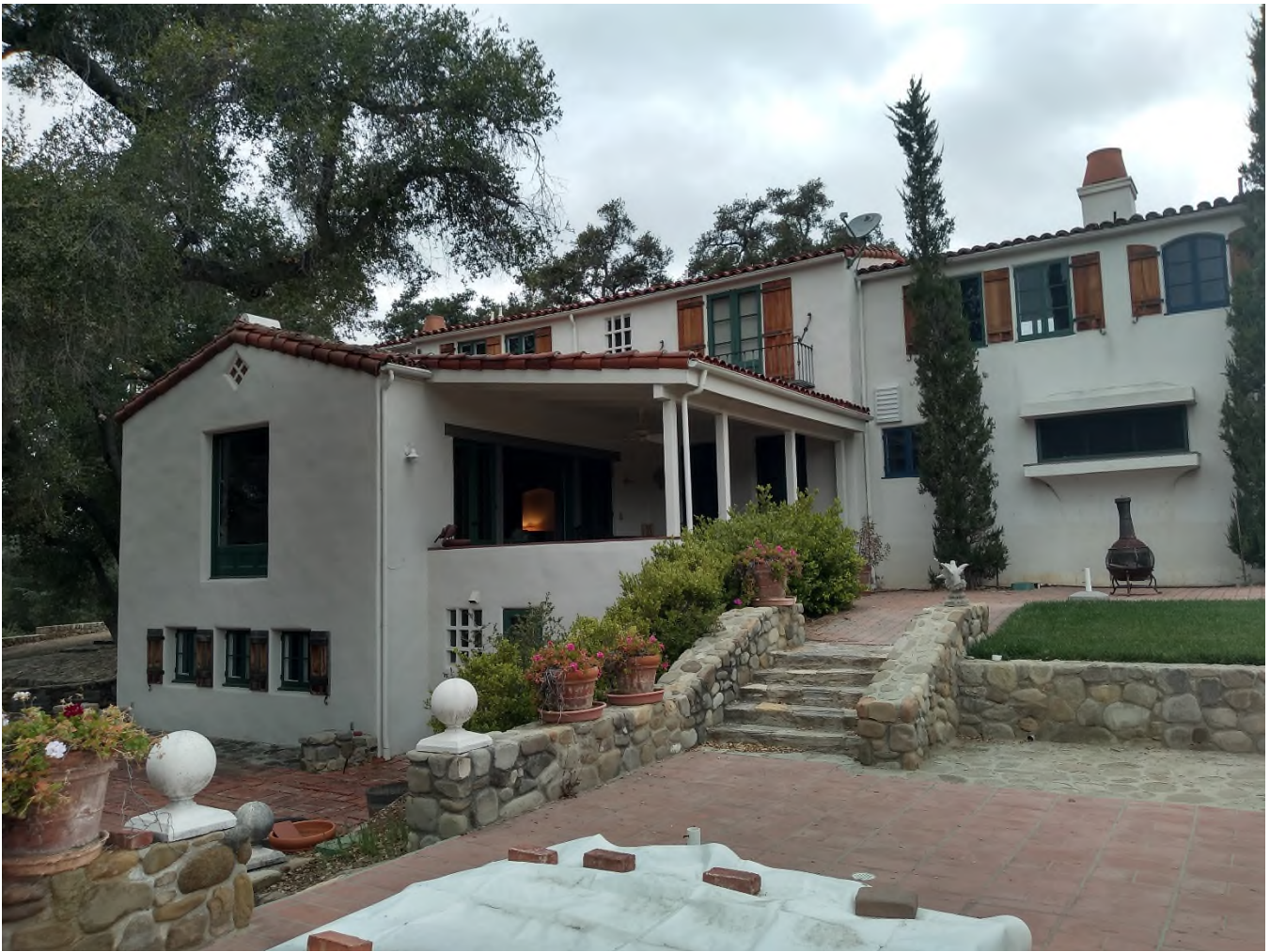
Photograph 10, South Elevation, rear of house, existing conditions, looking northwest
