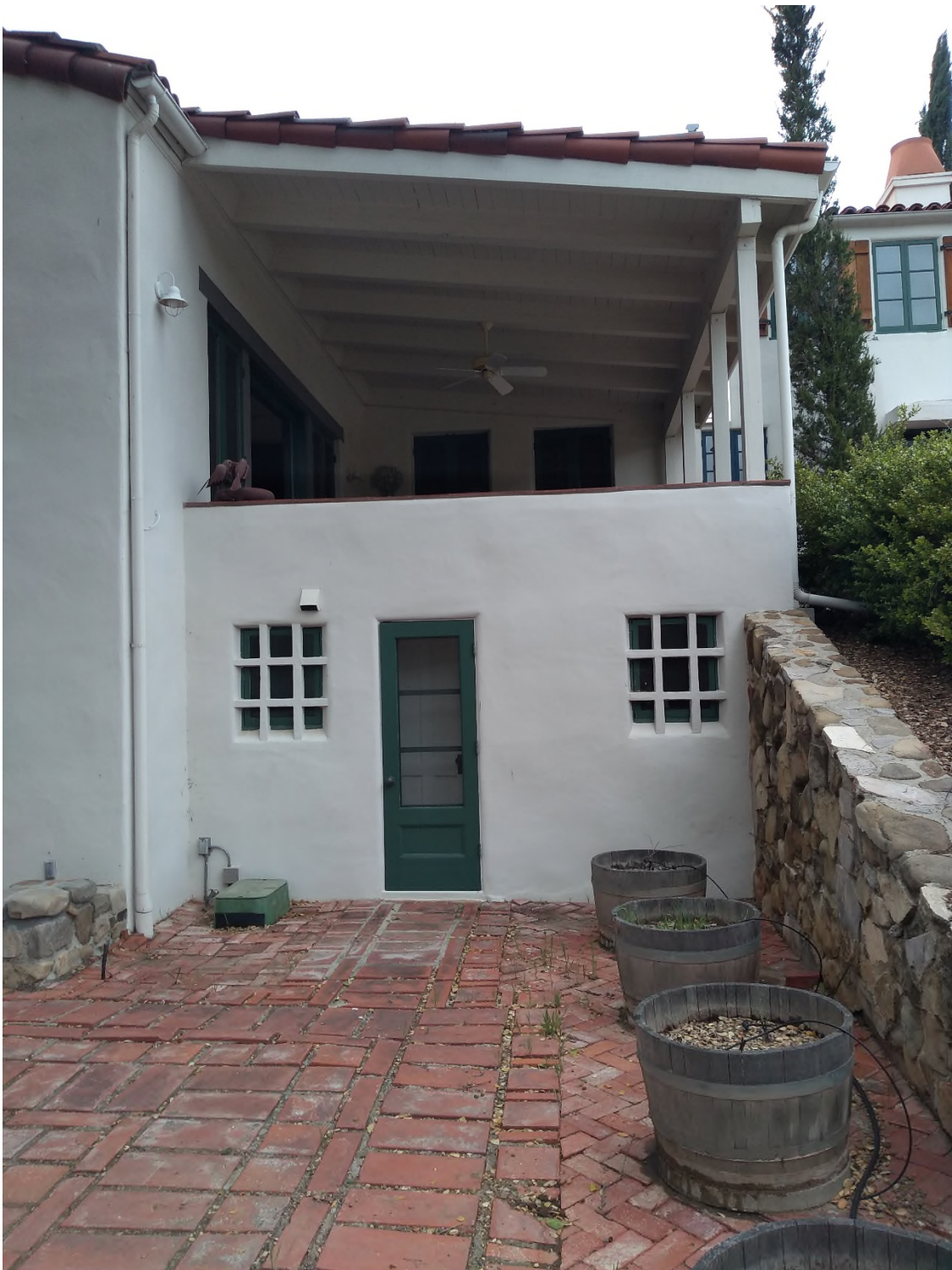
Photograph 11, South Elevation, rear of house, detail of basement entry, looking north
