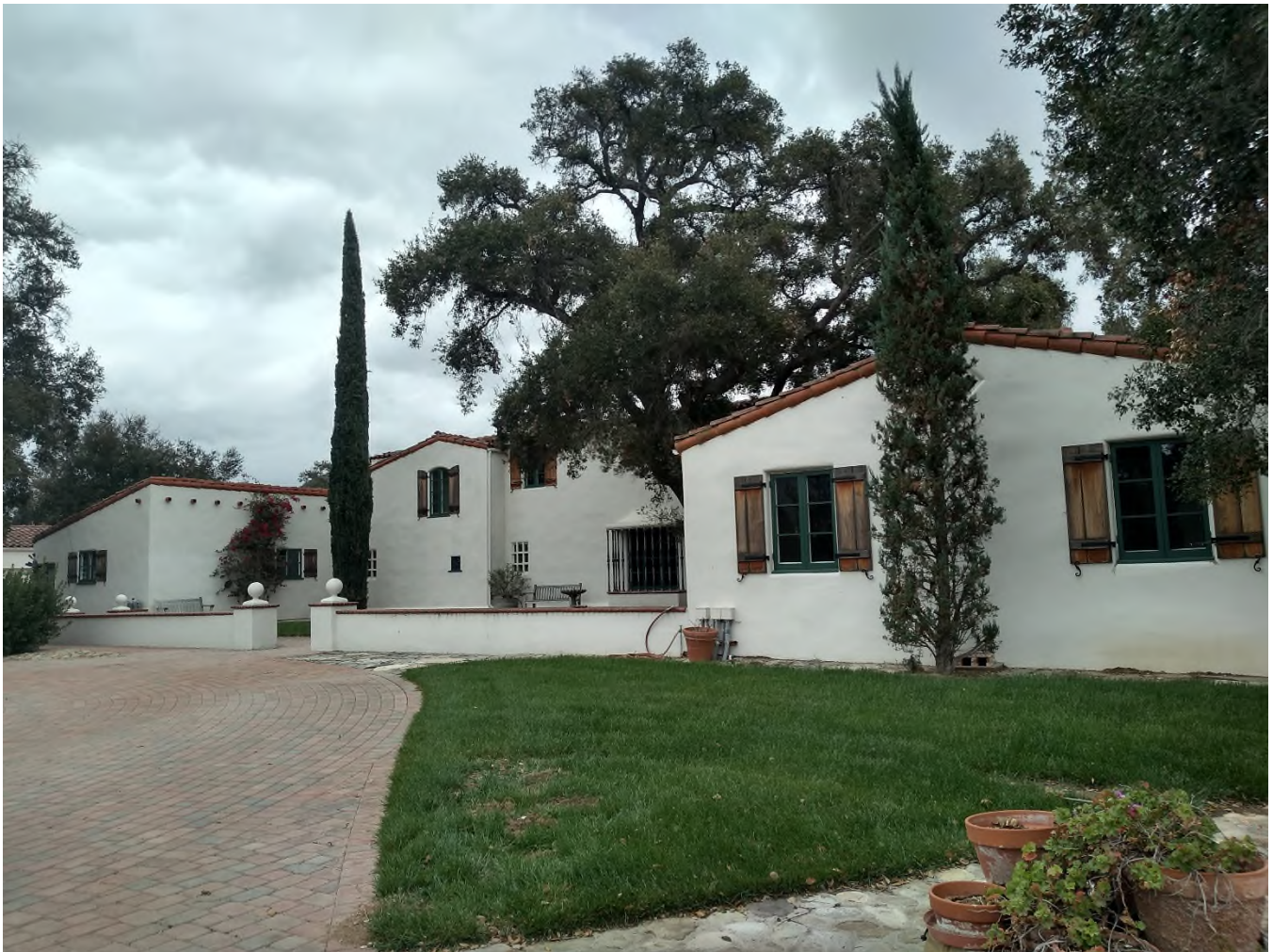
Photograph 2, North Elevation with entry courtyard, existing conditions, looking southeast
