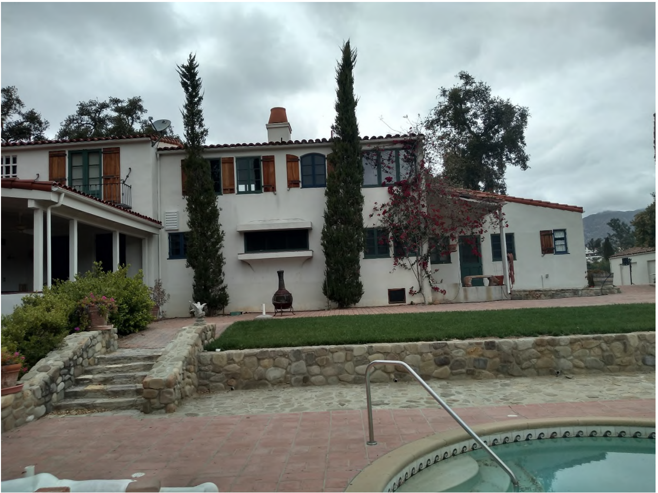
Photograph 7, South Elevation, rear of house, east end of the elevation, existing conditions, looking north
