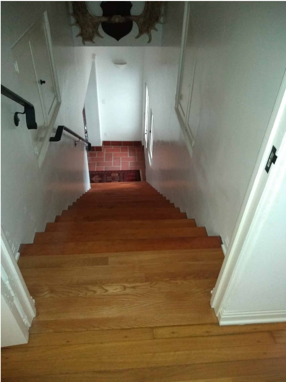
Photograph 29, Stairs to basement level, existing conditions
