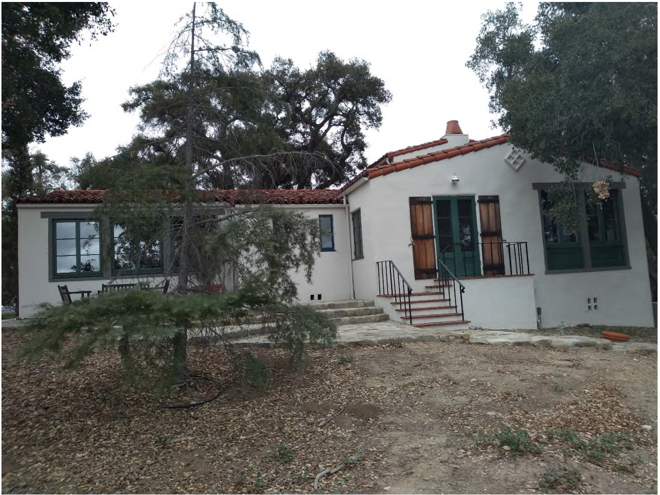
Photograph 16, West Elevation, north end, existing conditions, looking east
