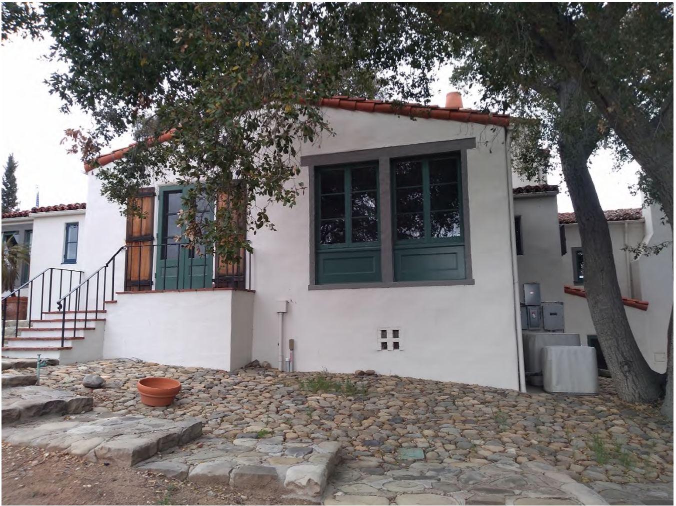
Photograph 17, West Elevation, central section of elevation, existing conditions, looking east
