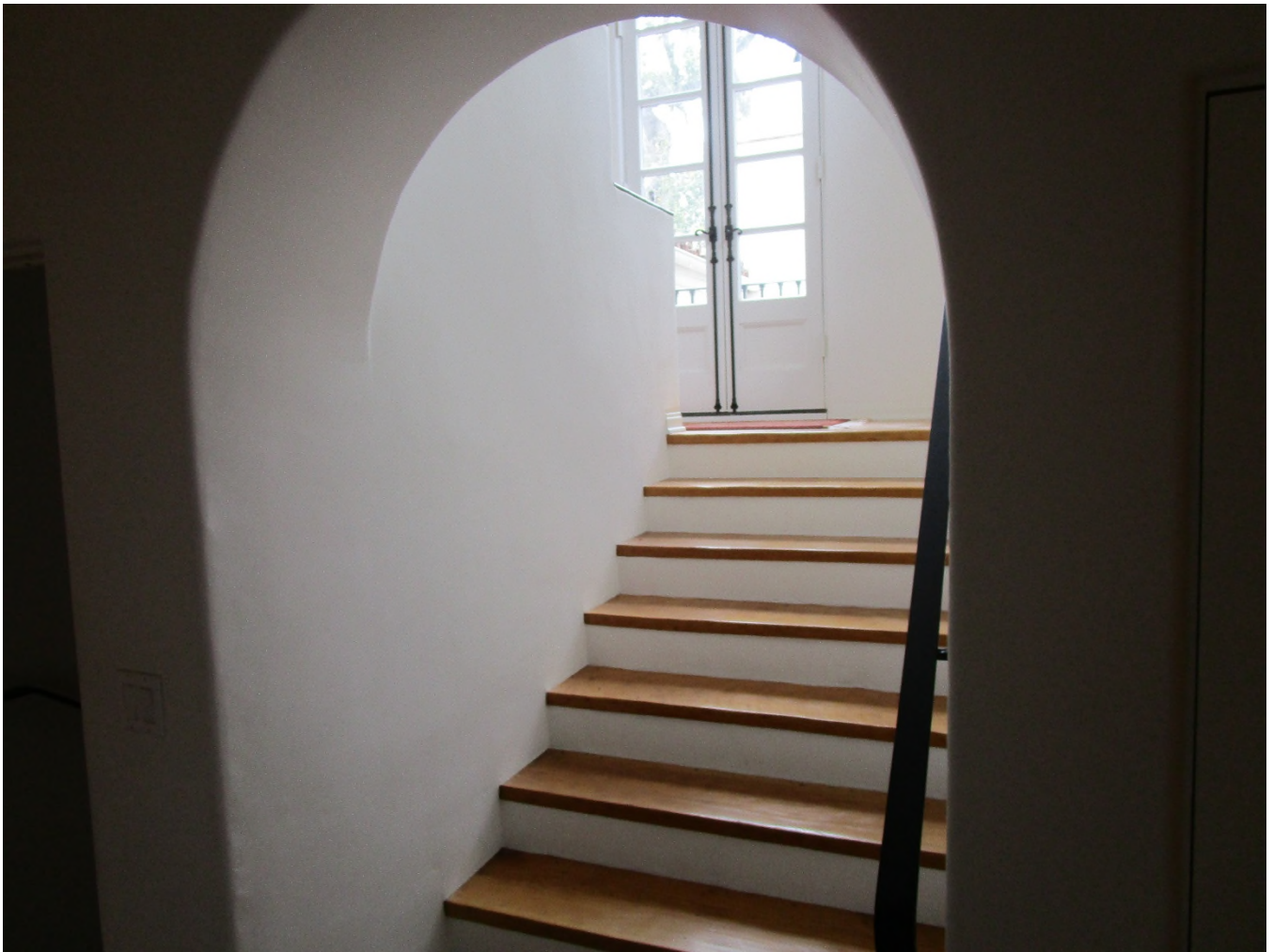
Photograph 28b, Stairway to second floor, existing conditions
