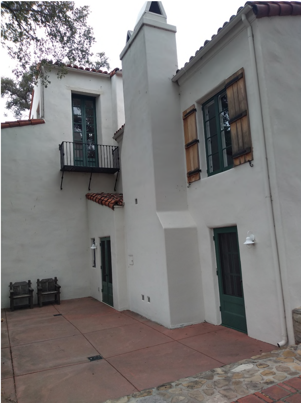
Photograph 18, West Elevation, south end of elevation, existing conditions, looking north
