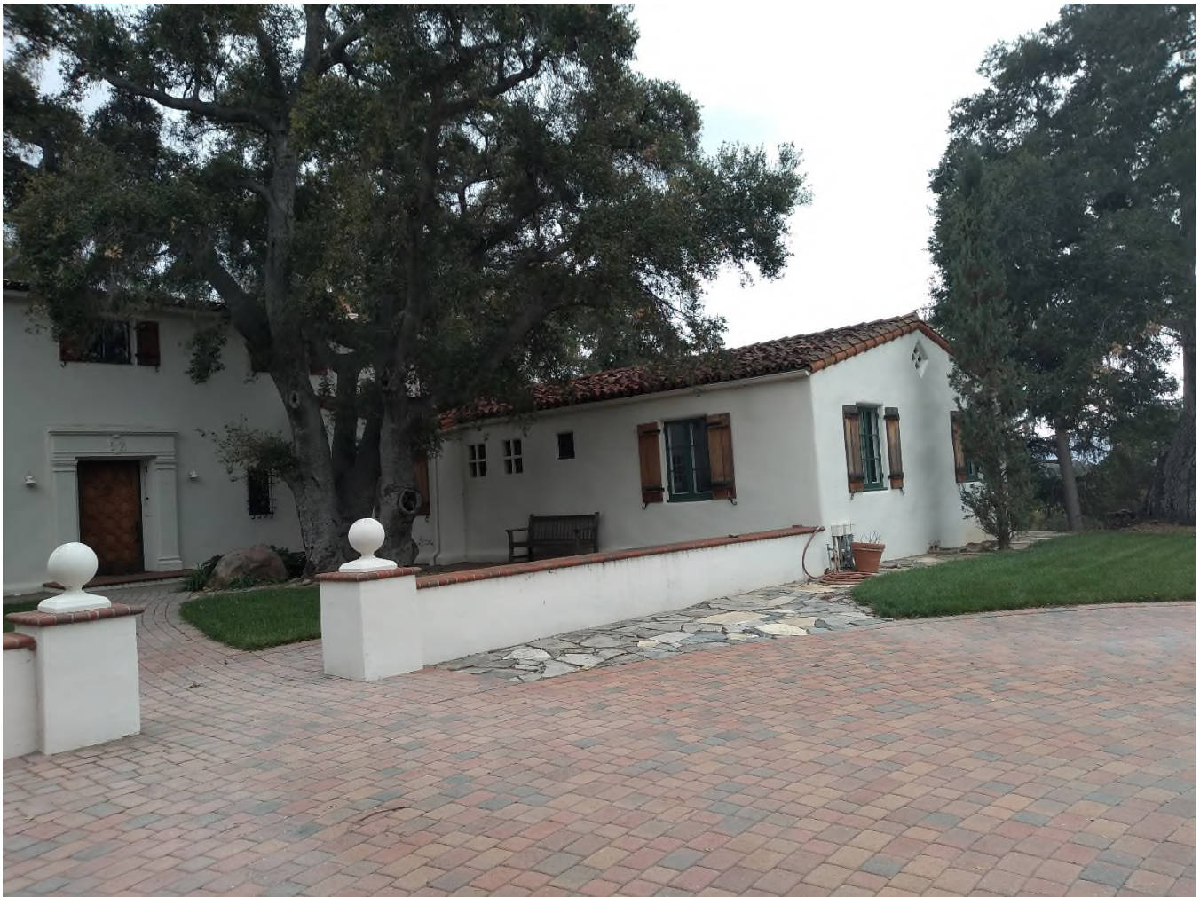
Photograph 4, West side of the North Elevation, existing conditions, looking southwest
