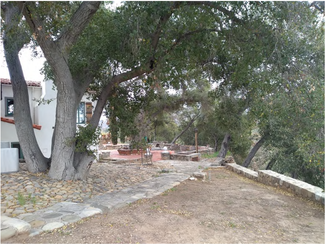
Photograph 37, Rear Terrace, detail of paving and retaining wall on right, existing conditions, looking east
