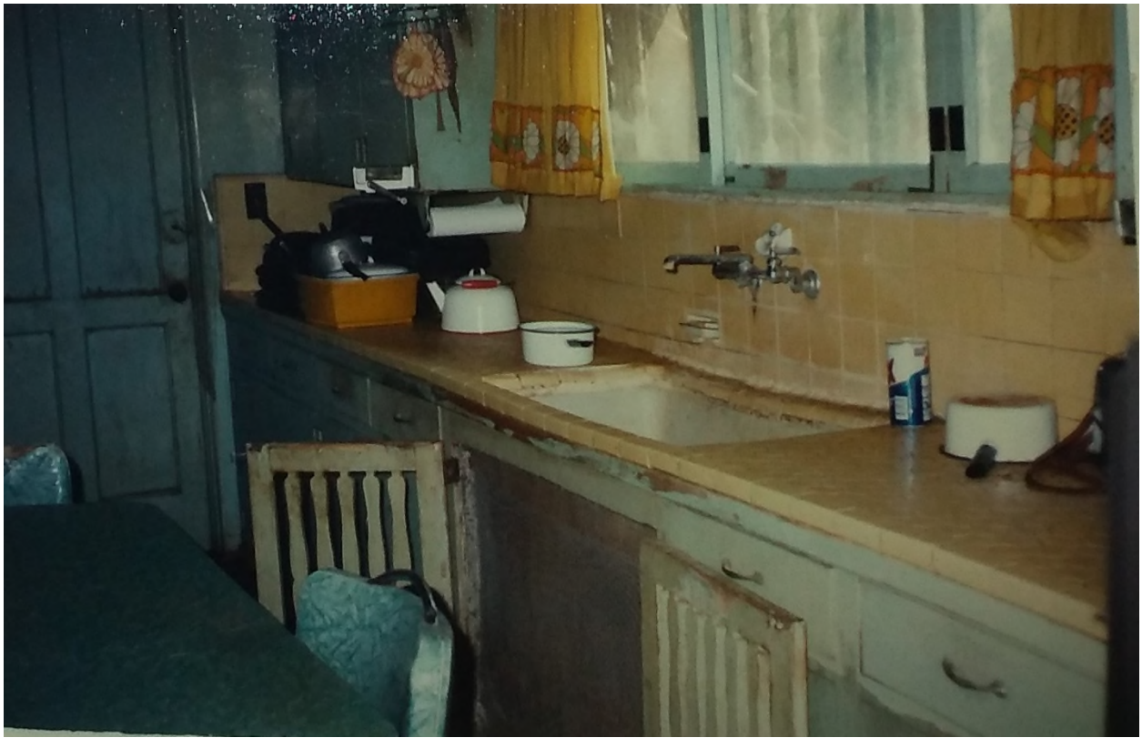
Figure 12, Interior, kitchen in 1988
