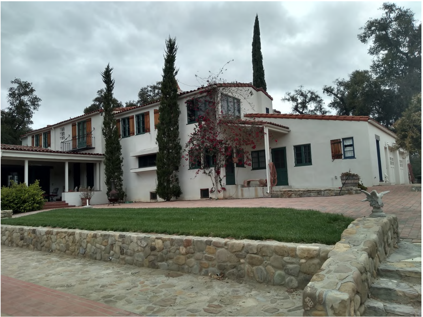
Photograph 8, South Elevation, rear of house, existing conditions, looking northwest
