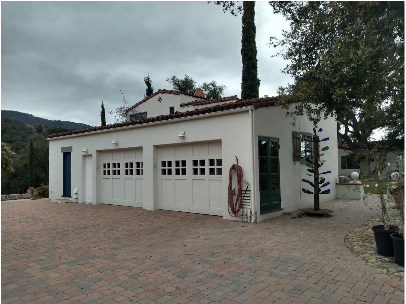
Photograph 15, East Elevation, garage bays attached to house, existing conditions, looking southwest
