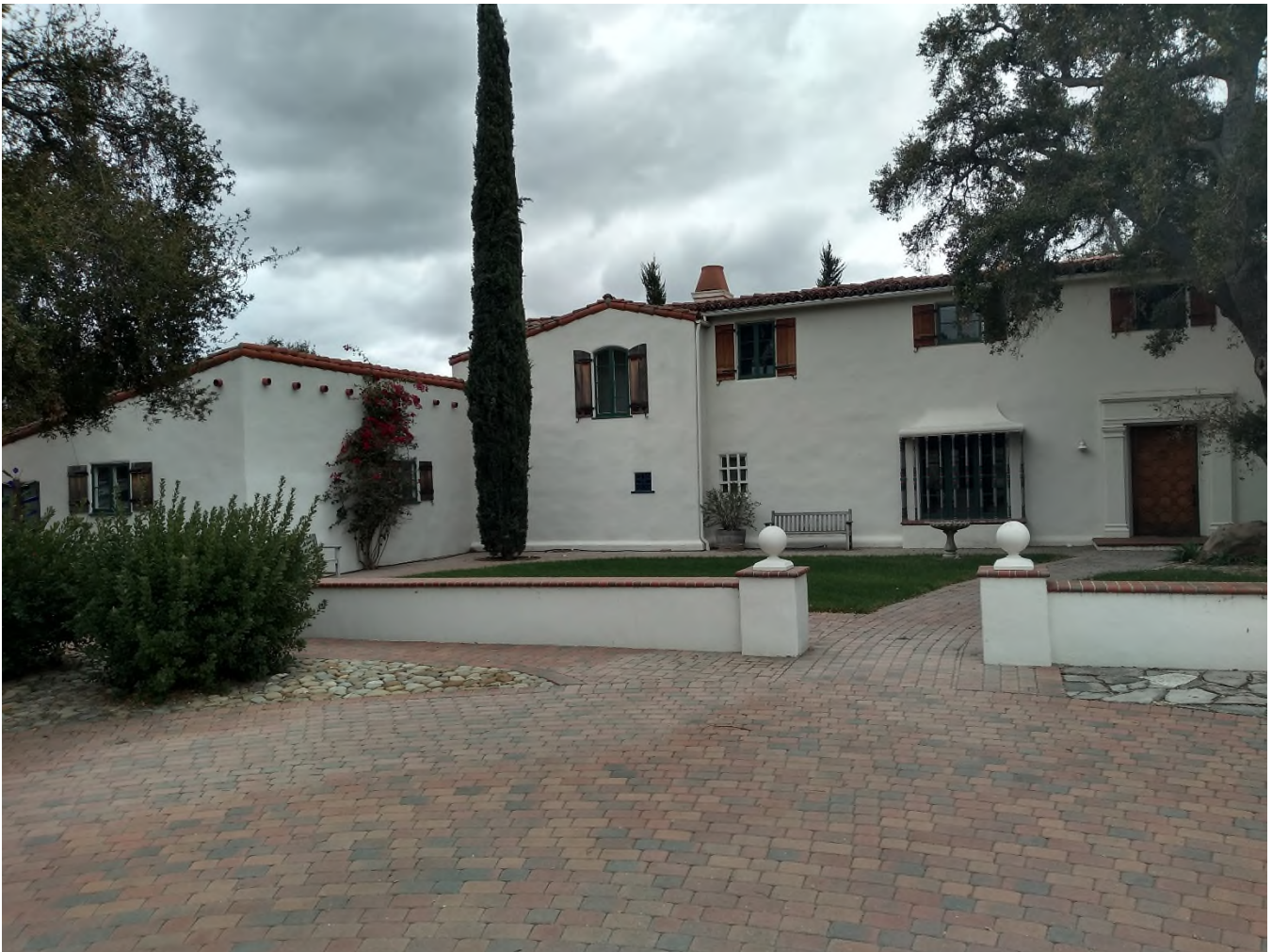
Photograph 5, North Elevation, east end of the elevation, existing conditions, looking southeast
