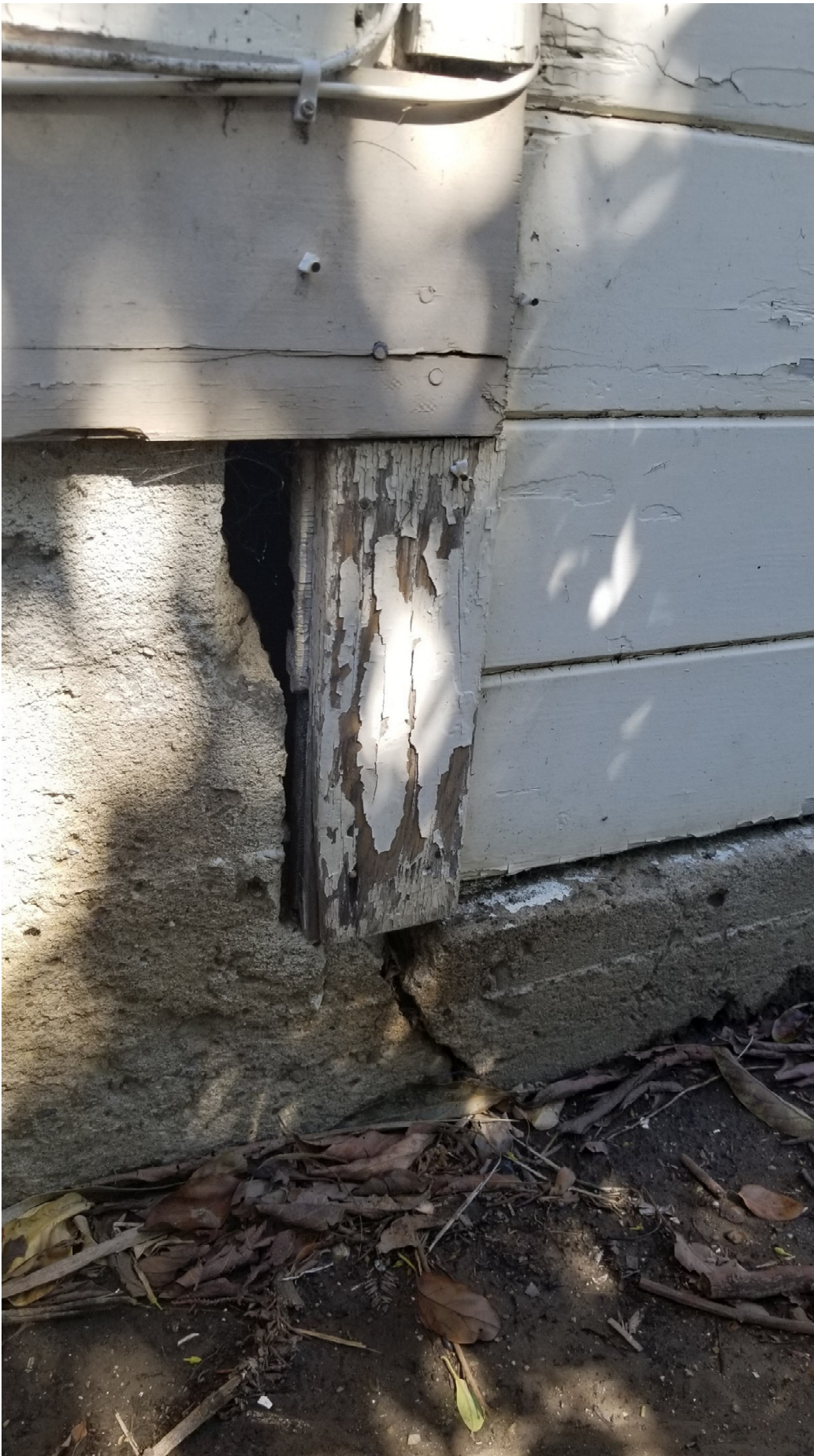
TYPICAL CONCRETE FOUNDATION WALL CONDITION
