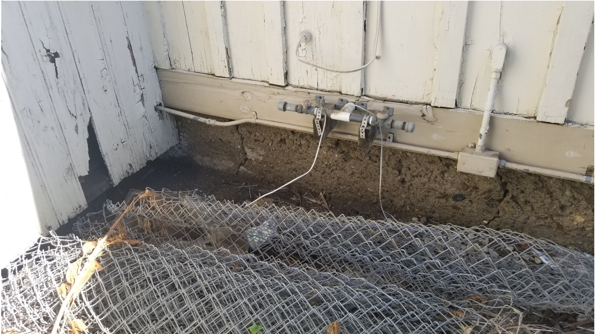
TYPICAL CONCRETE FOUNDATION WALL CONDITION
