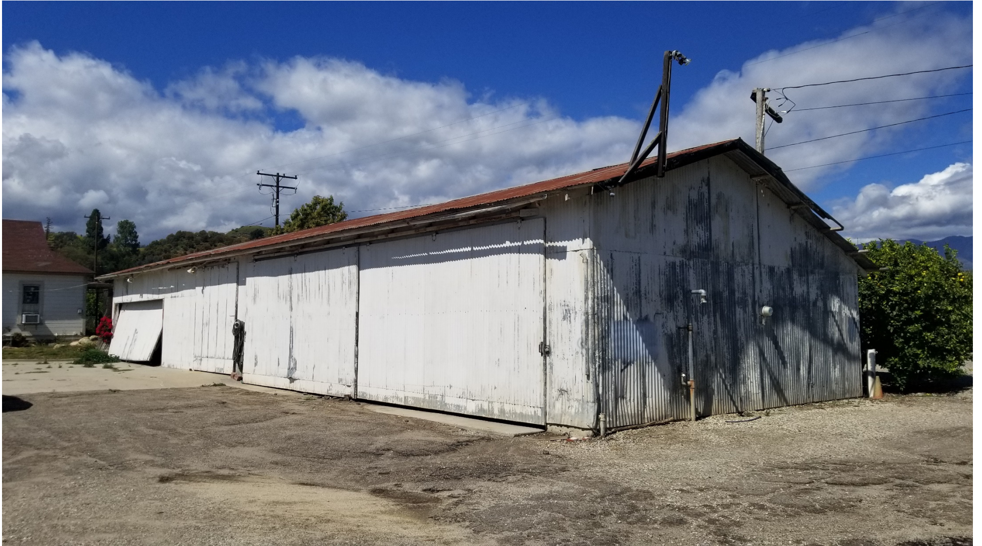
SOUTHWEST CORNER OF CORRUGATED METAL GARAGE BUILDING
