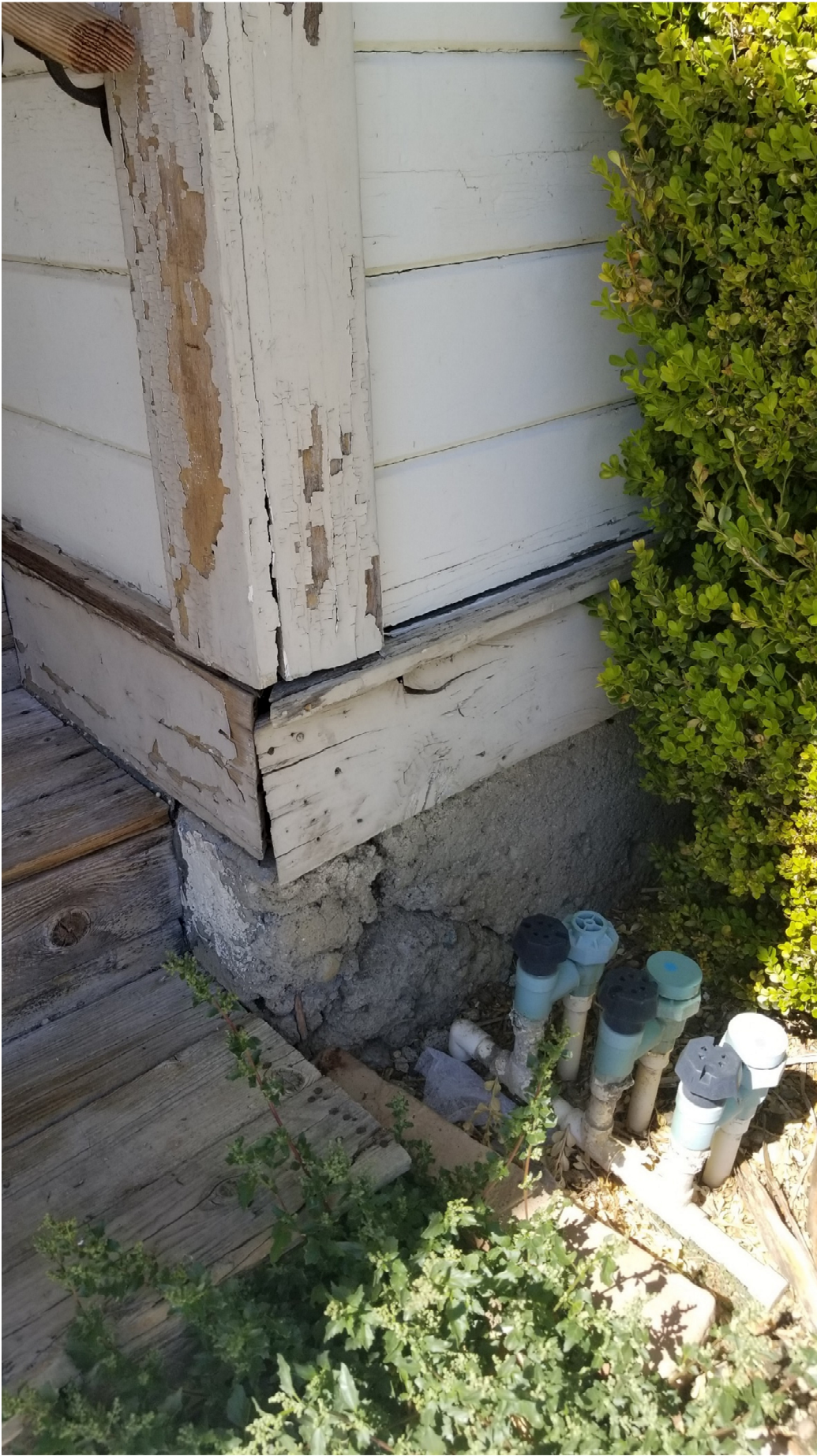
TYPICAL CONCRETE FOUNDATION WALL CONDITION
