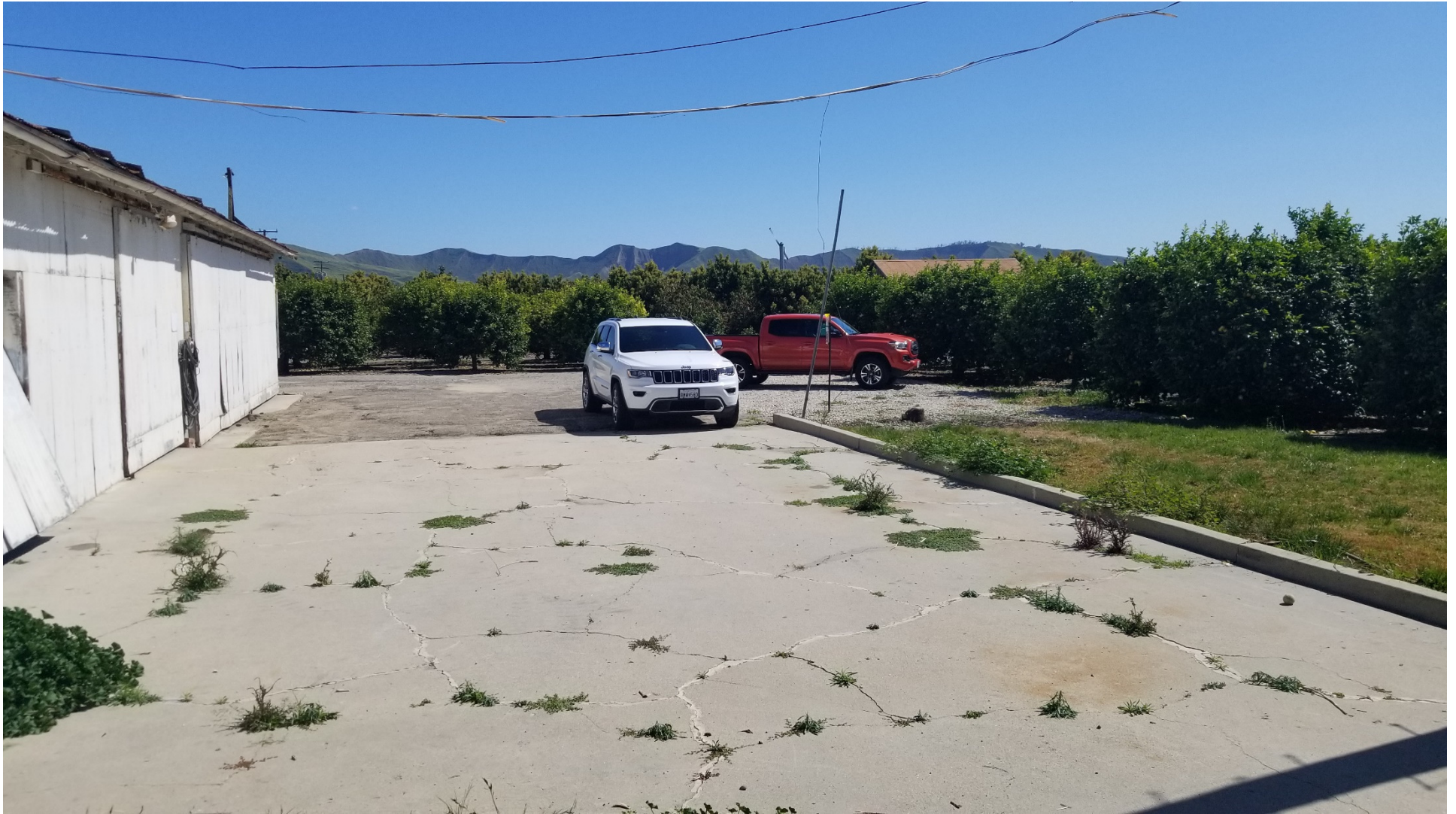
CONCRETE DRIVEWAY/PARKING AREA
