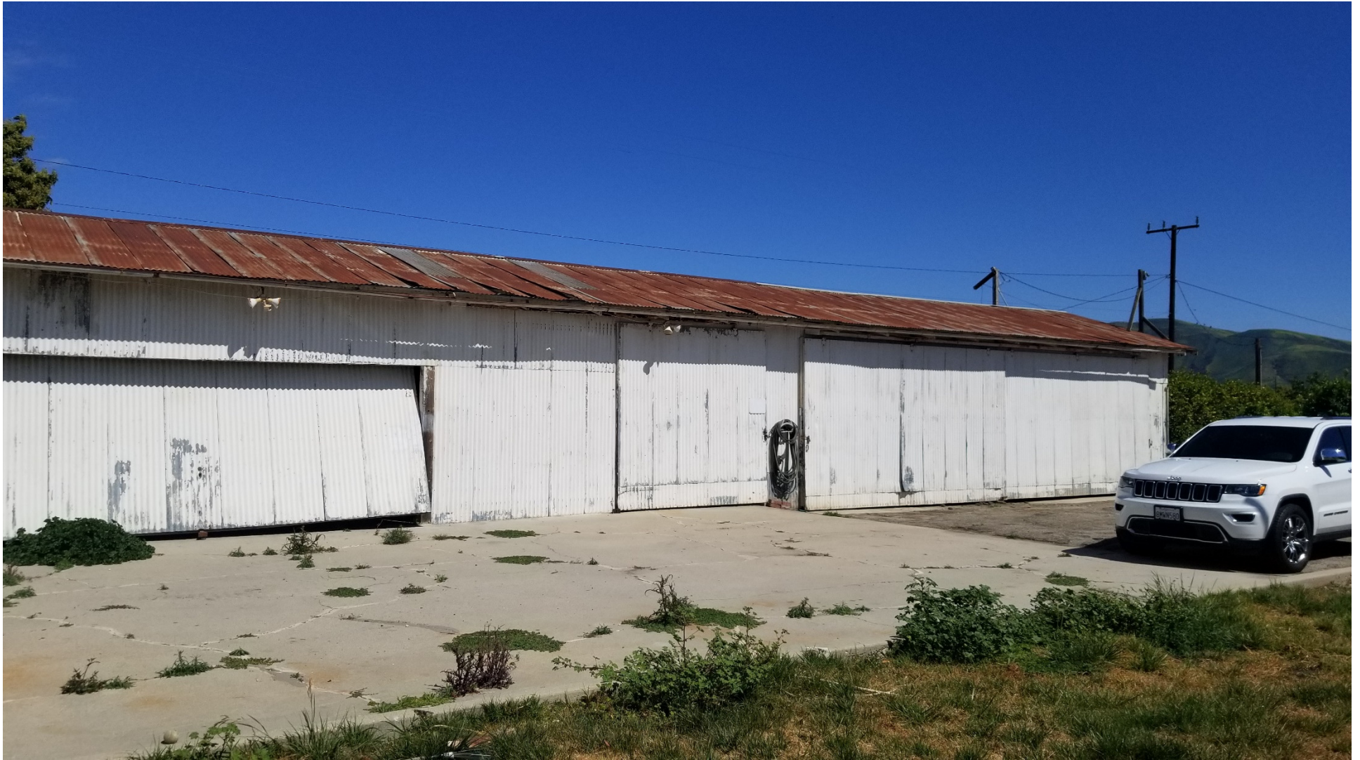
CORREGATED METAL GARAGE BUILDING
