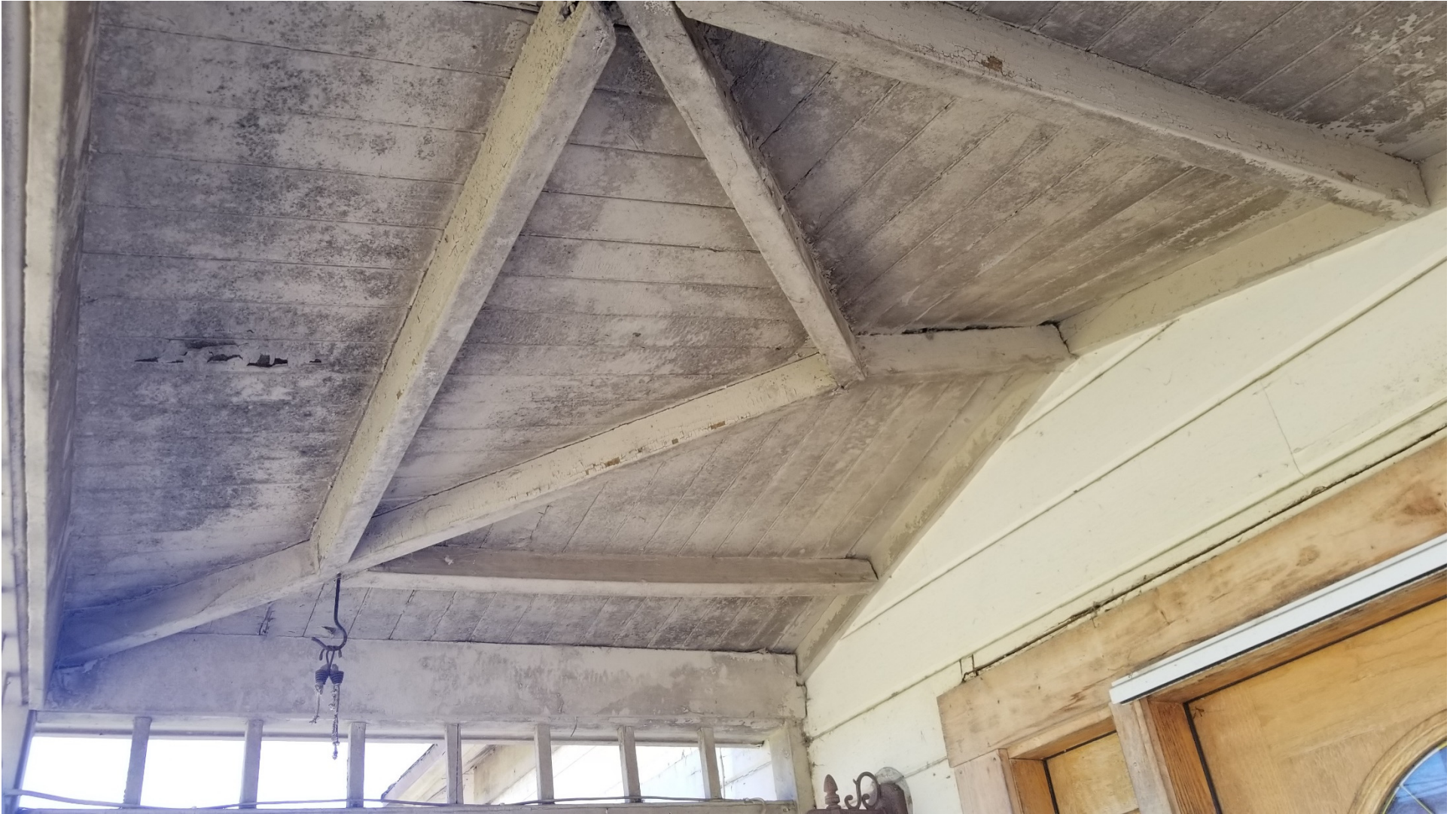
FRONT PORCH ROOF
