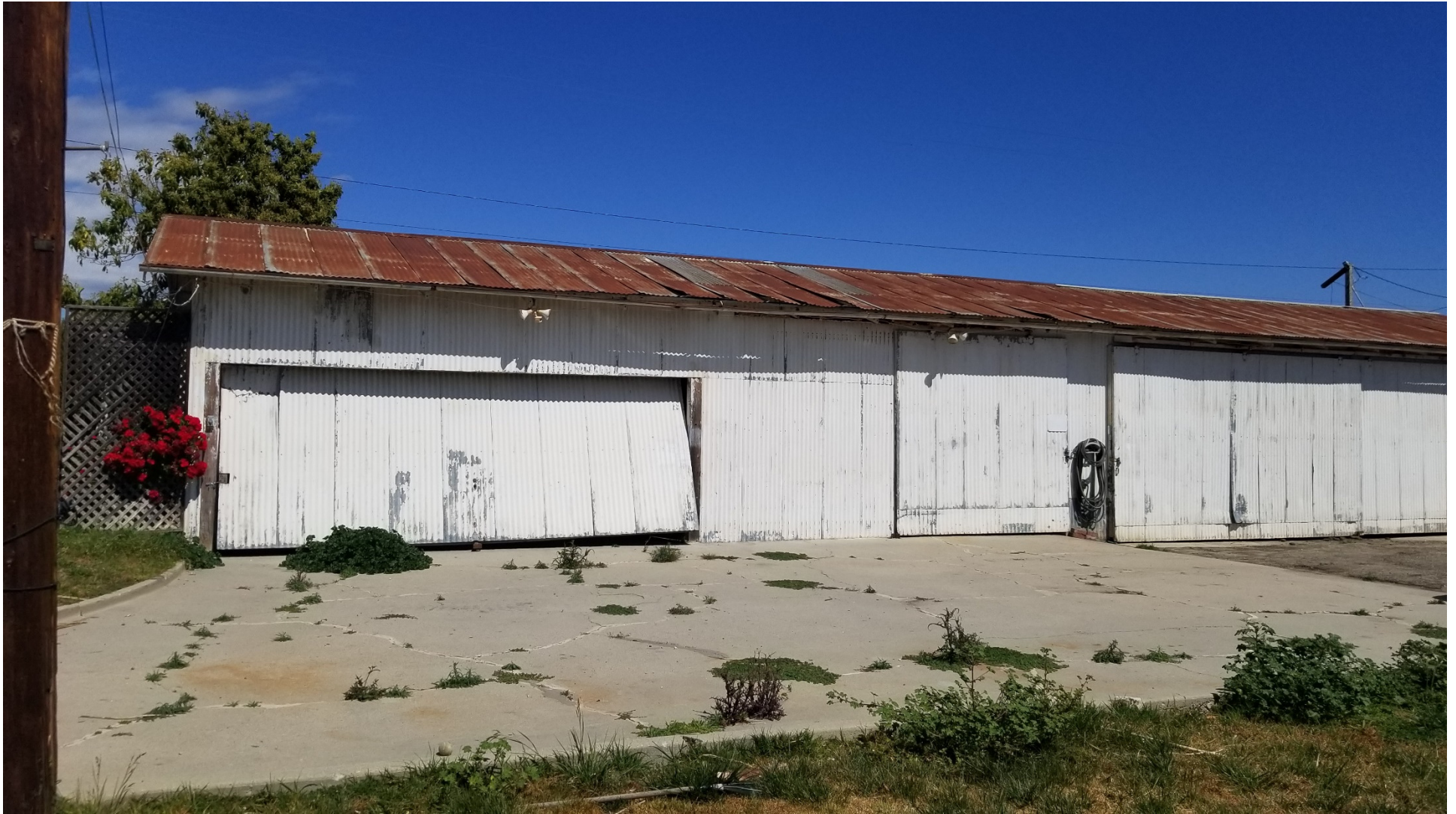
NORTHWEST CORNER OF CORRUGATED METAL GARAGE BUILDING
