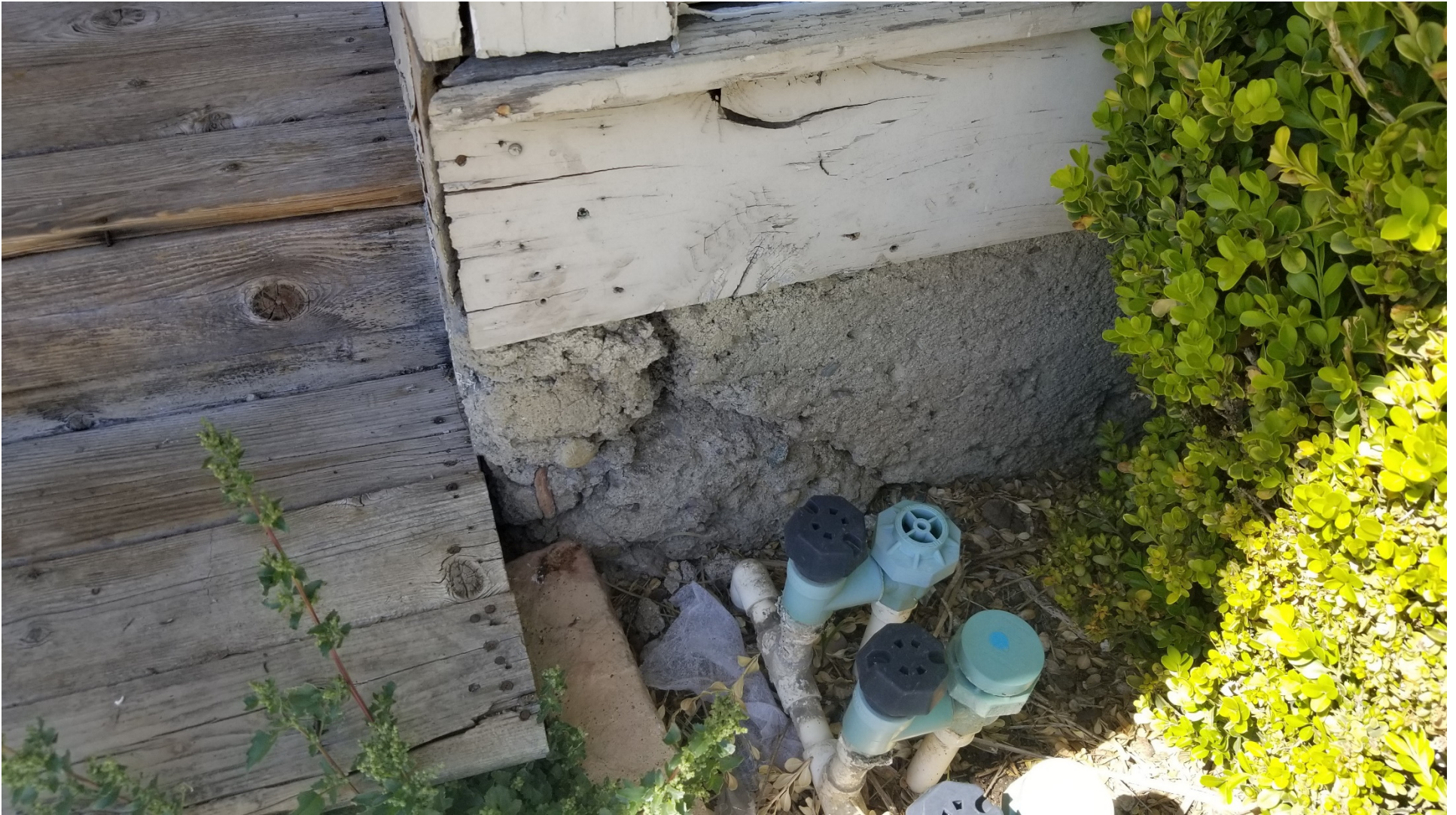
TYPICAL CONCRETE FOUNDATION WALL CONDITION
