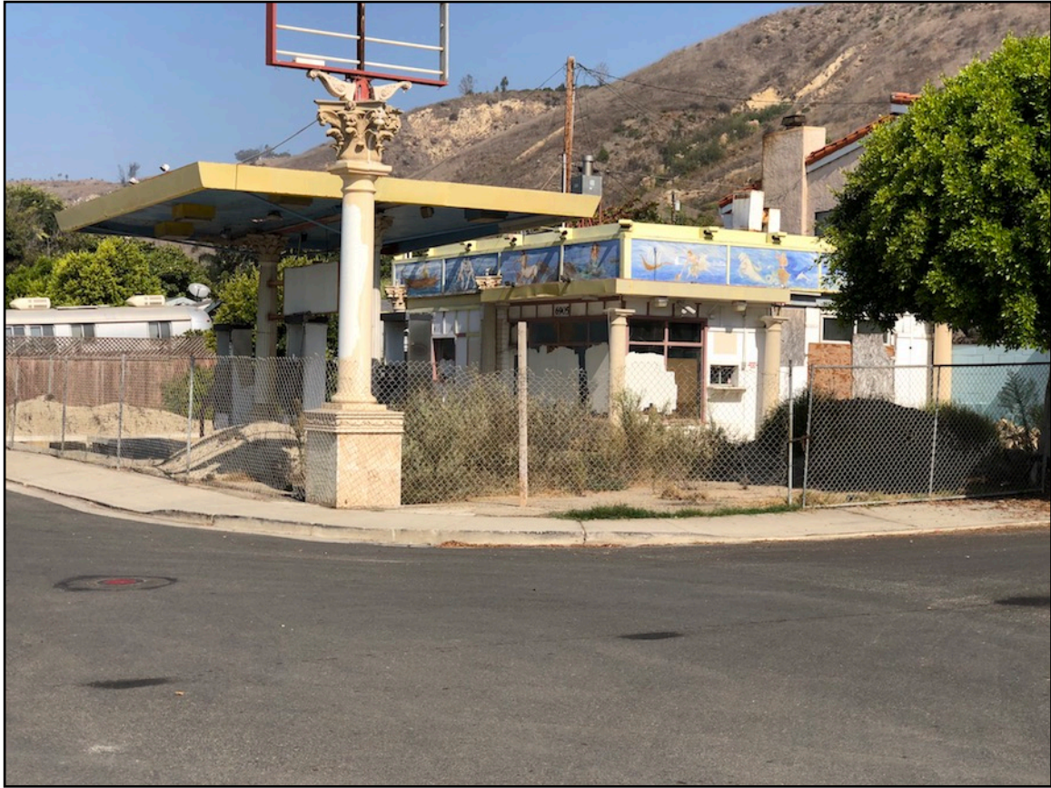
Photo 1. Property viewed from southeast. [10-10-2019]
