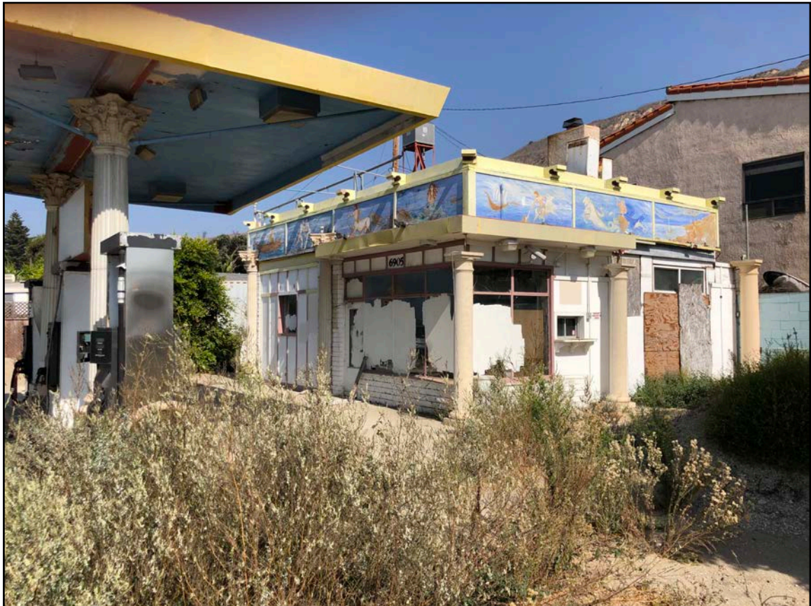
Photo 2. Southern and eastern elevations. [10-10-2019]
