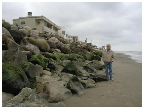
Photograph Dated 4/4/2002. Red Mark on the rock is elevation 4.5' MSL. Feet of man standing on the beach are at approximately 0.0' MSL
