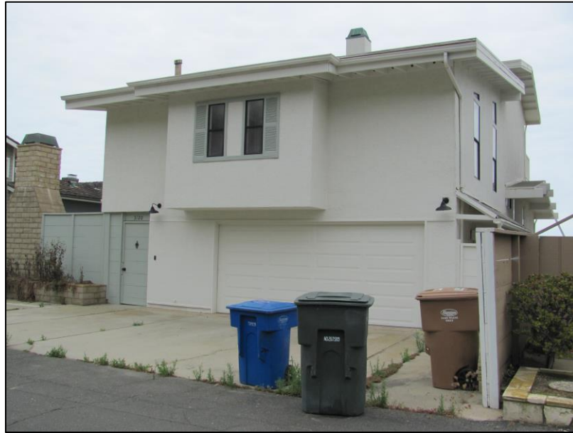
Figure 1-1: Site Photo of the Subject Building May 10, 2023
