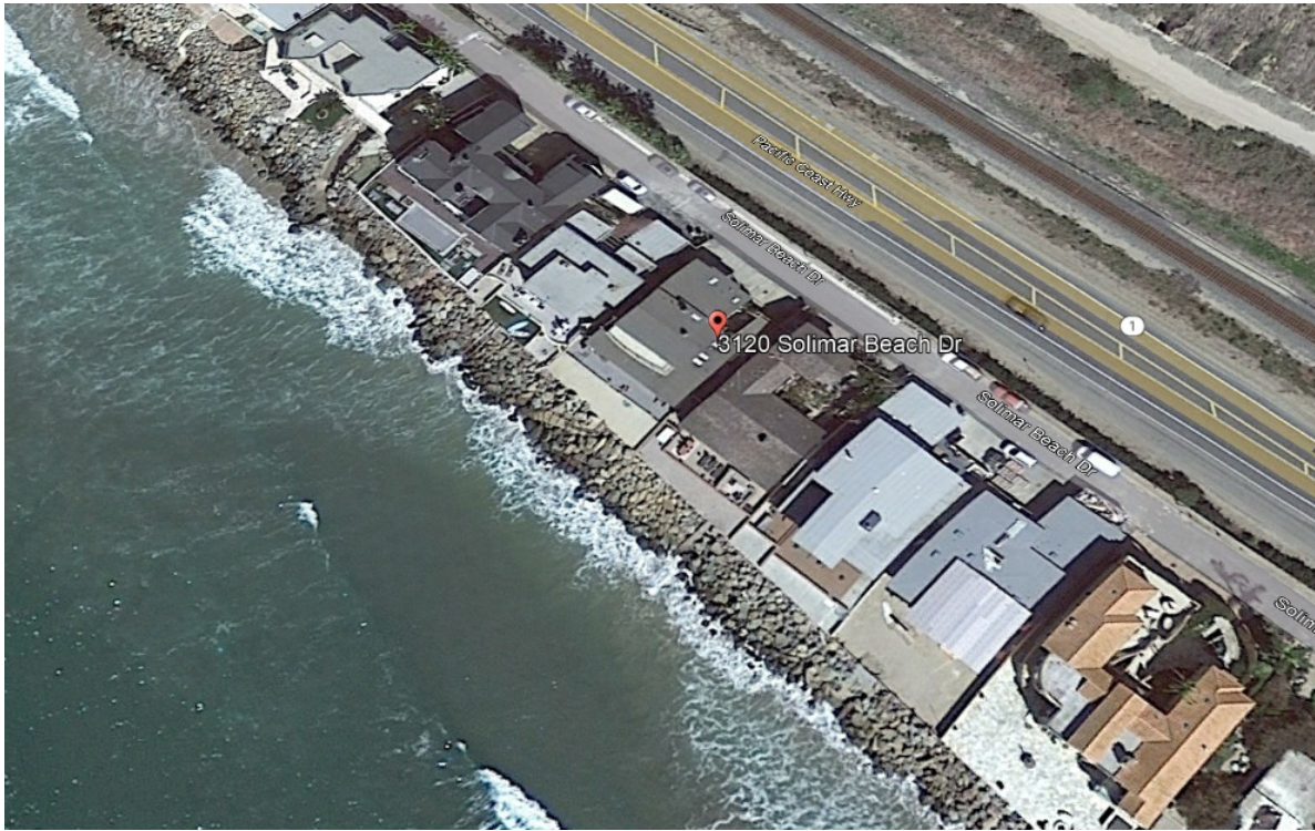
Photograph 1. Subject site and shoreline in 2020. Note the continuous community revetment fronting the properties.
