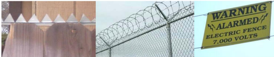
Examples of Prohibited Fencing
