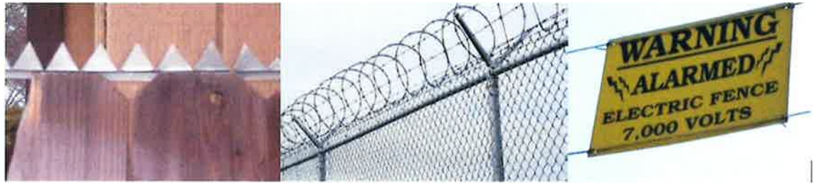
Examples of Prohibited Fencing
