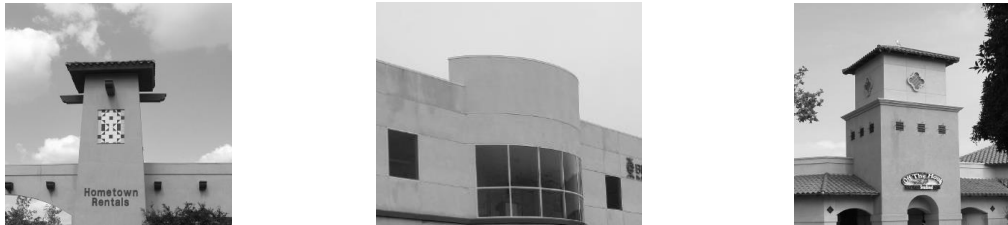
Examples of Building-Concealed Wireless Communication Facilities
