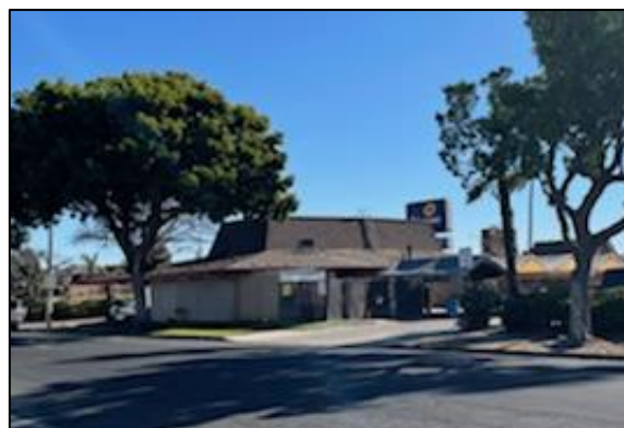
Project Homekey Site in Oxnard
