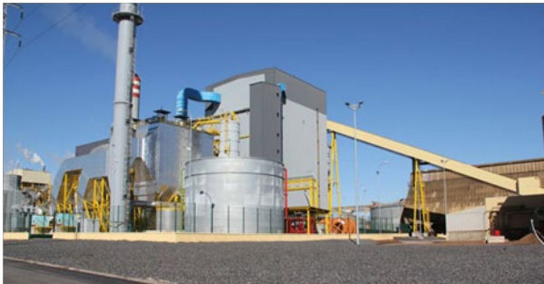
A 50 MW Biomass Power Plant
