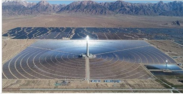
A 50 MW Solar Concentration Array
