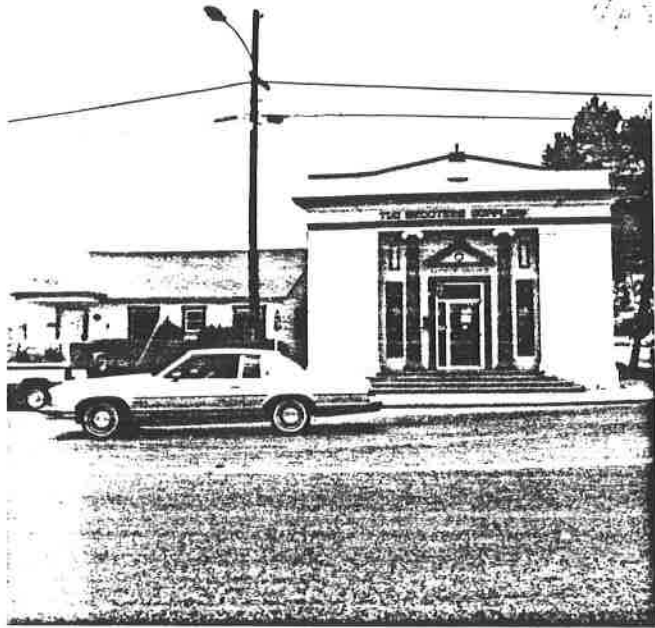
VIEW LOOKING SOUTH
