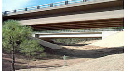
Figure 3.16: Underpass with open field of view for large mammals
