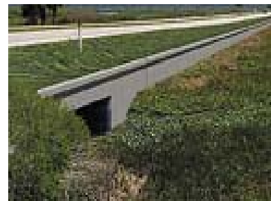
Figure 3.5: Lipped concrete wall
