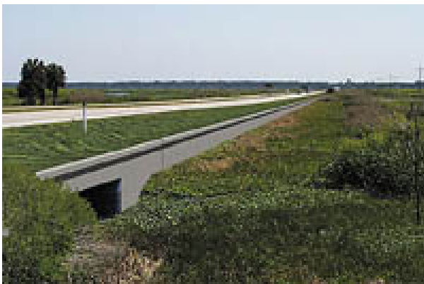
Figure 5.7: Lipped walls for amphibians (Critter Crossings Website, 2002)
