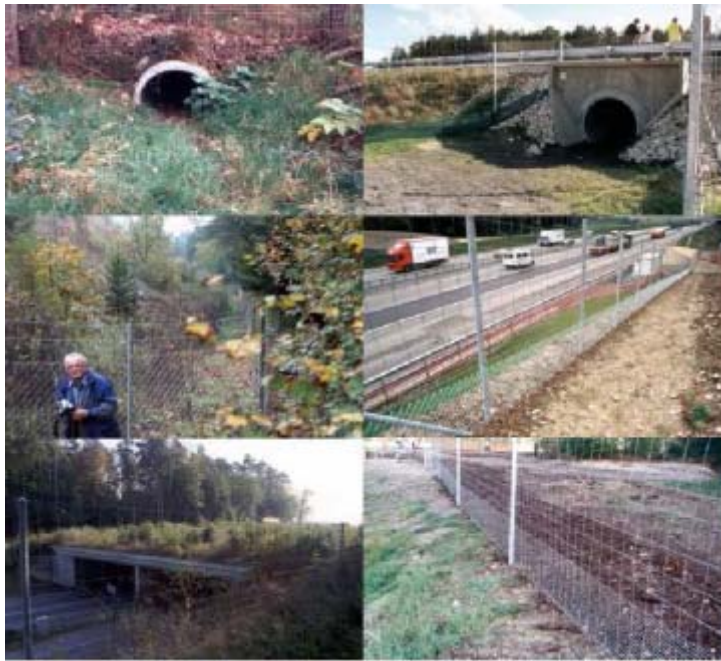
Figure 5.1: Various fence applications in Europe (FHWA/US DOT, 2002)
