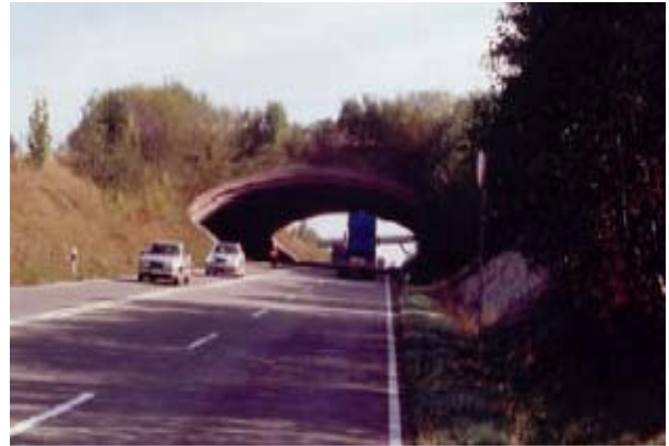
Figure 5.29: Wildlife overpass (Deer-Vehicle Crash Information & Research Center)
