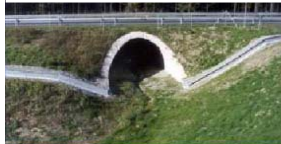
Figure 3.8: Arch culvert with fence for large mammals and lipped wall for amphibians
