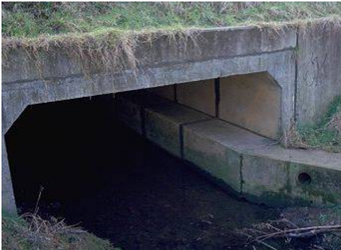
Figure 5.22: Box culvert modified with ledge for small animal passage (Jackson, 2004)
