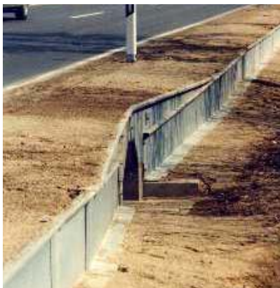
Figure 5.11: Amphibian tunnel (Maibach, 2004)
