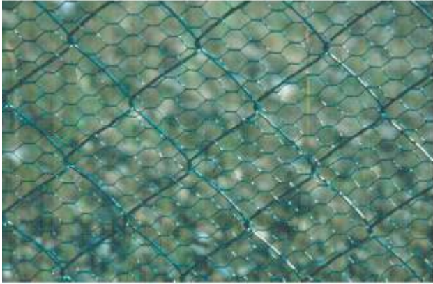
Figure 5.4: Chain link fence for large animals overlaid with fine plastic mesh fencing for small animals and amphibians (Puky, 2003)
