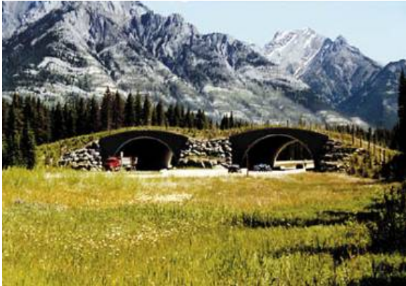
Figure 5.28: Overpass in Banff National Park, Canada (CPAWS, 2004)
