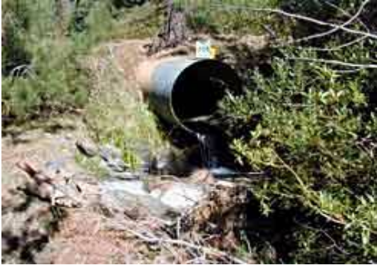
Figure 5.41: Perched pipe.
