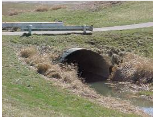
Figure 5.42: Culvert with standing water.
