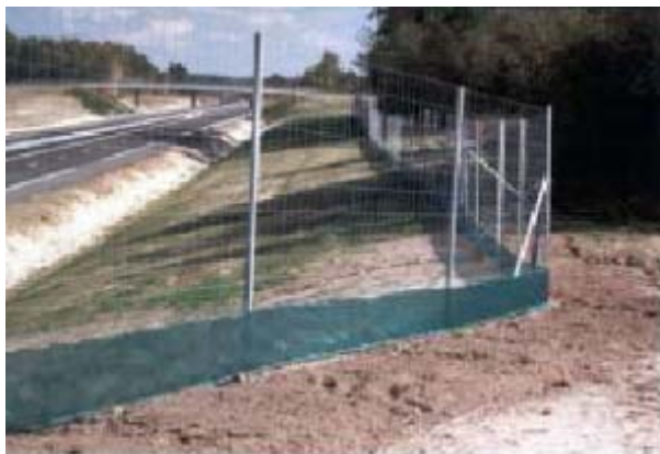
Figure 5.2: Wide mesh chain fence for large mammals, with a fine mesh fence border for small mammals and amphibians (FHWA/US DOT, 2002)
