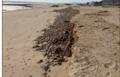
Beach erosion at surfers point in the City of Ventura.
