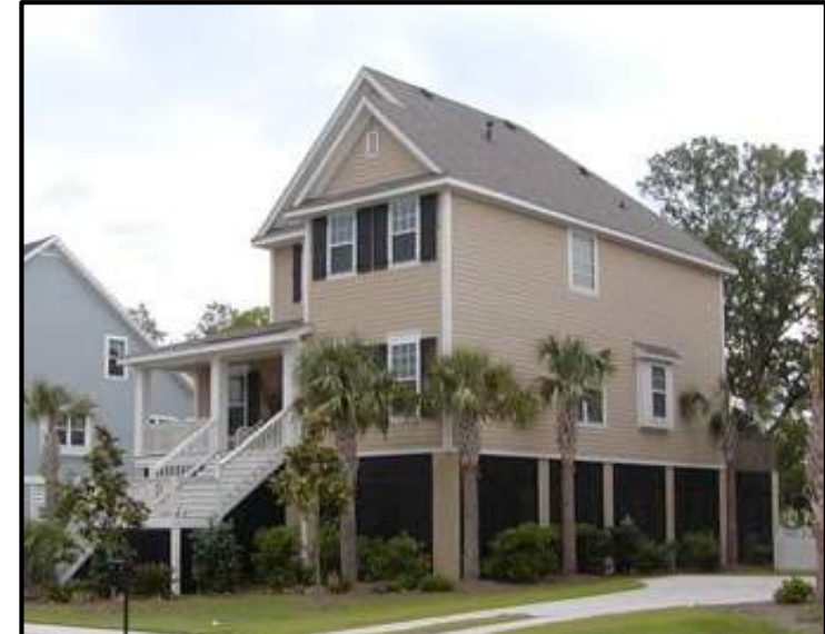
Design to Accommodate Flooding
