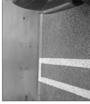
These parking stalls use pervious concrete which allows for water infiltration; the drive aisles are made with traditional asphalt. The County has high expectations for stormwater management in parking areas. Section 8108-5.9
