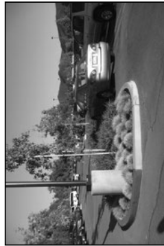
Light poles MAY NOT be located in finger planters (as pictured above), end row planters (below) or tree wells.
