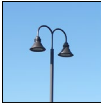
Full cut-off lighting prevents light from going above the horizontal plane in order to minimize lighting of the dark night sky. All new lighting fixtures in parking areas must be full cut-off. Sec. 8108-5.12(e)
