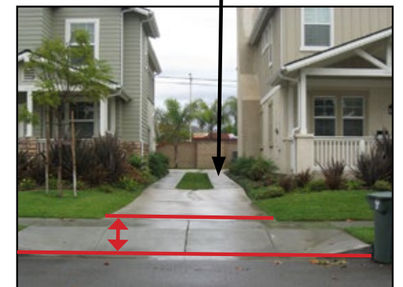
The portion of driveways in the public right-of-way. Width requirements are per the Ventura County Road Standards.
