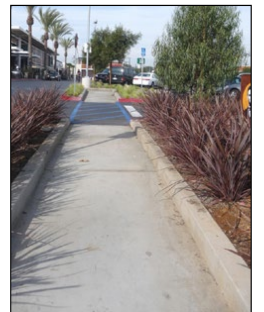
A safe and direct pedestrian pathway must be provided from the street to the primary building entrance. Section 8108-5.4.2
