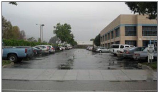
This excessively wide drive aisle wastes space and creates an unnecessary amount of impervious surface. Drive aisle and parking space dimensions may not be exceeded without Planning Director approval.
