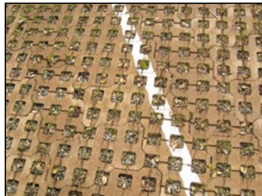
Interlocking pavers, blocks, or stones allow water to pass through gaps. Photo below: Tricia Maier
