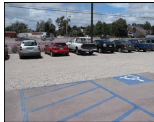
In some cases gravel may be used in parking areas, though this surface may not be used for accessible spaces for disabled persons.
