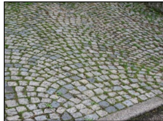
Interlocking pavers, blocks, or stones allow water to pass through gaps. Photo below: Tricia Maier
