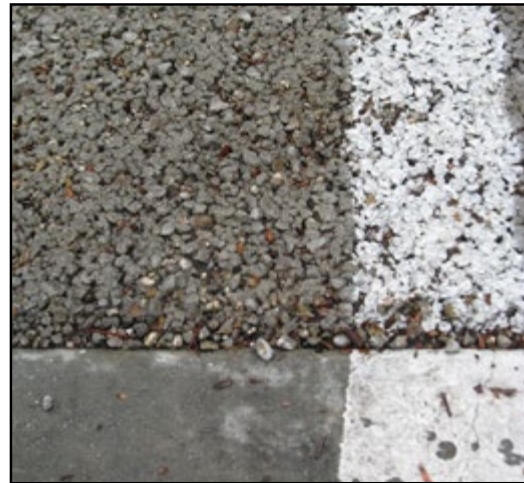
Pervious concrete and asphalt have pore spaces within the material itself which allow water to pass through.
