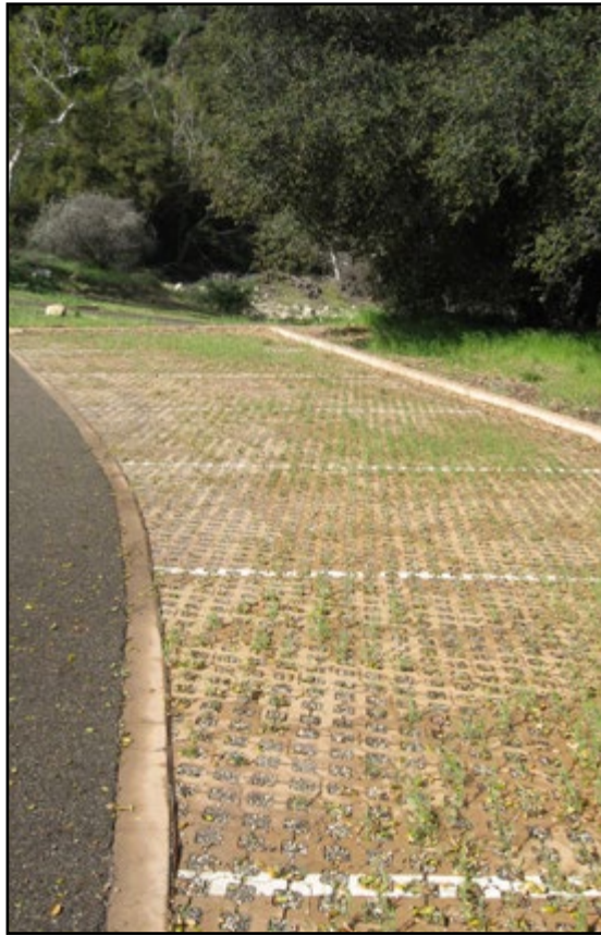
The use of pervious surface materials in parking areas is encouraged, particularly for uses such as campgrounds or retreats where paved surfaces may detract from the natural character of the site. Sec. 8108-5.9
