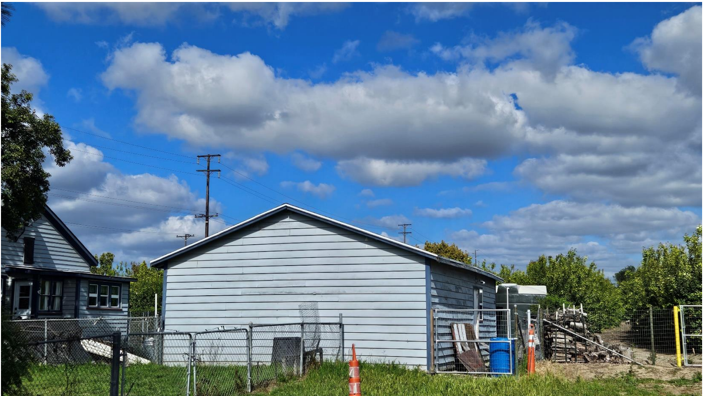
GARAGE SOUTH – WEST SIDES
