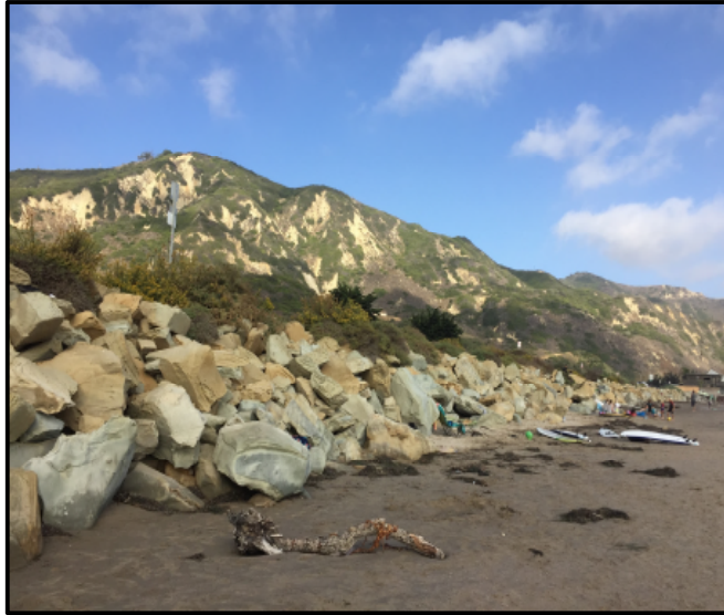
Armor Rock Revetments
