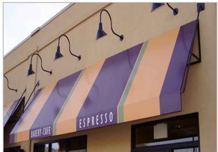
Example of a canopy sign with lighting.
