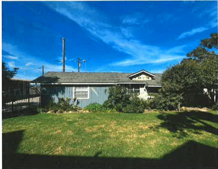
Overview of South Elevation
