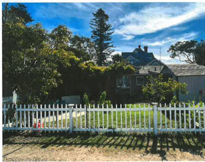
Overview of North Elevation
