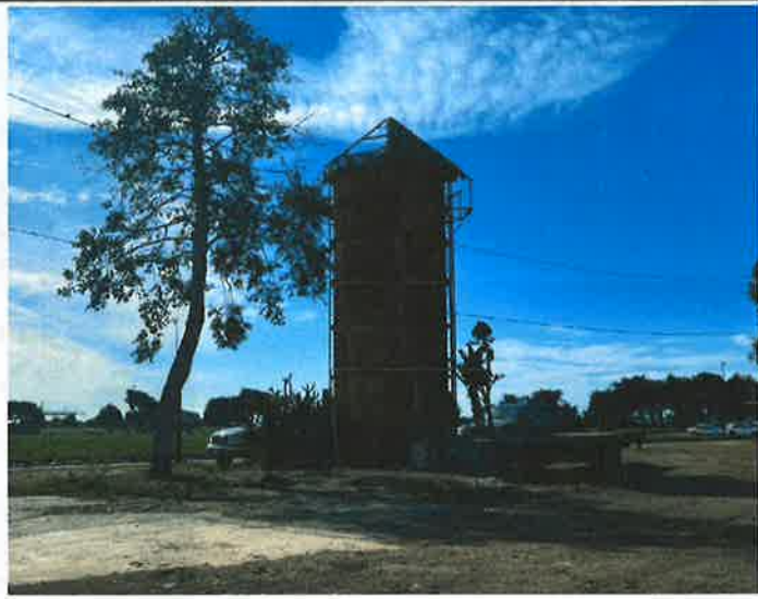
View Facing Southwest
