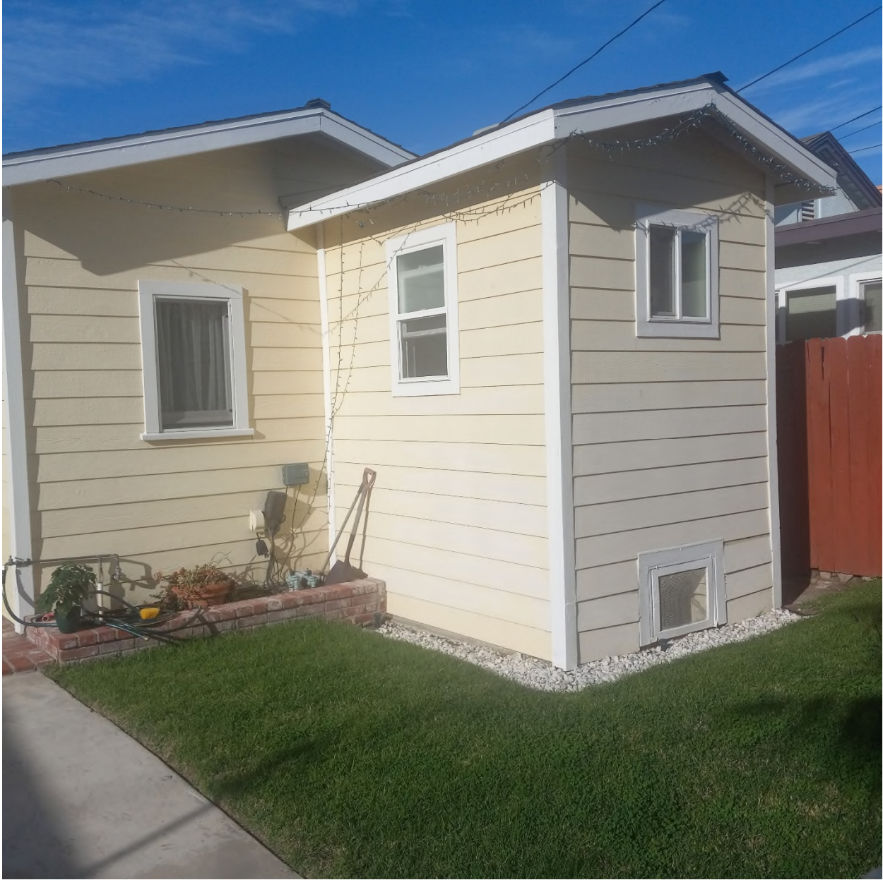
Photograph 16, Looking towards the south elevation of 136 Los Angeles Avenue (December 28, 2023)
