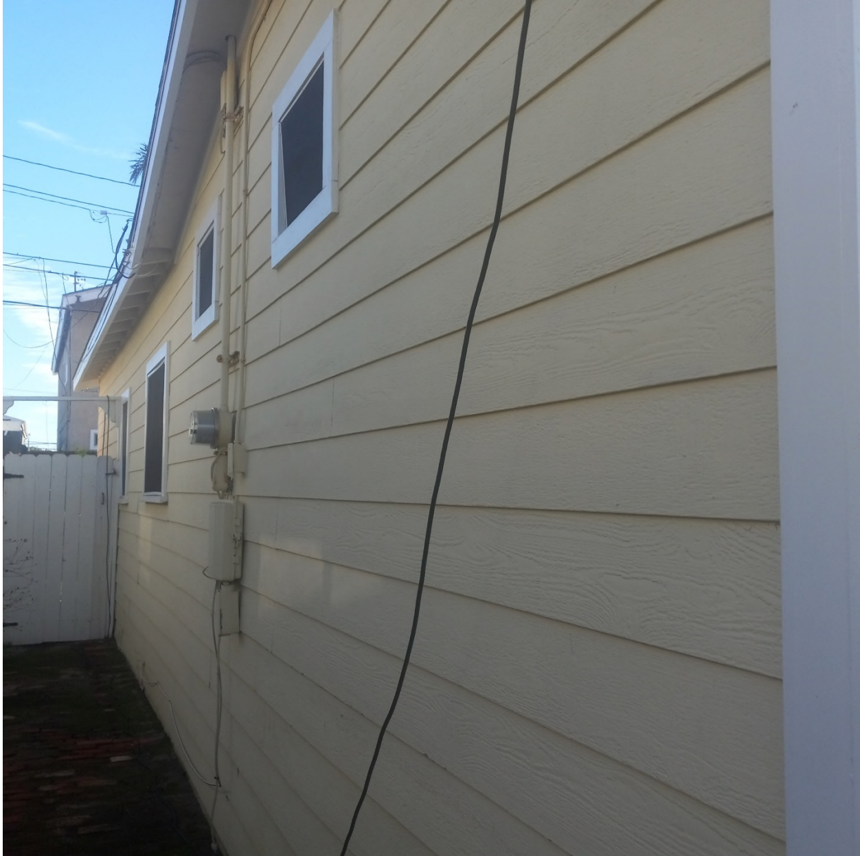
Photograph 18, Looking southwest towards the east elevation of 136 Los Angeles Avenue
