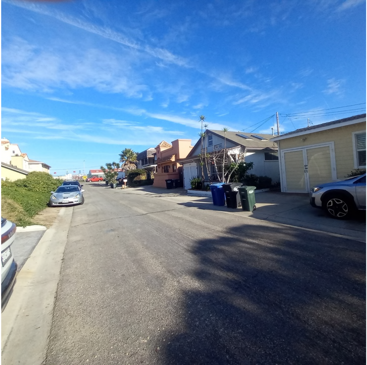
Photograph 6, Looking east towards the north end of Los Angeles Avenue with the northeast end of the north side of the 100 block of Los Angeles Avenue, looking southeast (December 28, 2023)
