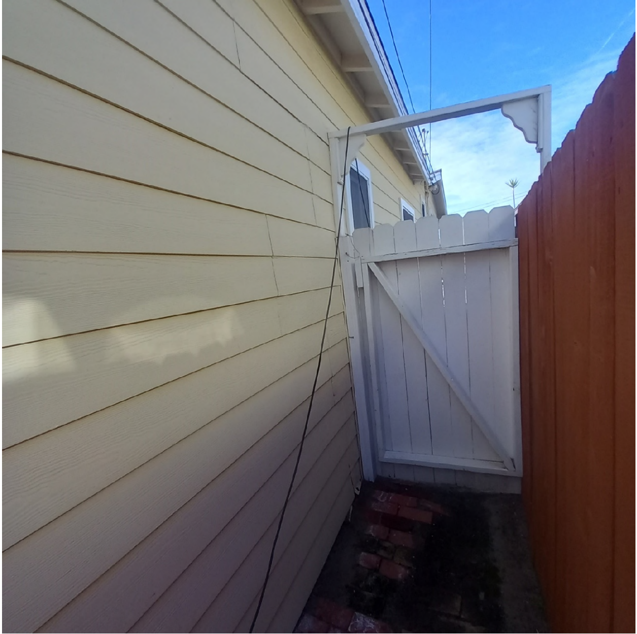
Photograph 17, Looking northwest towards the east elevation of 136 Los Angeles Avenue
