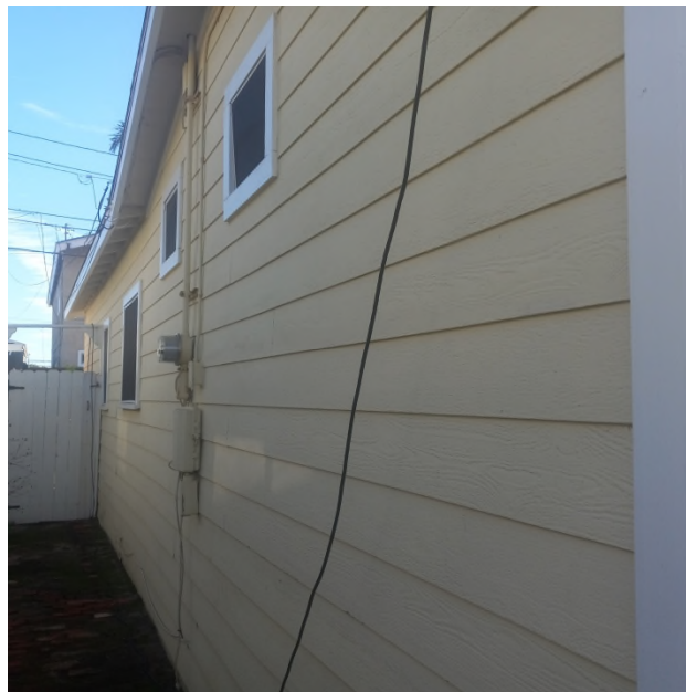
Photograph 3, East Elevation of 136 Los Angeles Avenue, Looking south, December 28, 2023
