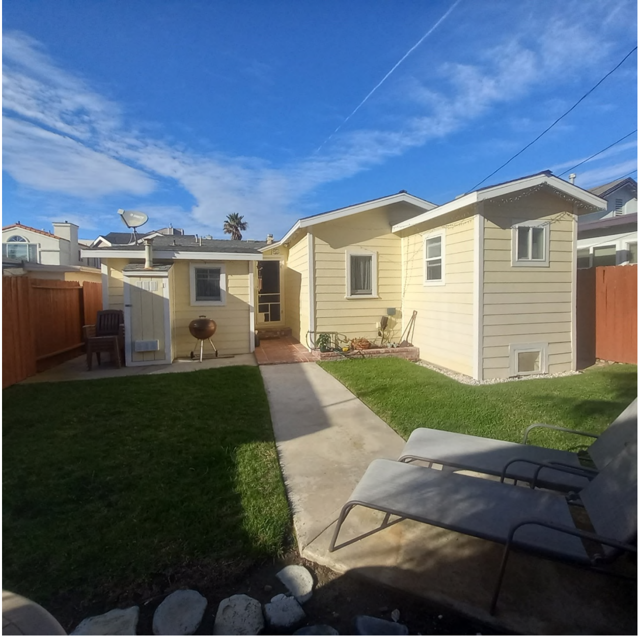
Photograph 14, Looking towards the south elevation of 136 Los Angeles Avenue (December 28, 2023)
