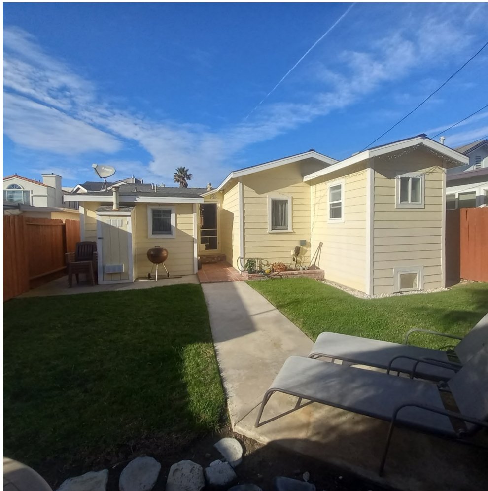
Photograph 2, South Elevation of 136 Los Angeles Avenue, Looking northwest December 28, 2023
