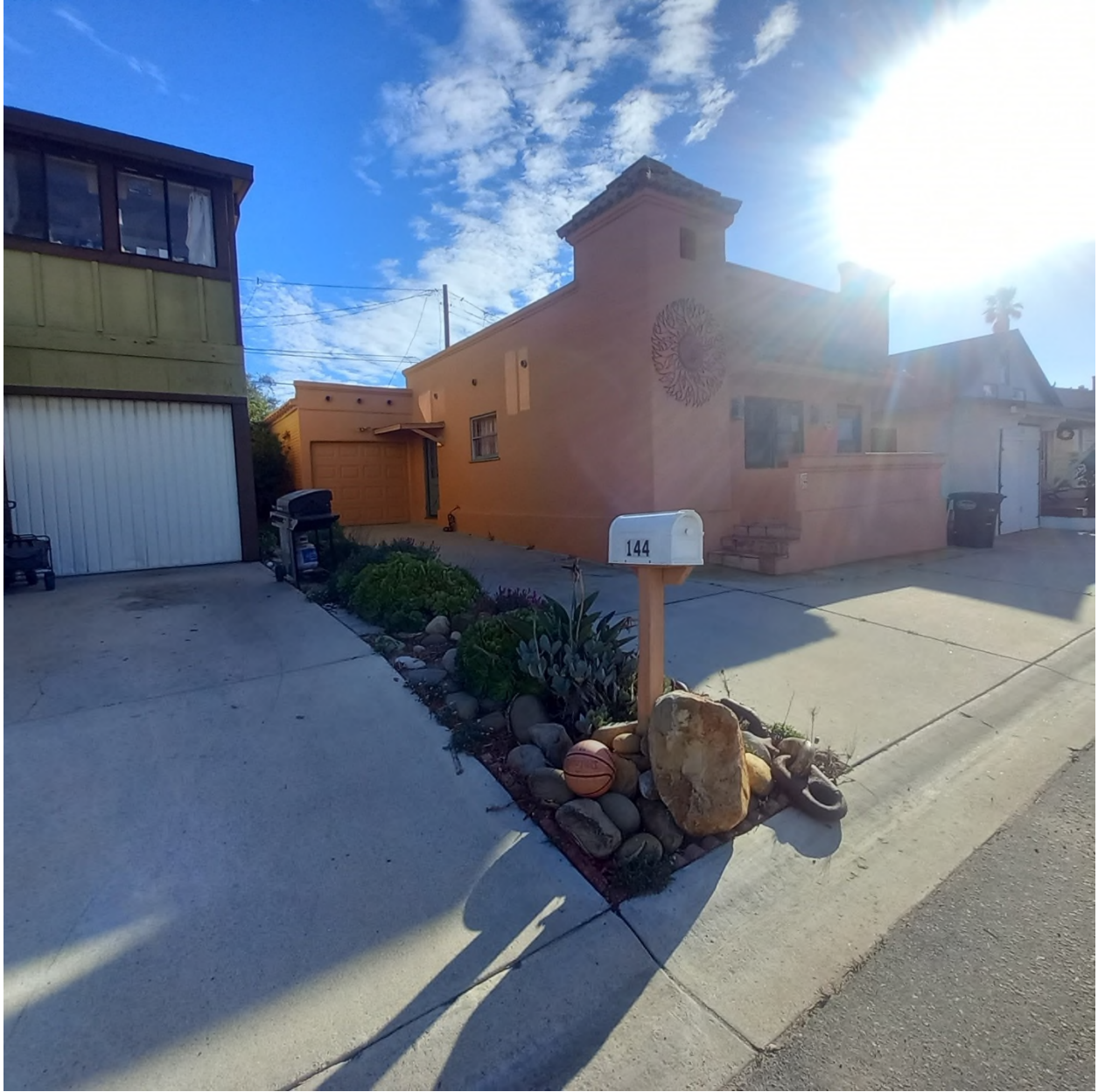
Photograph 9, Looking southwest towards 144 Los Angeles Avenue (December 28, 2023)
