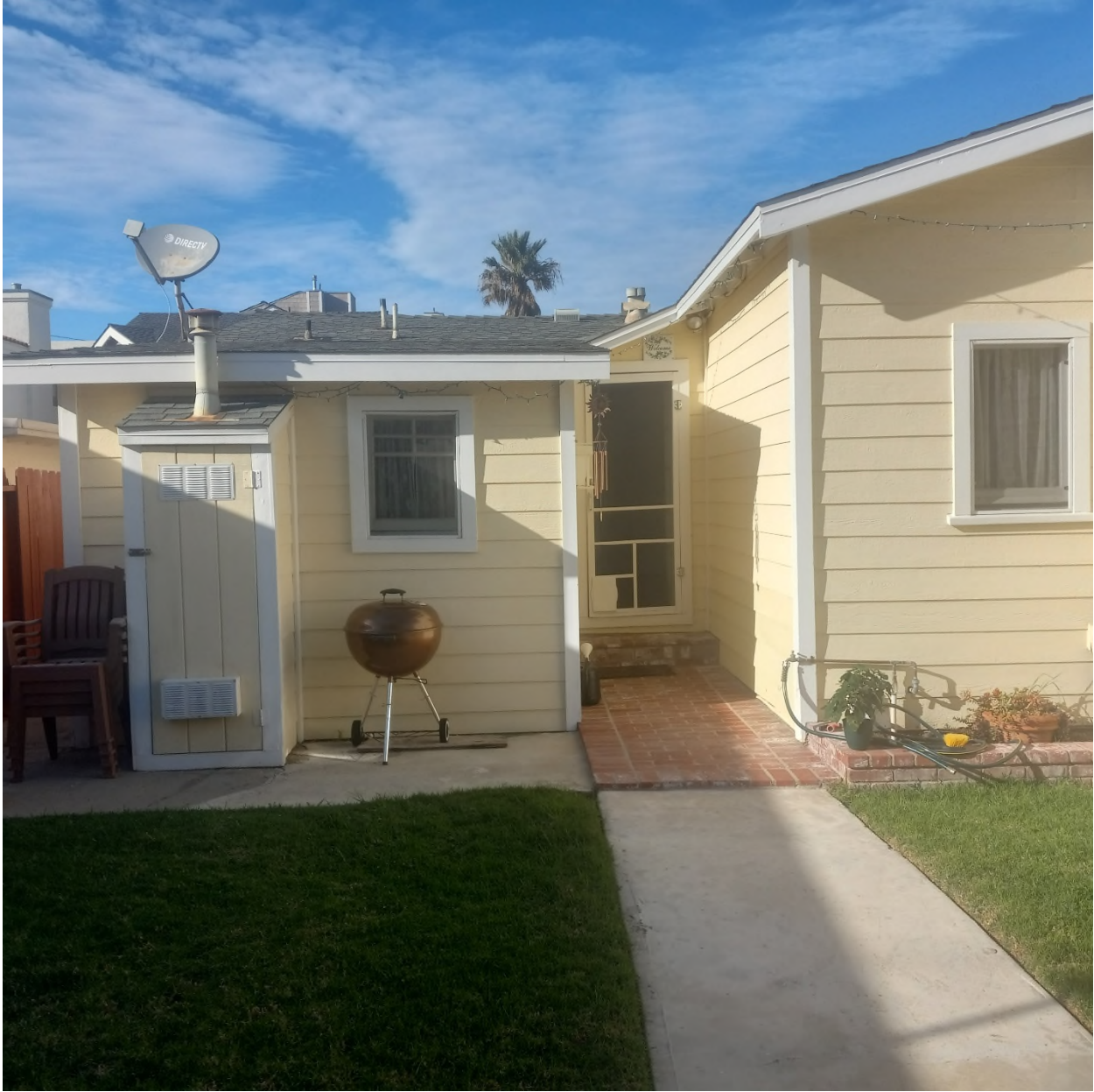
Photograph 15, Looking towards the south elevation of 136 Los Angeles Avenue (December 28, 2023)
