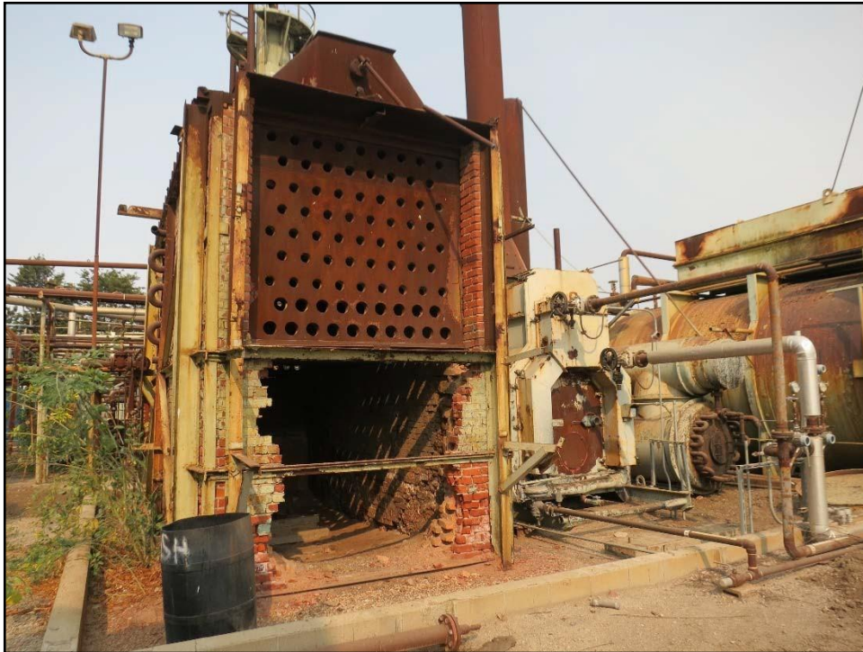
Figure 43. Brick heater, looking northwest.
