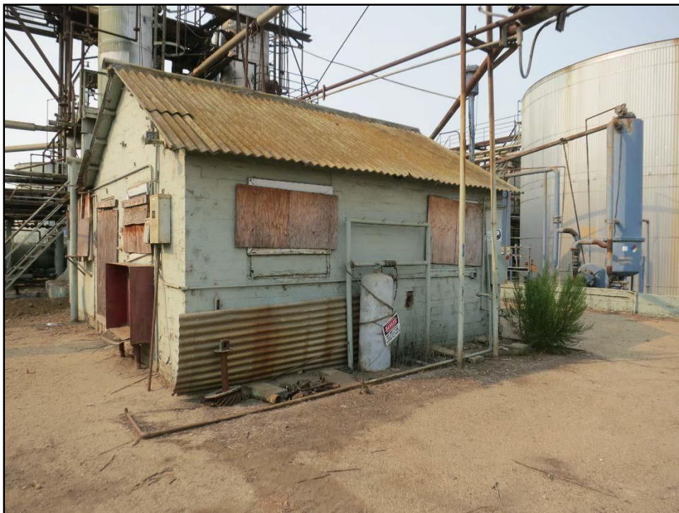
Figure 13. North façade of Control Room, looking southwest.
