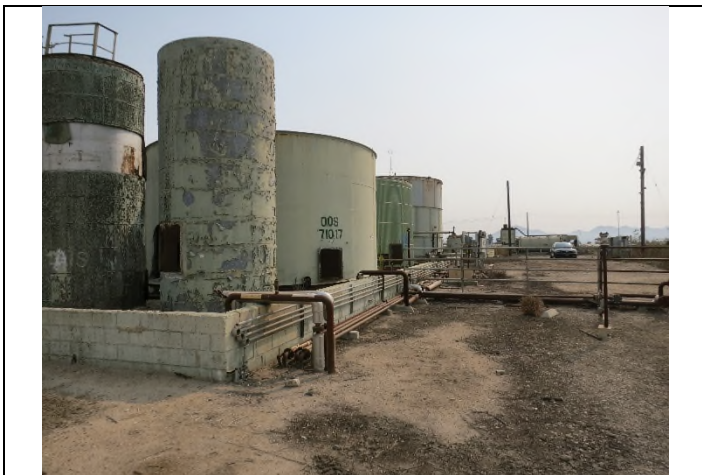
Image 5. View of tanks looking east.
