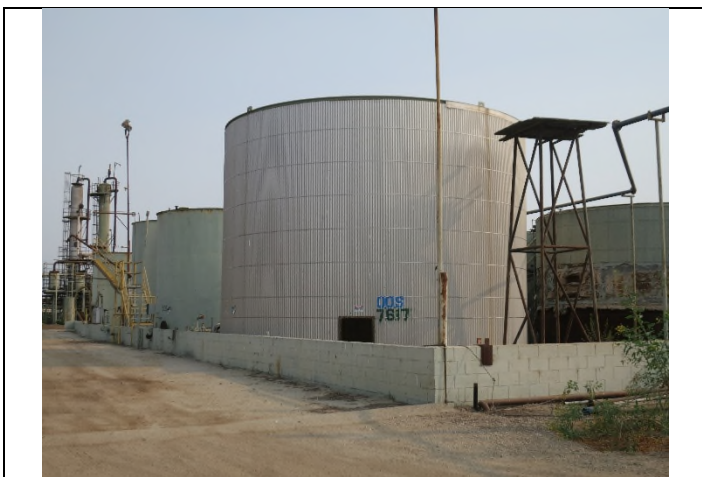
Image 5. View of Tank 3502 looking northeast.
