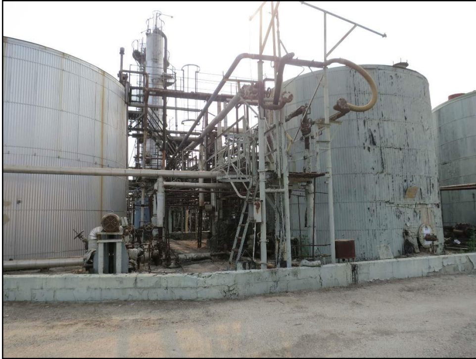
Figure 27. View showing tank 3501 to the left and Tank 1002 to the right, looking east.
