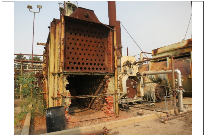
Image 4. Brick heater looking northwest
