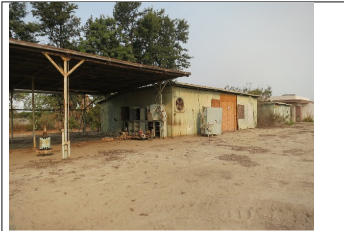
Image 3. View of Maintenance Shop and Lab.
