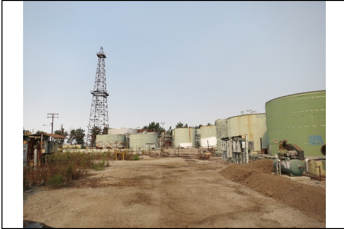
Image 1. Overview of district looking west.
