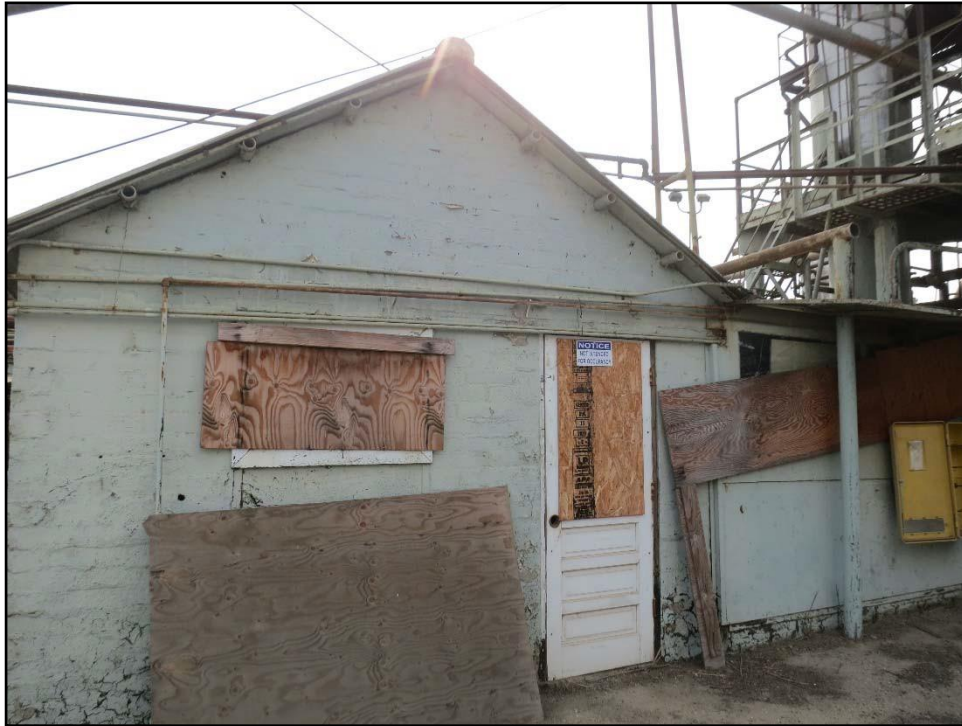
Figure 14. West façade of Control Room, looking southeast.
