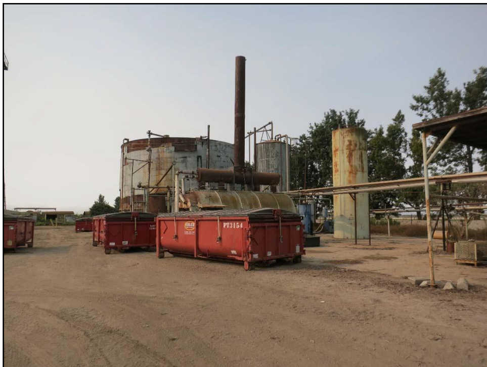
Figure 26. Tanks 506 and 506, looking south.
