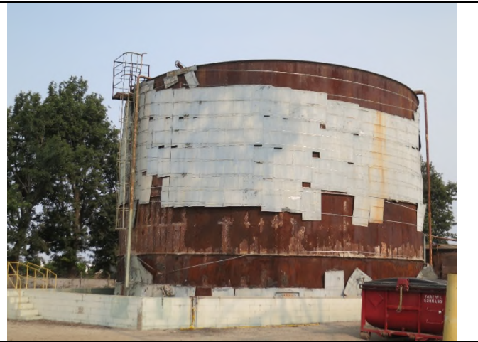
Image 2. Tank 12001 looking west.
