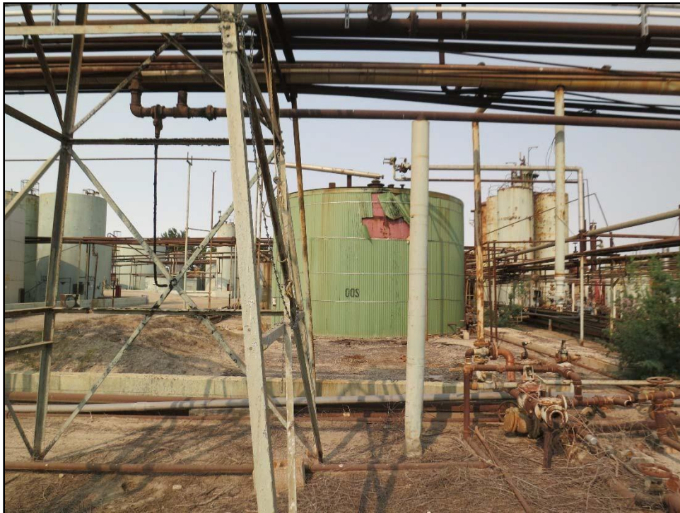
Figure 30. Tank 2003 with empty space where Tank 2004 was located, looking west.
