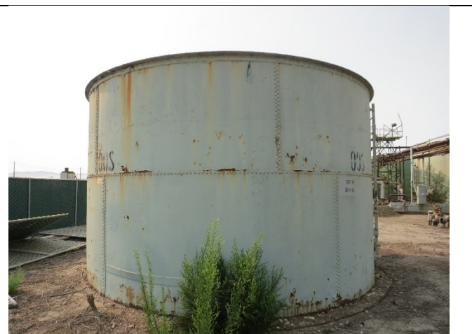
Image 6. Tank 501 looking south.
