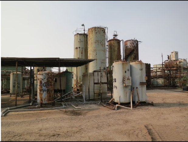
Image 1. Smaller tanks near the center of the parcel looking south.
