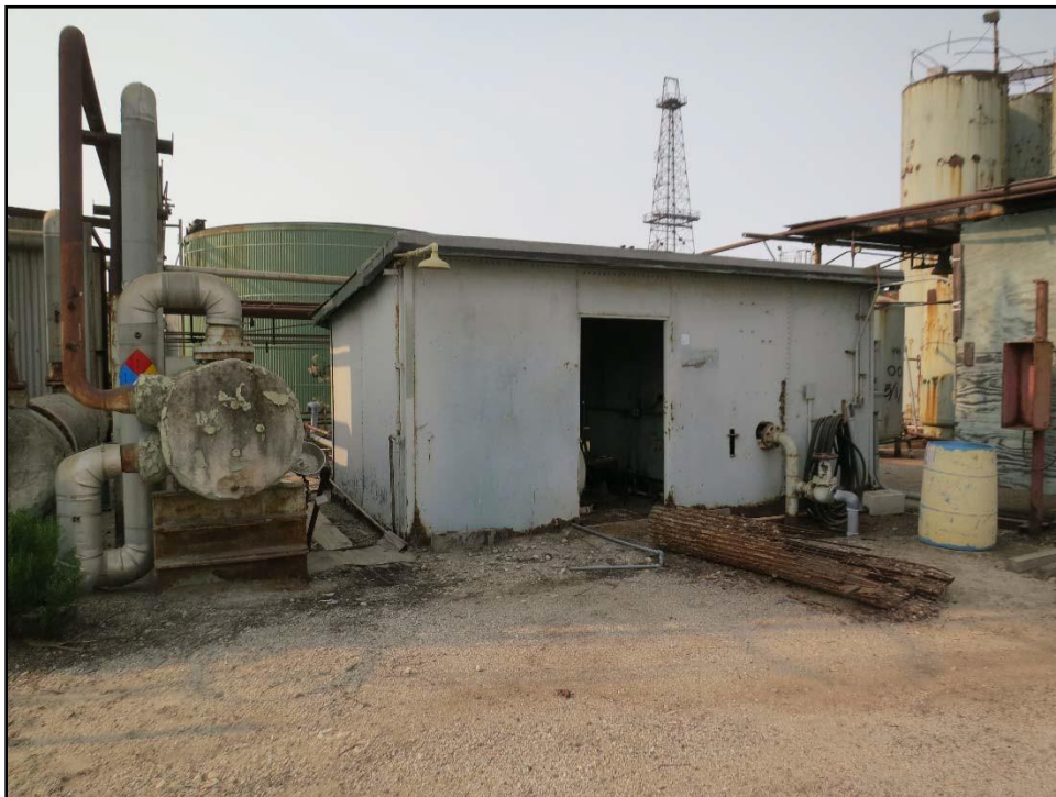
Figure 23. View of north façade of Shed, looking south.
