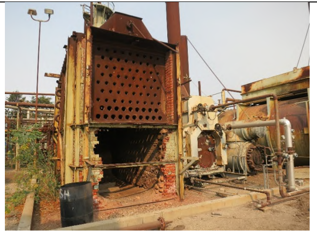
Image 4. Brick heater looking northwest
