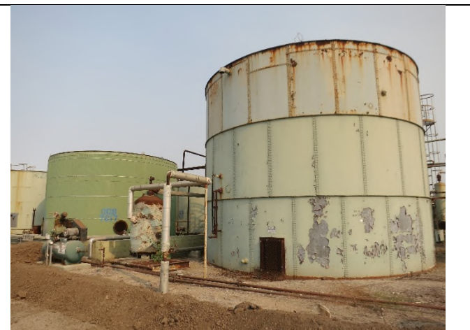
Image 4. View of Water Tank looking northwest
