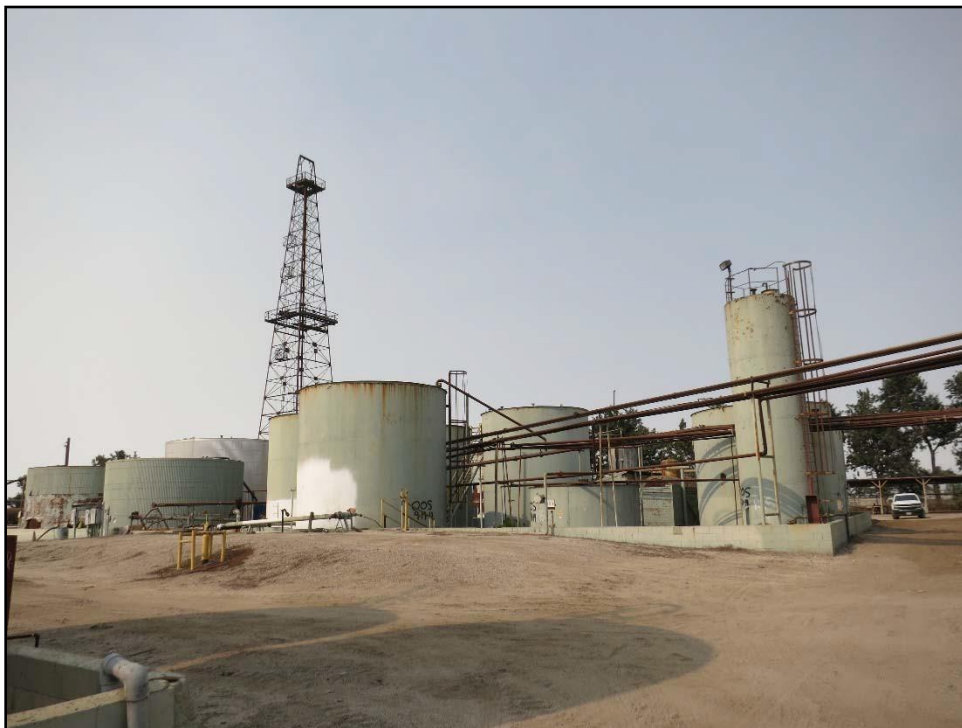
Figure 28. Distant view showing 1500 series tanks in the foreground.
