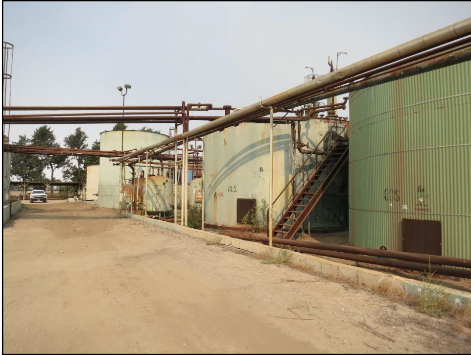
Figure 29. Tank 2002 on right and 2001 to its left, looking west.
