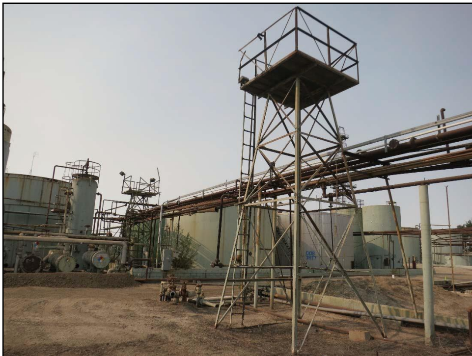
Figure 42. Access platform and pipelines, looking southwest.
