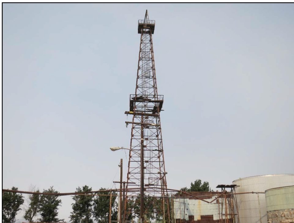
Figure 24. View of Derrick, looking west.
