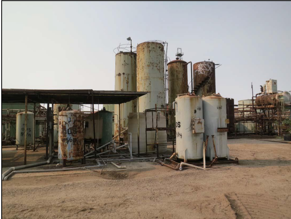
Figure 39. Smaller tanks near the center of the parcel, looking south.
