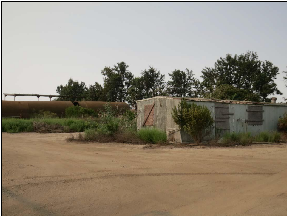
Figure 50. Portable unit and scrap metal on south end of parcel.
