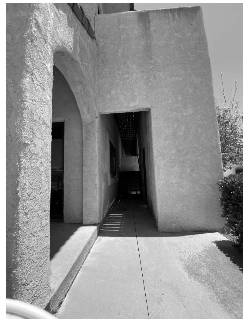
EXISTING STAIR TO REMAIN
