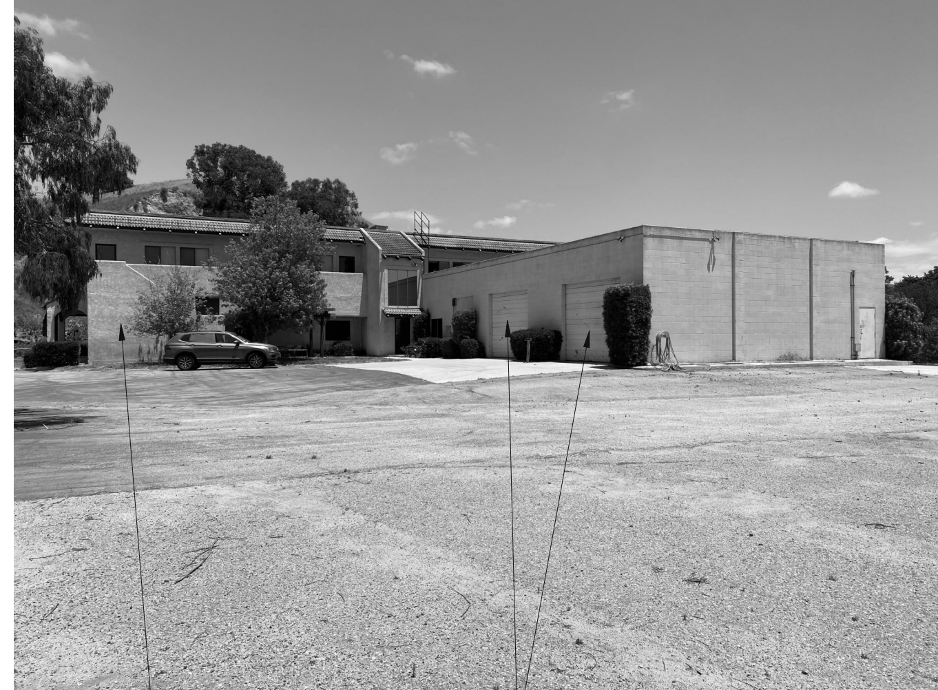
EXISTING STAIR TO REMAIN
