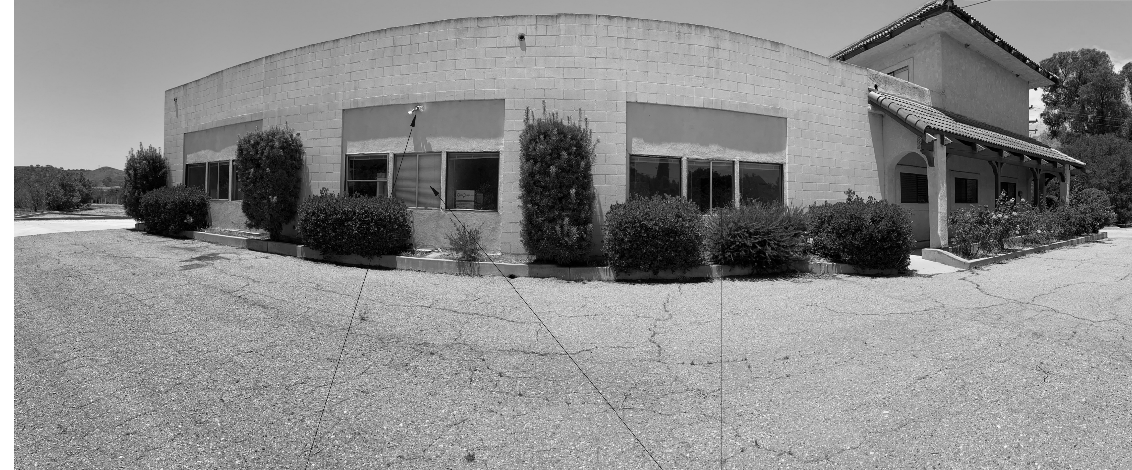
EXISTING LIGHTING TO REMAIN.
