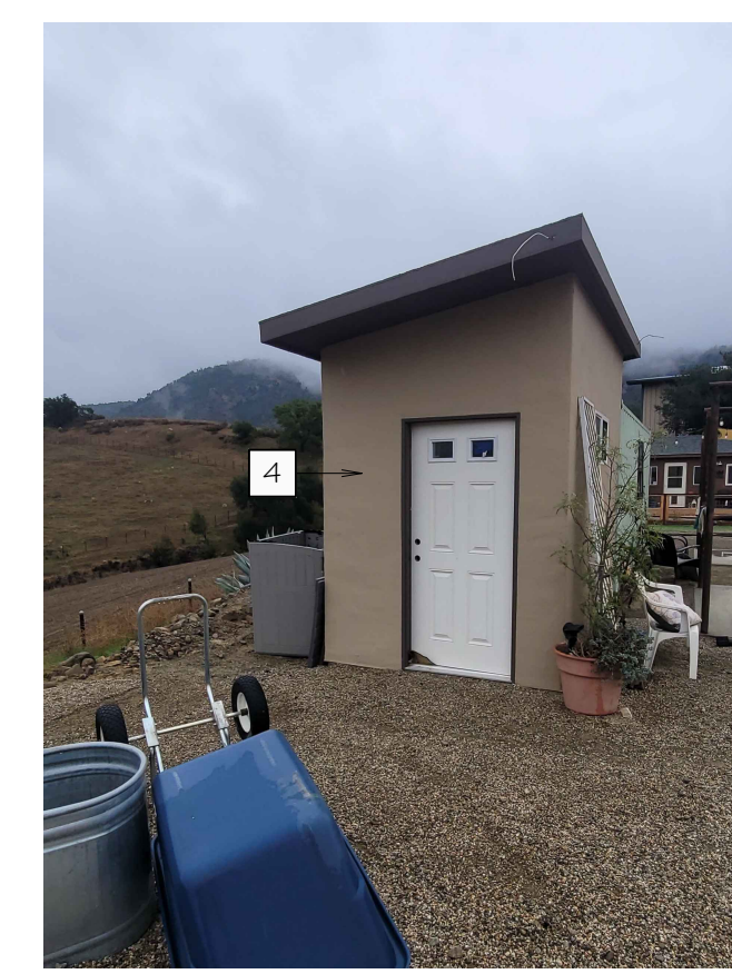
SHED No. 1 NORTH ELEVATION (SHIPPING CONTAINER BEYOND)
