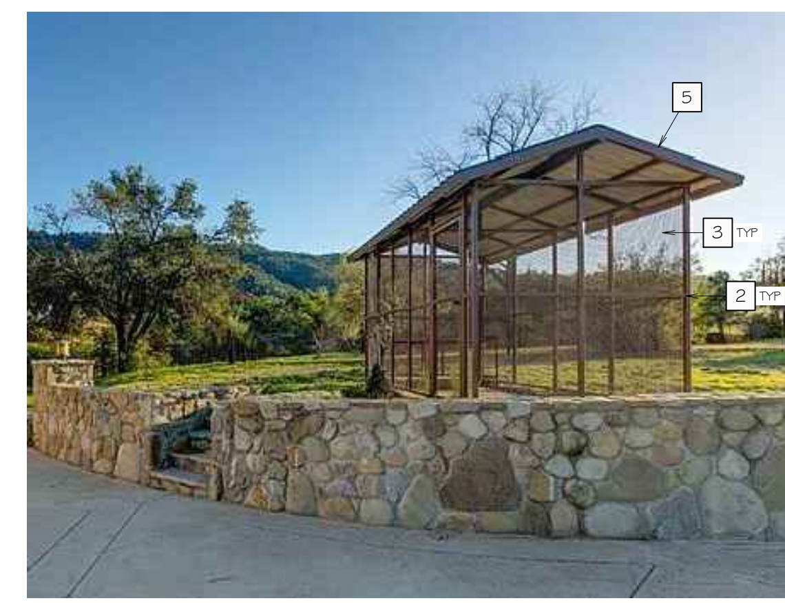
SHED No. 3 NORTH ELEVATION
