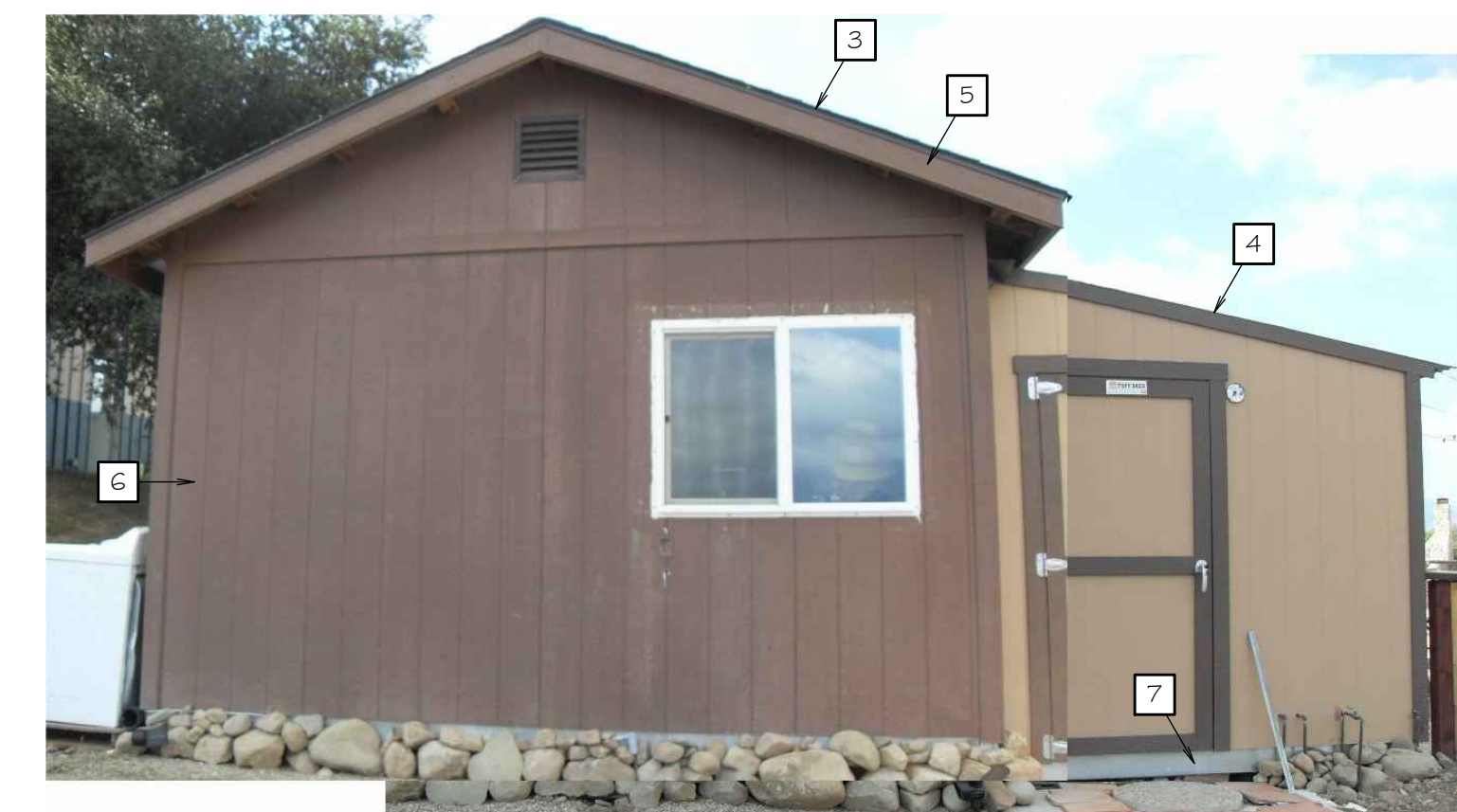
6 EAST ELEVATION AS-BUILT
