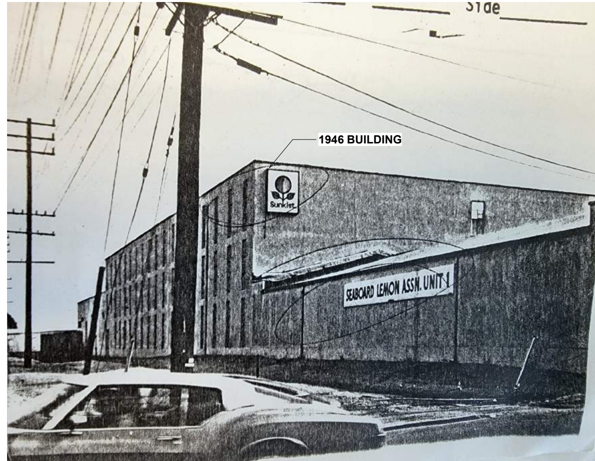
PERSPECTIVE FROM COLONIA ROAD, VIEW TOWARDS NORTH EAST, 1970s
