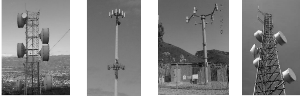
Examples of Non-Stealth Wireless Communication Facilities
