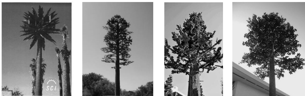
Examples of Faux Trees (Wireless Communication Facilities)
