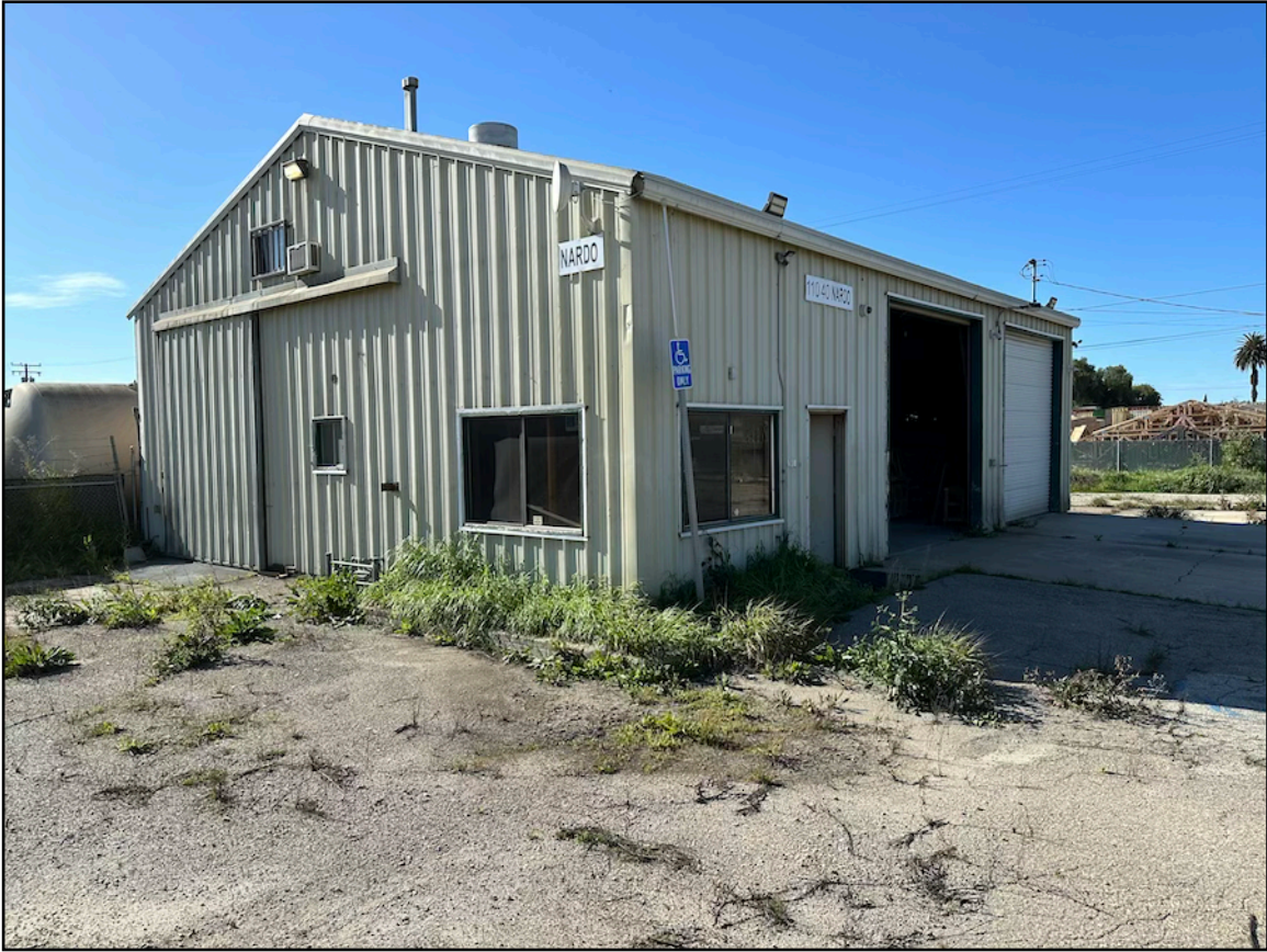
Photo 1. Shop Building, northwestern and northeastern elevations, viewed from north. [3-15-2024]
