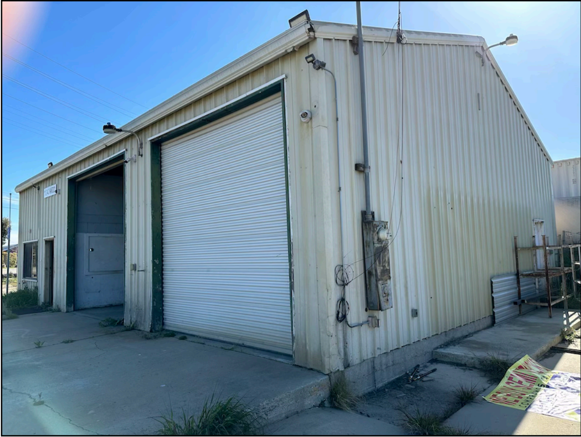
Photo 2. Shop building, northeastern and southwestern elevations, viewed from west. [3-15-2024]
