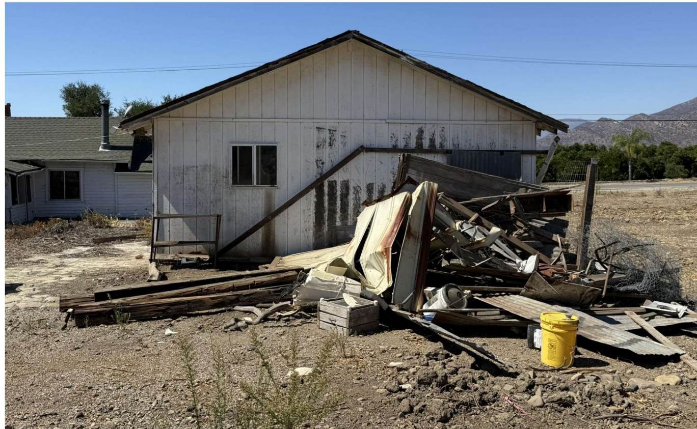
EXISTING GARAGE - EAST ELEVATION
