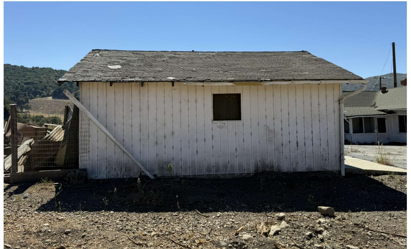
EXISTING GARAGE - NORTH ELEVATION
