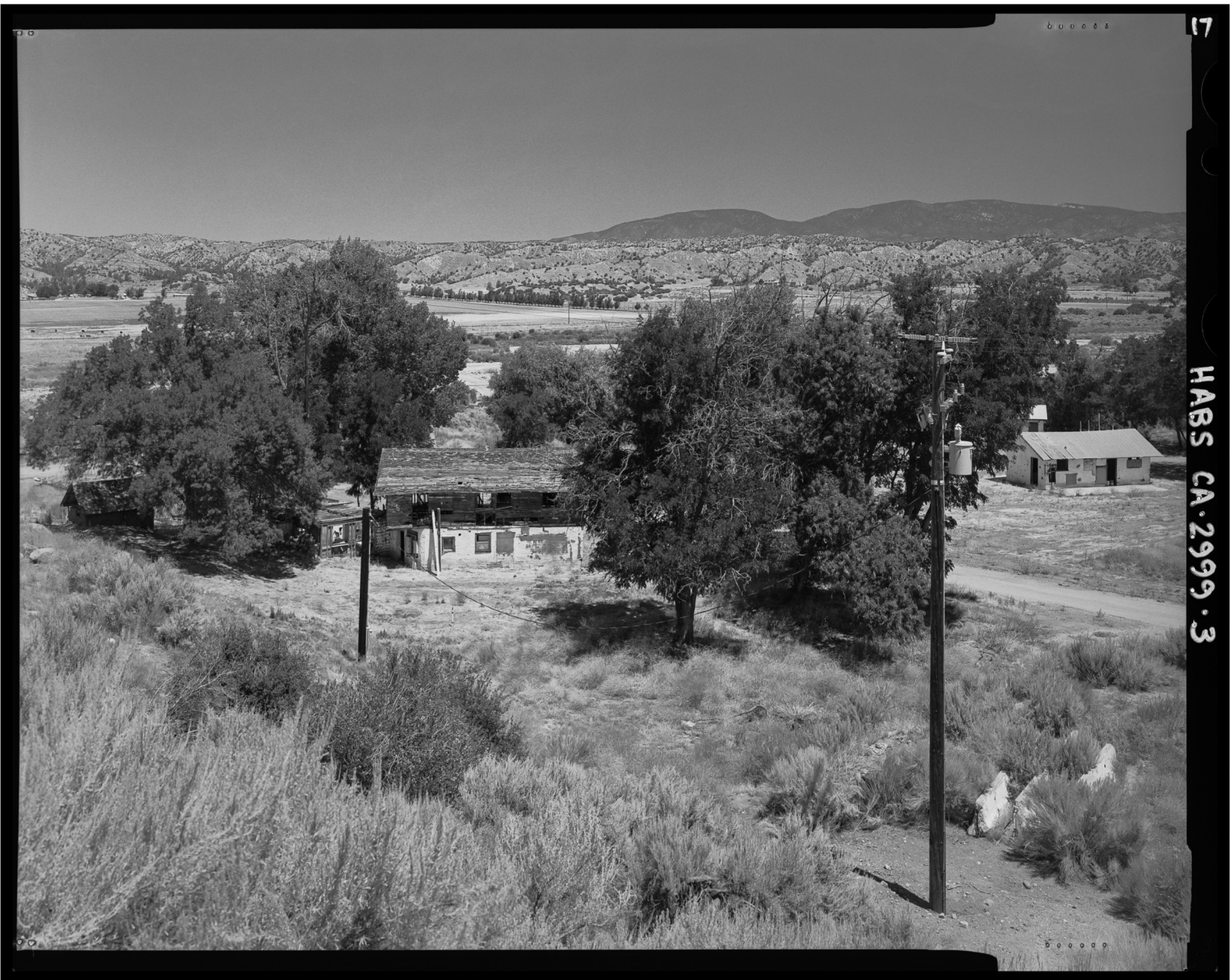
HISTORIC AMERICAN BUILDINGS SURVEY SEE INDEX TO PHOTOGRAPHS FOR CAPTION HABS No. CA - 2999 - 3
