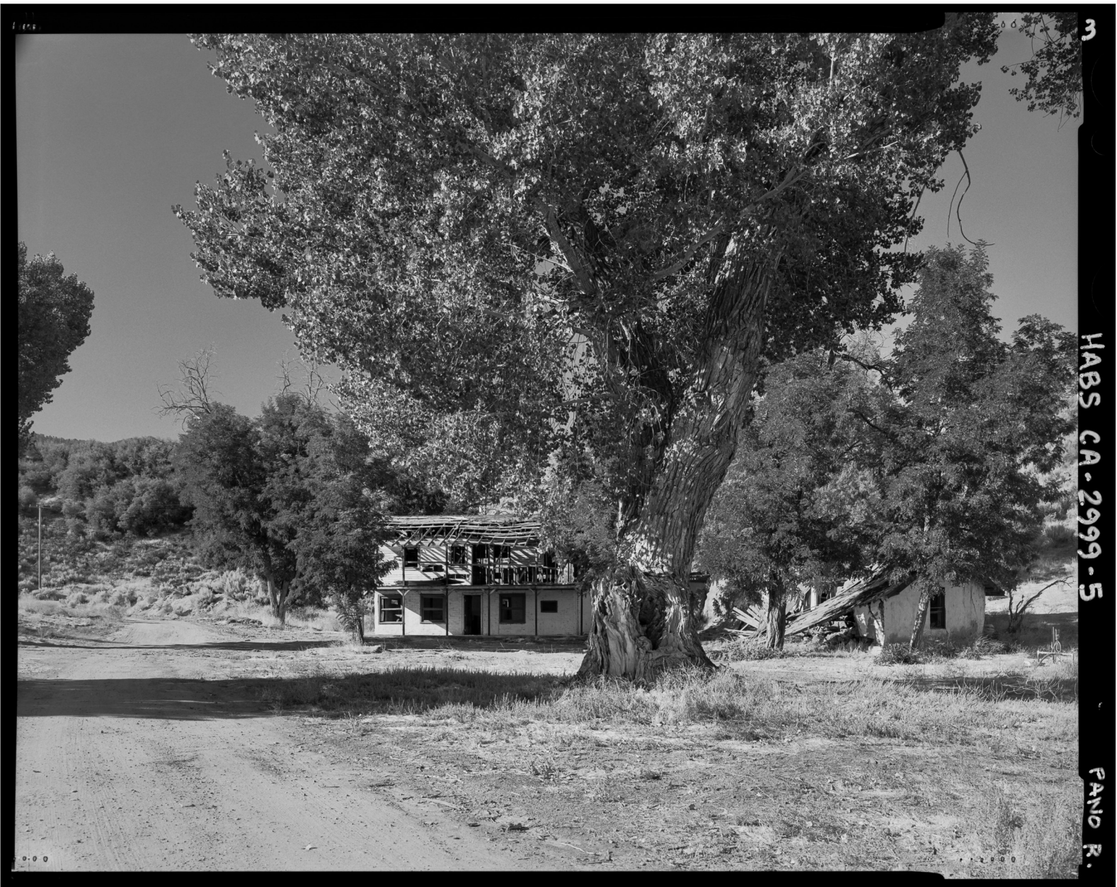
HISTORIC AMERICAN BUILDINGS SURVEY SEE INDEX TO PHOTOGRAPHS FOR CAPTION HABS No. CA - 2999 - 5
