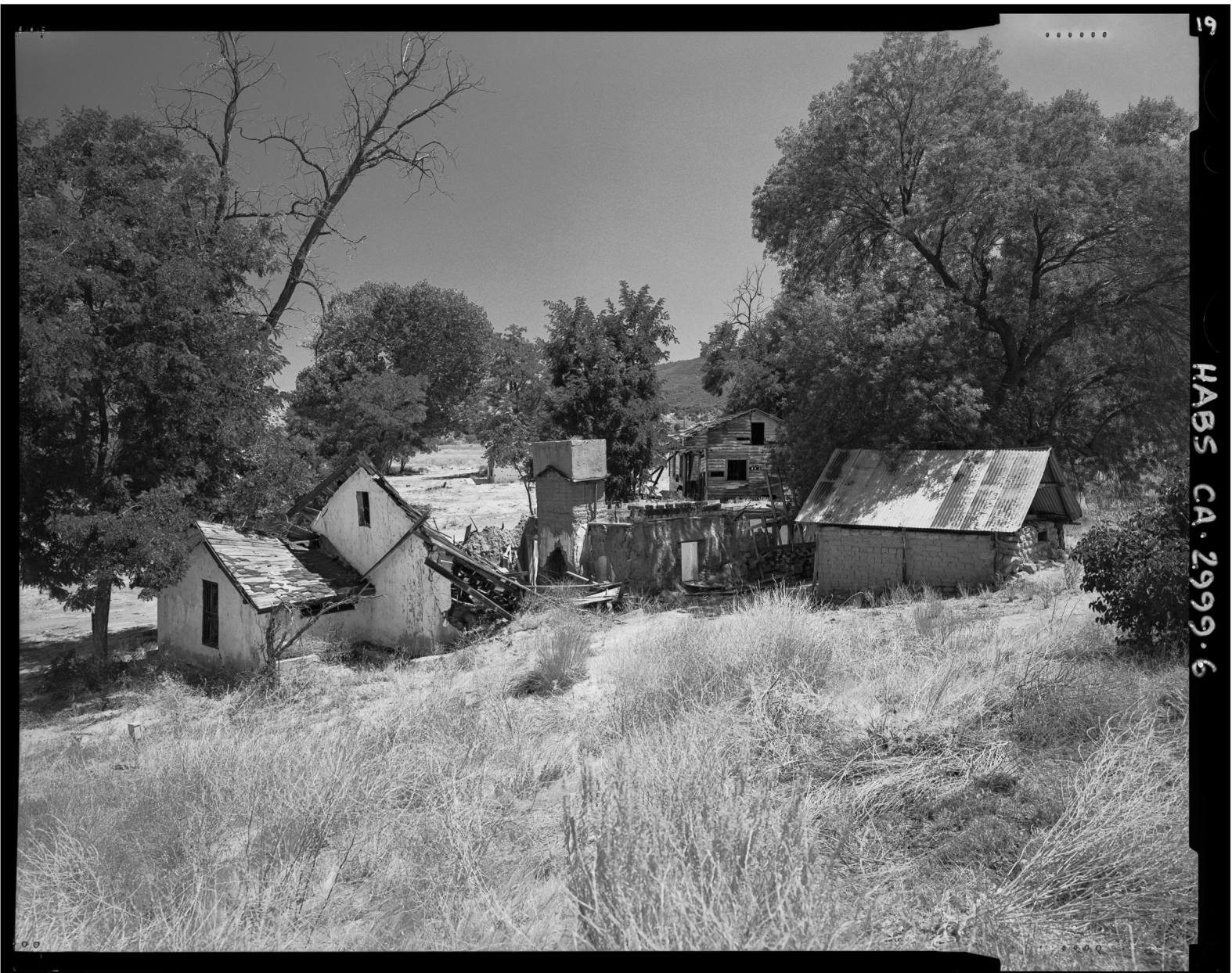
HISTORIC AMERICAN BUILDINGS SURVEY SEE INDEX TO PHOTOGRAPHS FOR CAPTION HABS No. CA - 2999 - 6
