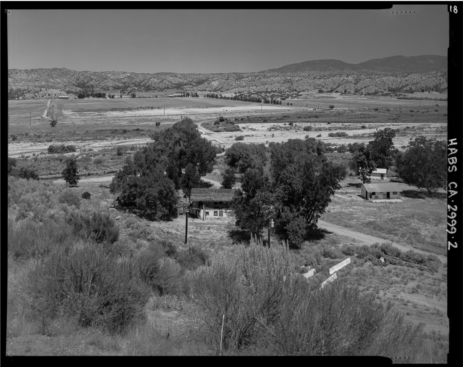
HISTORIC AMERICAN BUILDINGS SURVEY SEE INDEX TO PHOTOGRAPHS FOR CAPTION HABS No. CA - 2999 - 2
