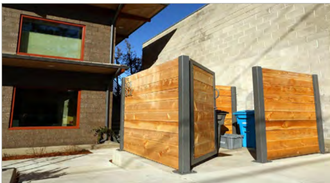
Image 6.19. A screened trash enclosure.
