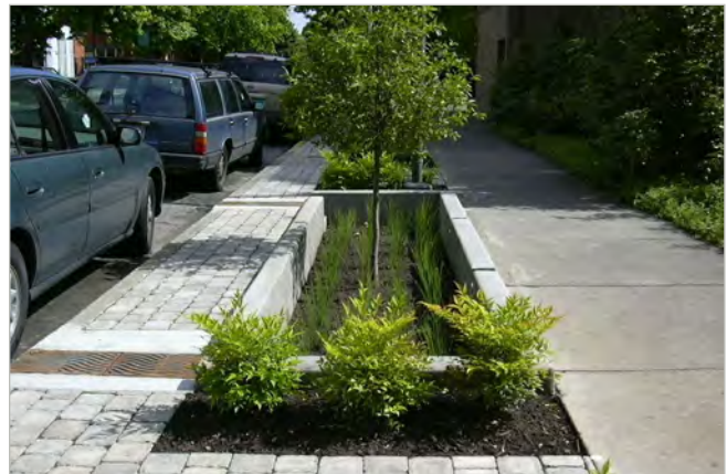
Image 6.30. A curbside rain garden collects and filters stormwater.
