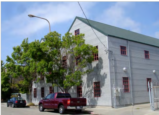
The Light Industrial zone is up to two stories in height, and is occupied by industrial, manufacturing, office and small scale retail uses.
