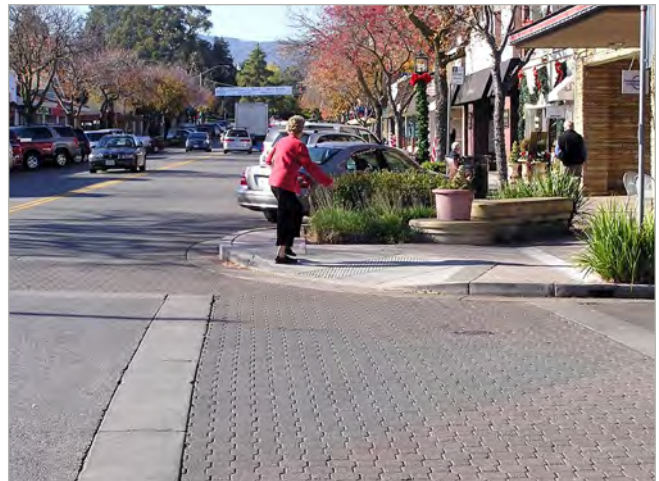
Image 6.35. A crosswalk finished with pavers and cast concrete borders.
