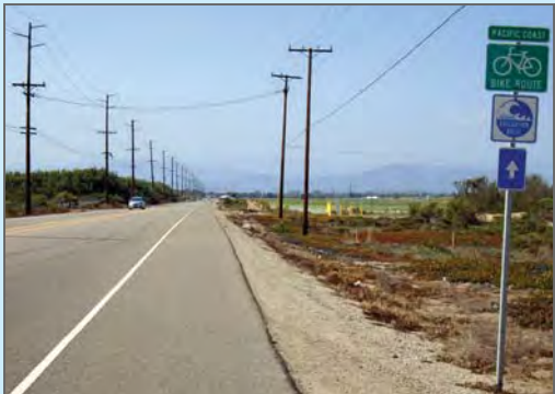
Harbor Boulevard includes a Class 2 Bike Lane
