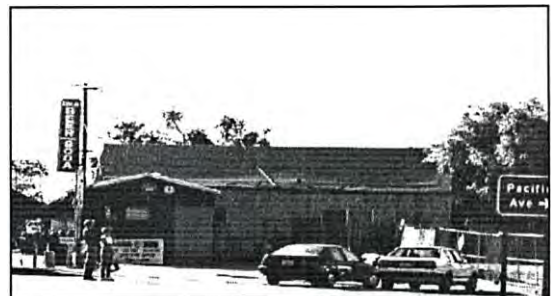
Existing highway commercial – the Plan acknowledges the need for revitalizing Piru’s highway frontage consistent with the image of the town.
