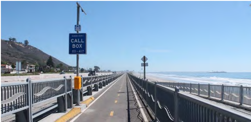
This Multi-Modal Route (N1) includes a path constructed by Caltrans as part of the Ventura to Santa Barbara Highway 101 HOV project.
