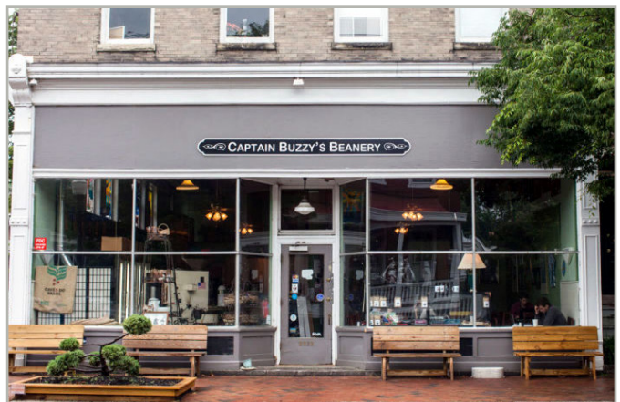
Shopfront Example - large glazing area of display windows, and recessed storefront entry with glass door.
