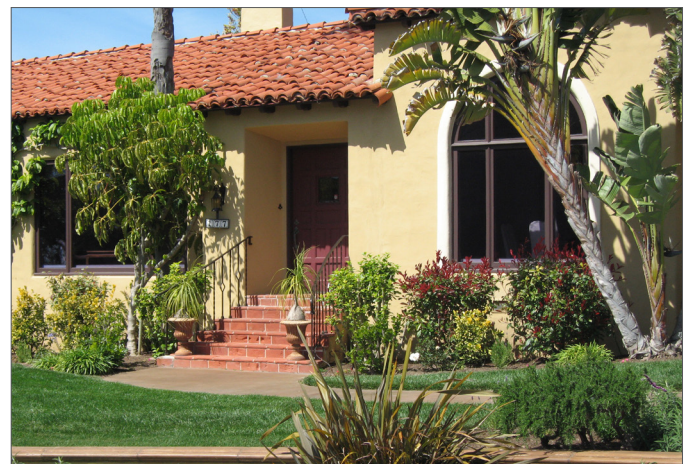
Stoop Example - stairs, landing, and landscape area.
