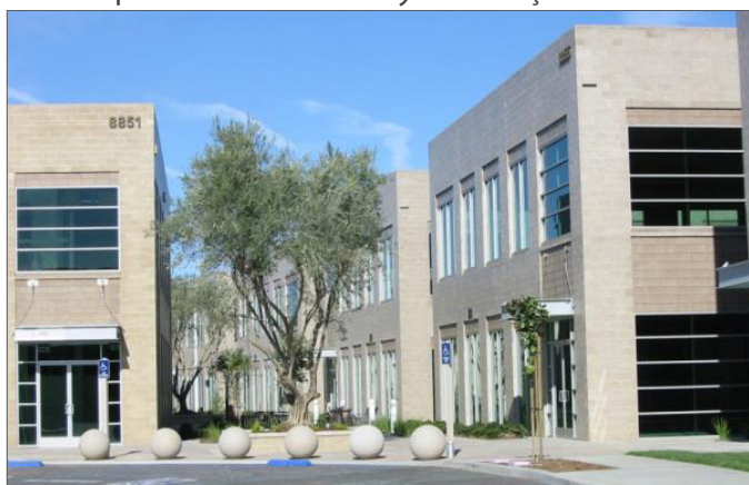
Example of an Industrial Building with a continuous band of street-facing windows.
